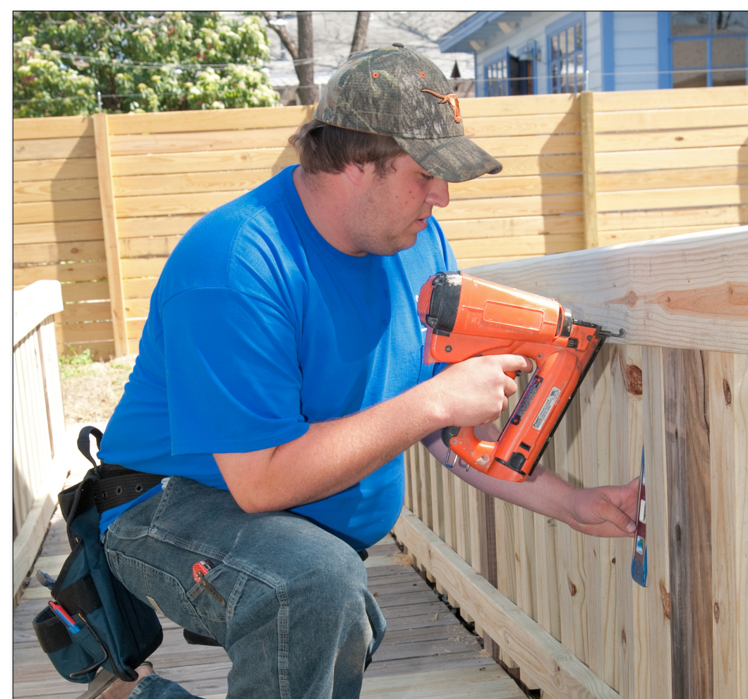
We install ramps for easy home accessibility.
