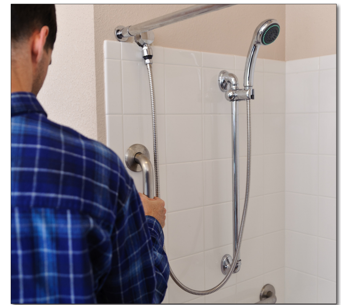
We install grab bars for safety.
