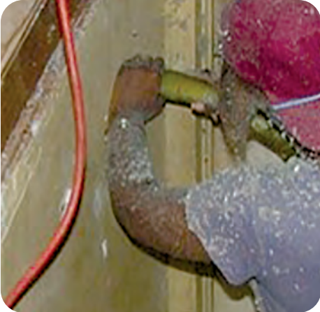
7. Dense pack stairway walls
