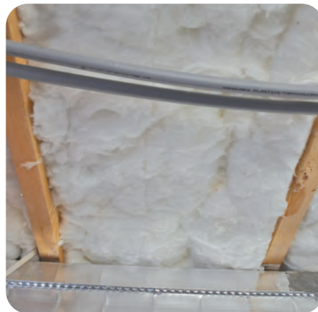
4. Batts installed with no gaps
