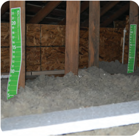
5. Depth rulers installed, 1 per 300 square feet
