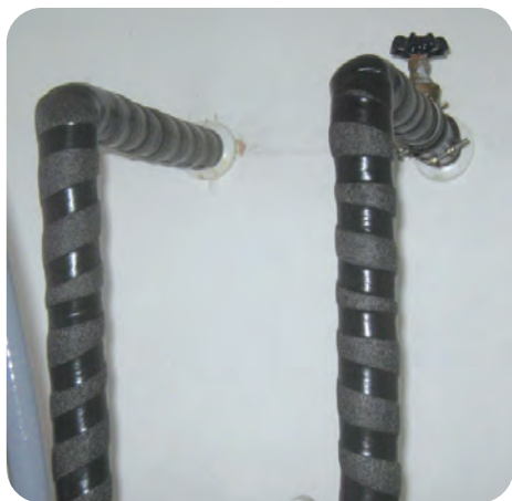
Secure seams with tape
