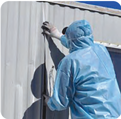
8. Reinstall siding
