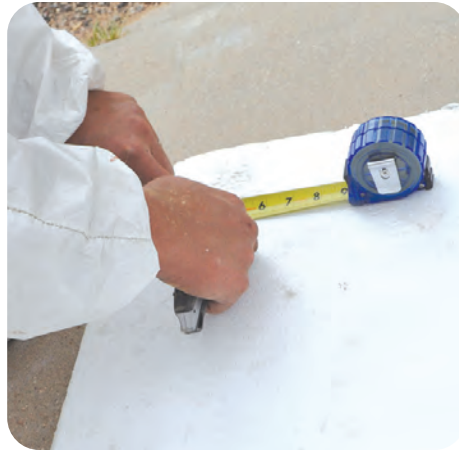
2. Cut blocking material to fit
