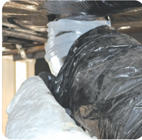
2. Pull insulation over hard connections as needed
