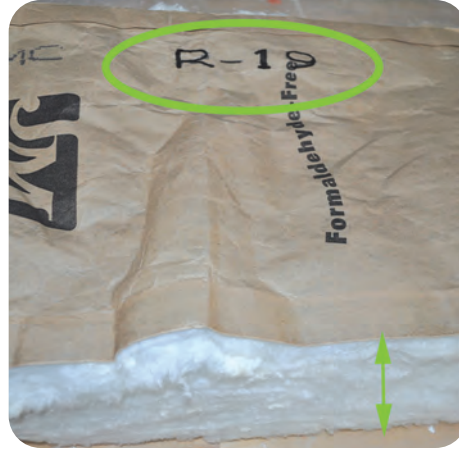
2. Insulation R-value matches work order
