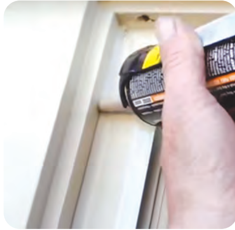
8. Caulk all exterior edges
