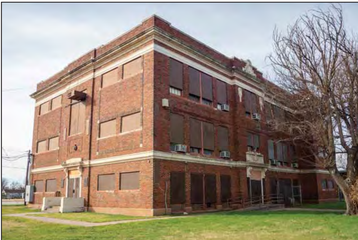
2. Classroom Building, Oblique, North and East Elevations View SW
