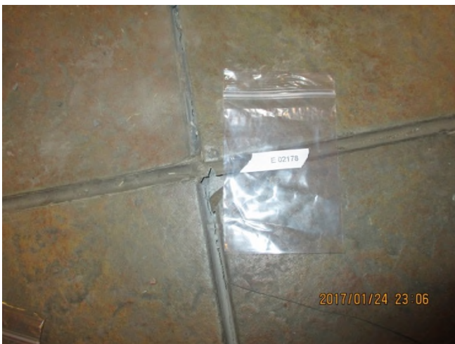
Photo 5: View of expansion joint caulk sample location.
