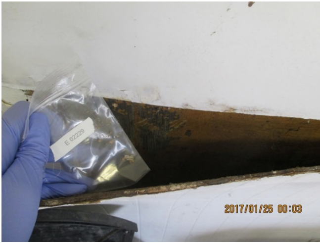
Photo 19: View of the FRP mastic sample location.
