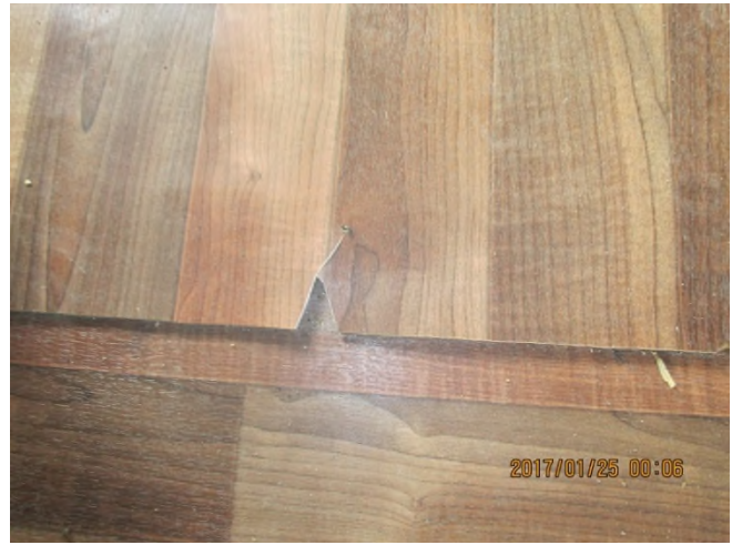
Photo 20: View of the linoleum sheet flooring sample location.
