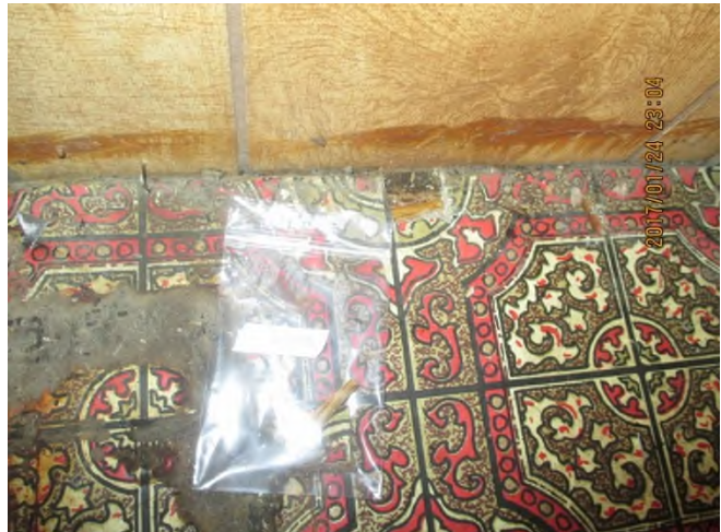
Photo 4: View of red linoleum sheet flooring and mastic (multiple layers) sample location (30% Chrysotile).
