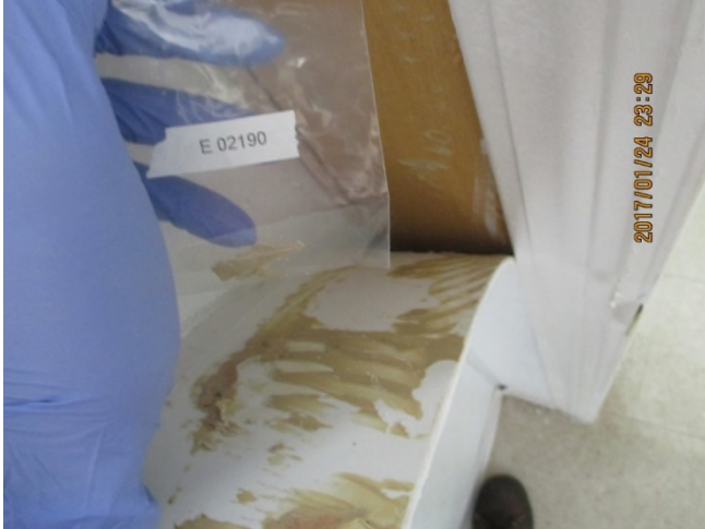
Photo 9: View of the FRP mastic sample location.
