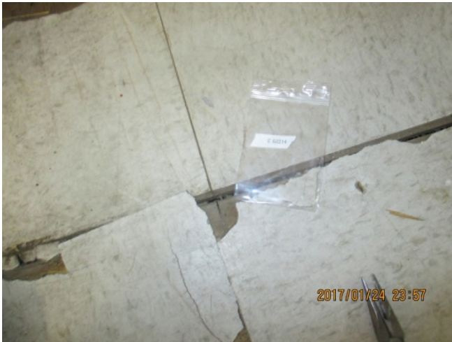
Photo 15: View of the white VFT and associated mastic sample location.
