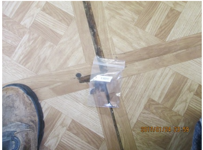
Photo 16: View of wood look linoleum flooring sample location.
