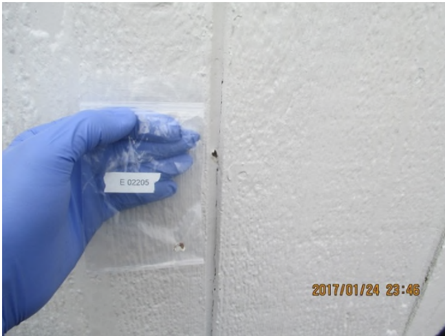
Photo 13: View of the exterior caulking sample location.
