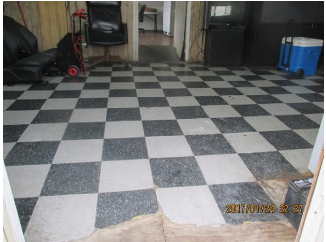
Photo 14: View of the black and gray VFT and associated mastic sample locations.
