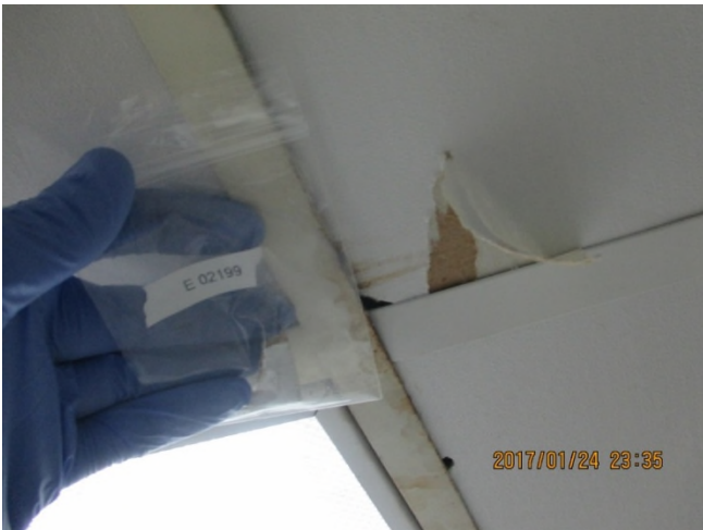
Photo 11: View of gypsum ceiling tile sample location.
