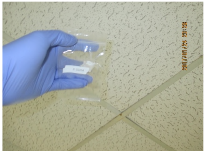
Photo 12: View of 2'x4' acoustic ceiling tile sample location.
