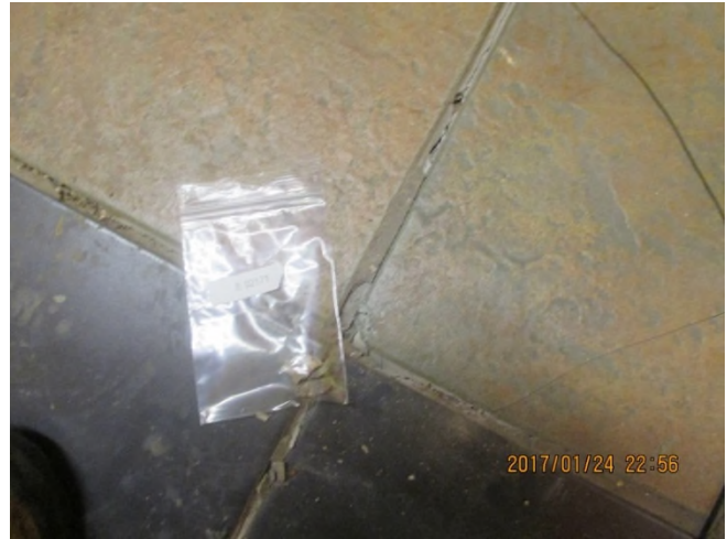
Photo 2: View of the brown ceramic tile, grout, thin-set, and fiber backing sample location (50% Chrysotile).
