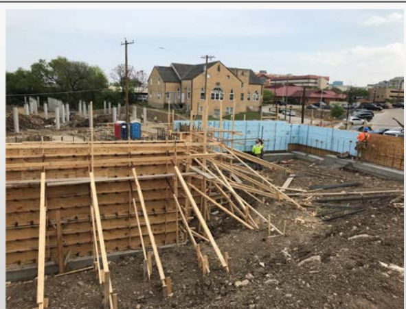
Foundation for Building B
