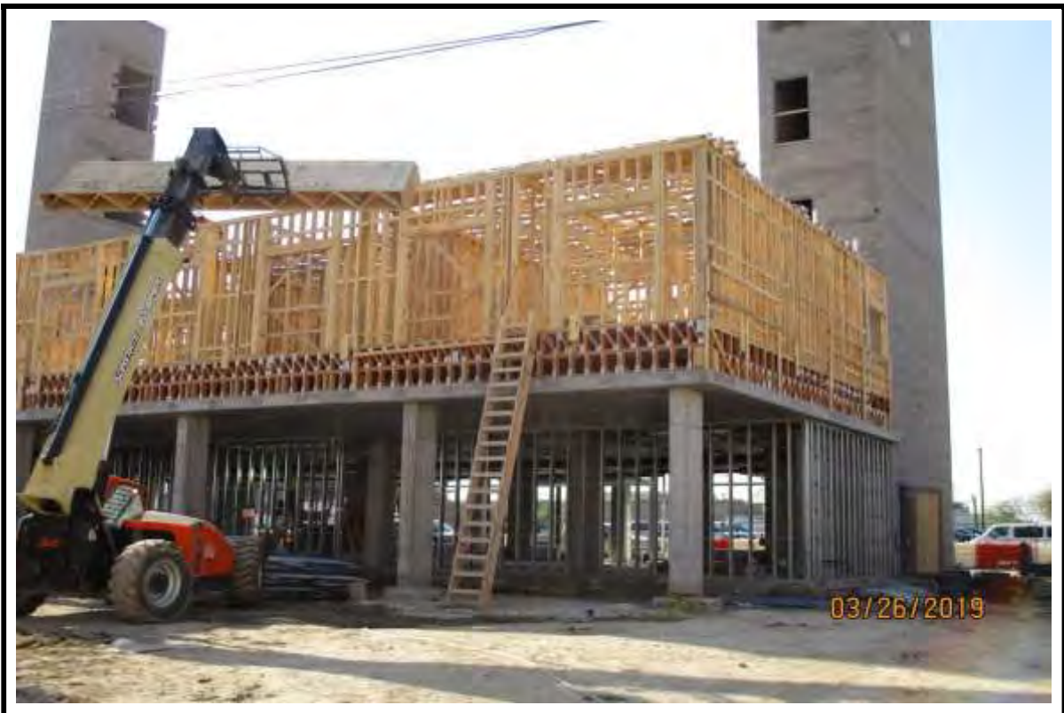
Photograph 8: Lifting trusses at Building "A".
