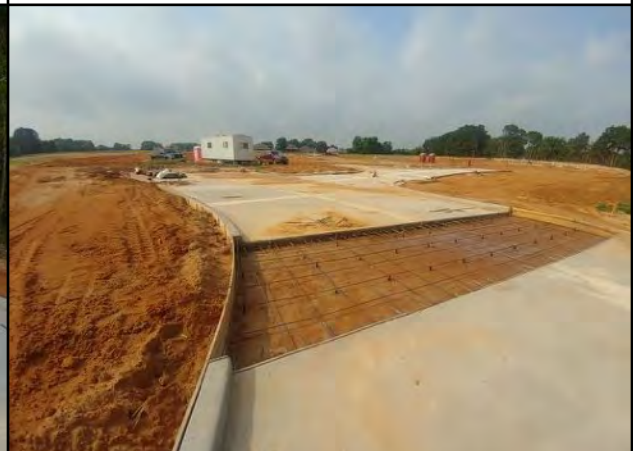
Photo # 6 Pouring of concrete paving in progress at Sunset Drive
