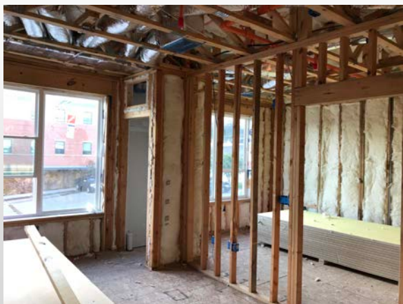
Insulation Installation at Building B
