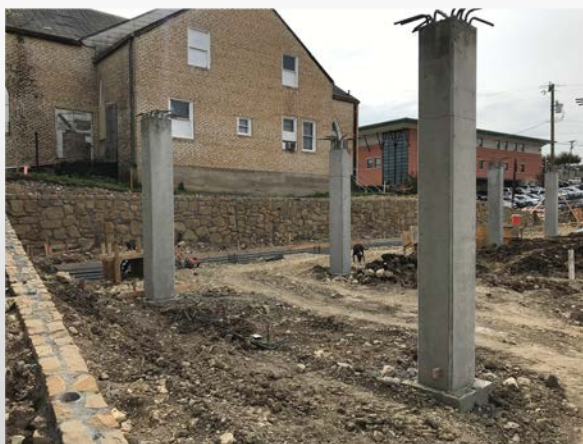
Podium columns and retaining wall at Building B
