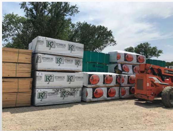
Stored Framing Material
