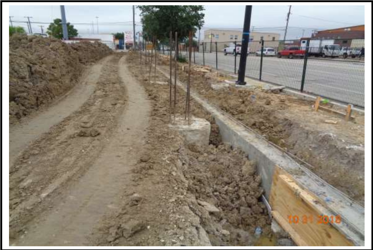
Photograph 8: Backfilled South grade beam at Building "A".
