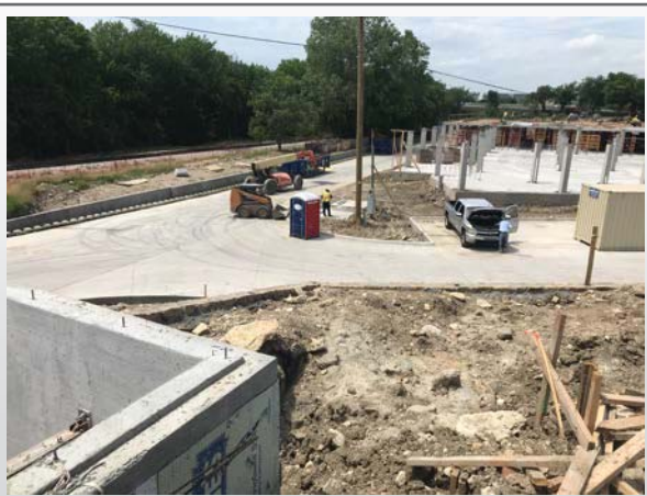
Looking North Across site toward Building A
