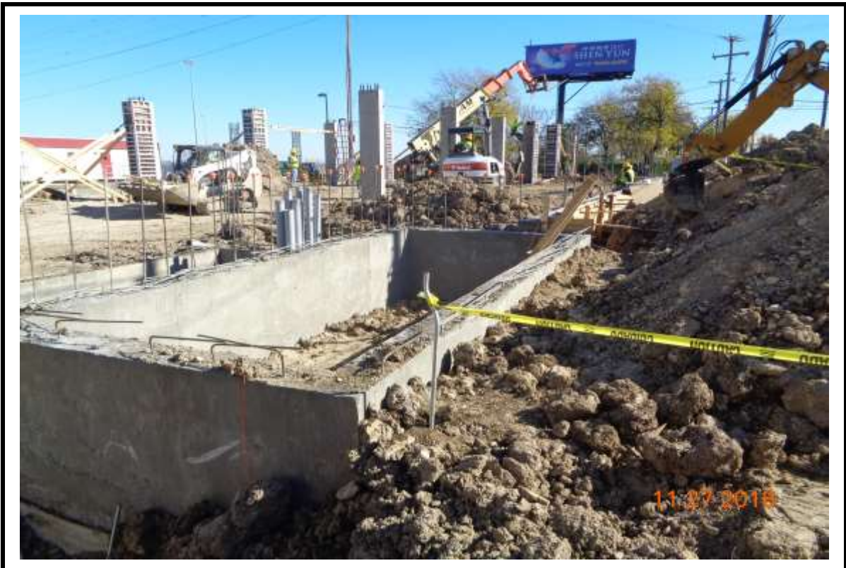
Photograph 6: Stairwell beams at Building "B".
