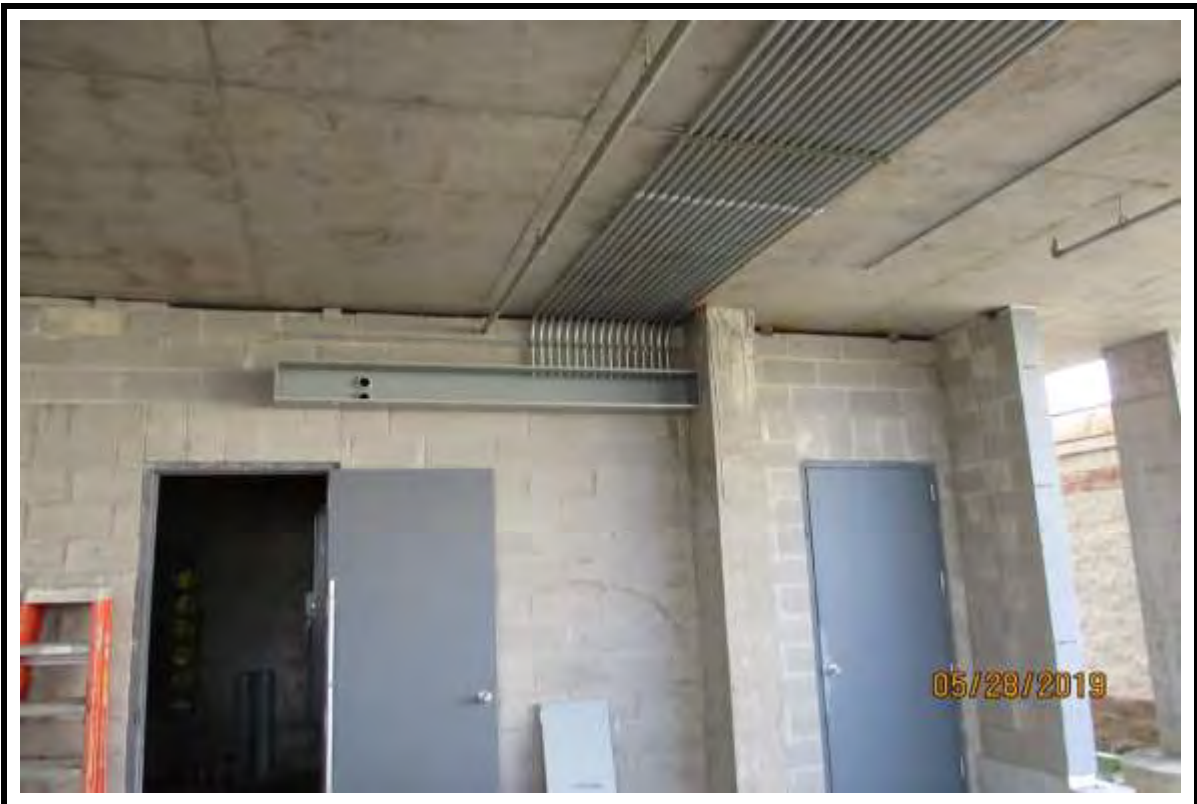
Photograph 10: Overhead conduit rough-in from electrical main distribution at Building "B".
