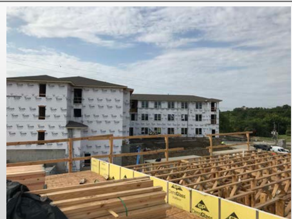
Framing and Firewall at Building A
