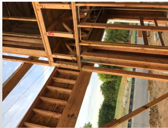
Framing at clubhouse storefront location
