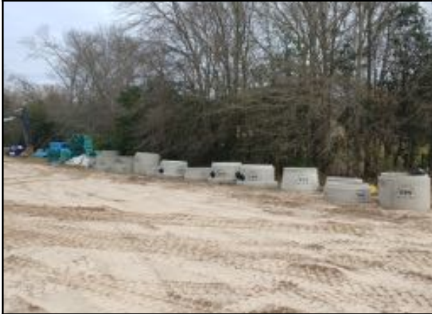
Photo # 3 Staged sanitary, domestic, and sewer
