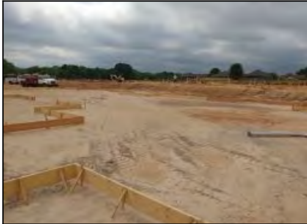
Photo # 13 Building pad 3 overview - form boards set and underground plumbing complete
