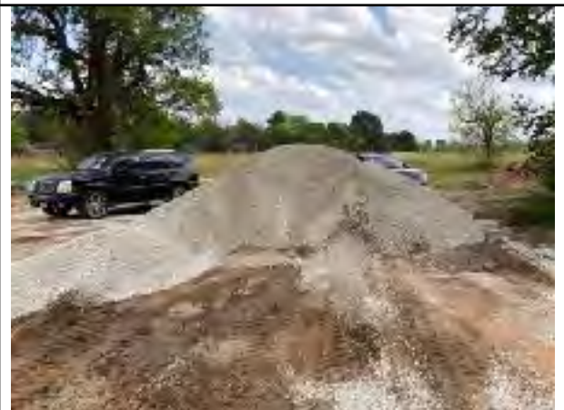
Photo # 24 Backfill gravel stored on site
