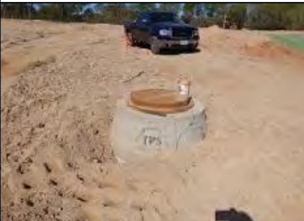
Photo # 6 Detail of sanitary sewer manhole
