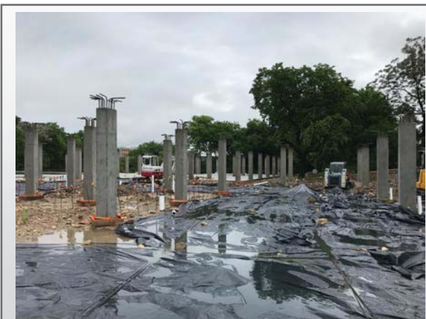
Building A parking and columns
