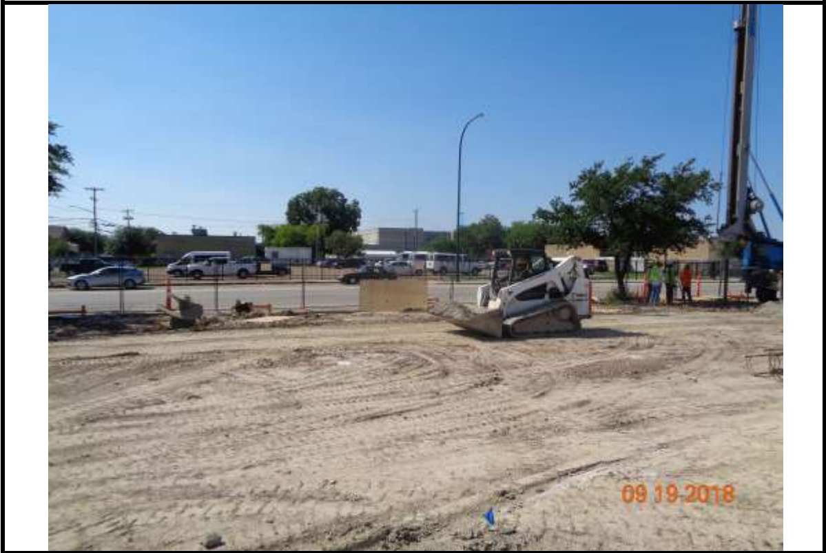
Photograph 9: Removing pier soil spoils to haul-off area.
