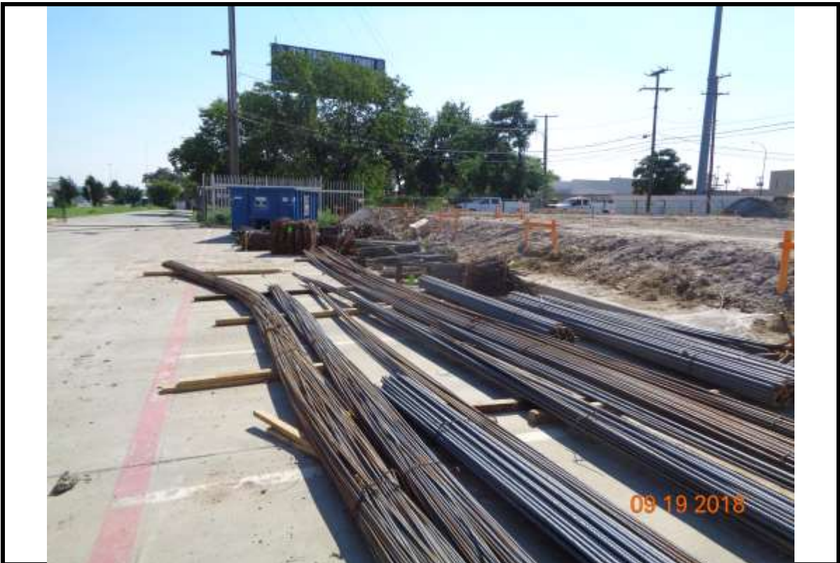
Photograph 2: Reinforcing for drilled piers.
