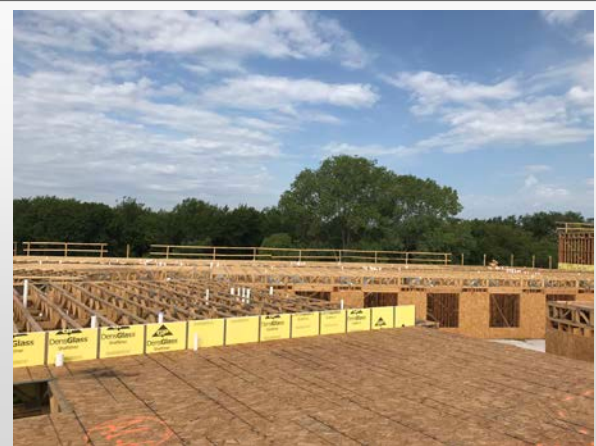
Framing and Firewall at Building A
