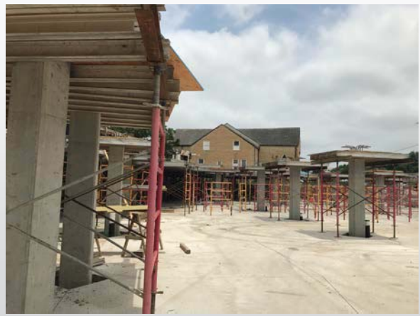
Formwork for Building A
