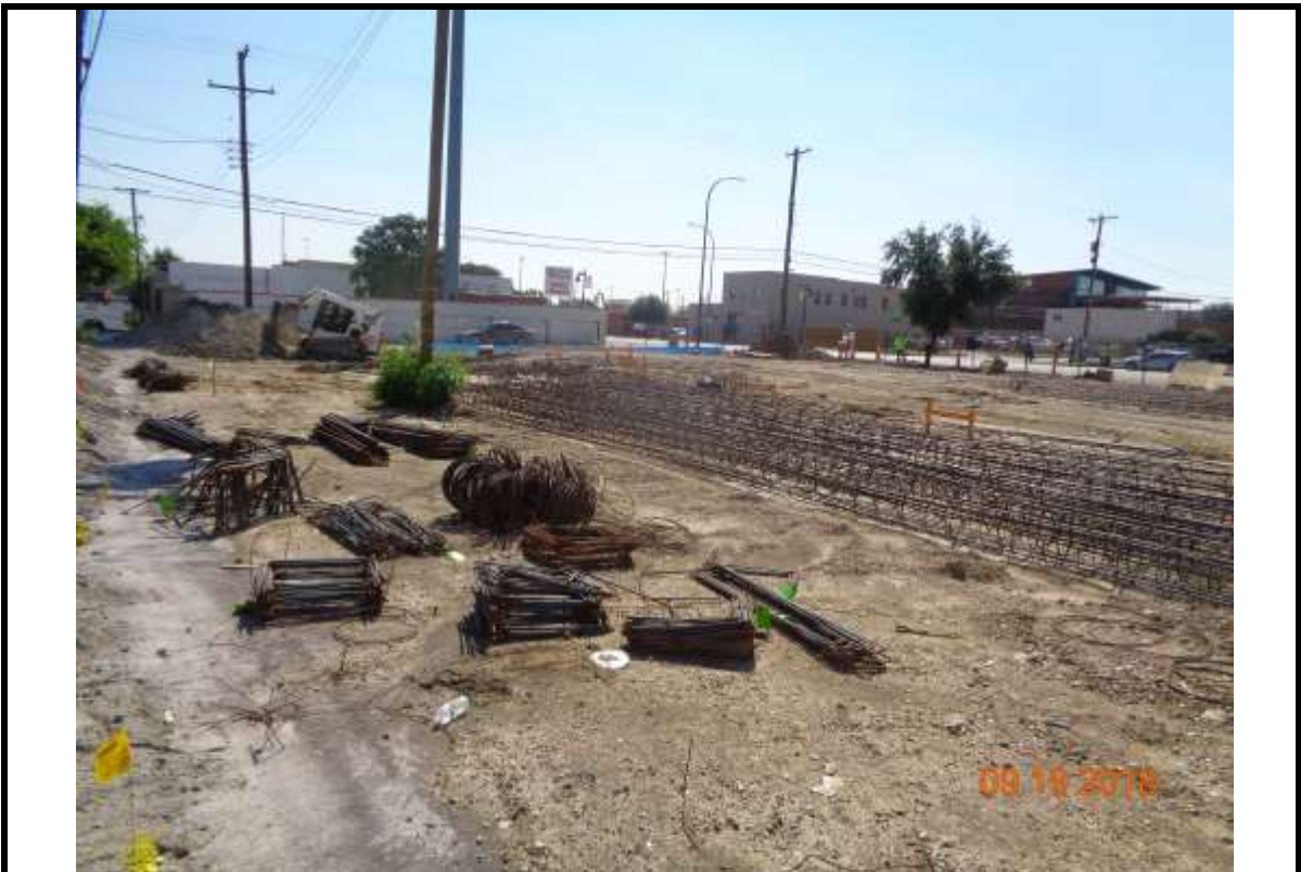
Photograph 4: Full length pier reinforcing steel cages staged for cutting and placing.
