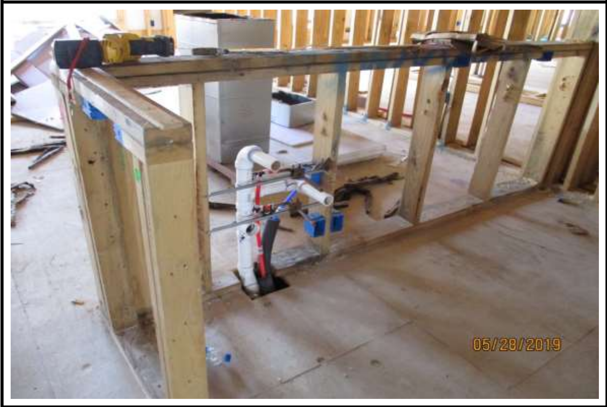
Photograph 5: Plumbing rough-in 3 th floor at Building "A".
