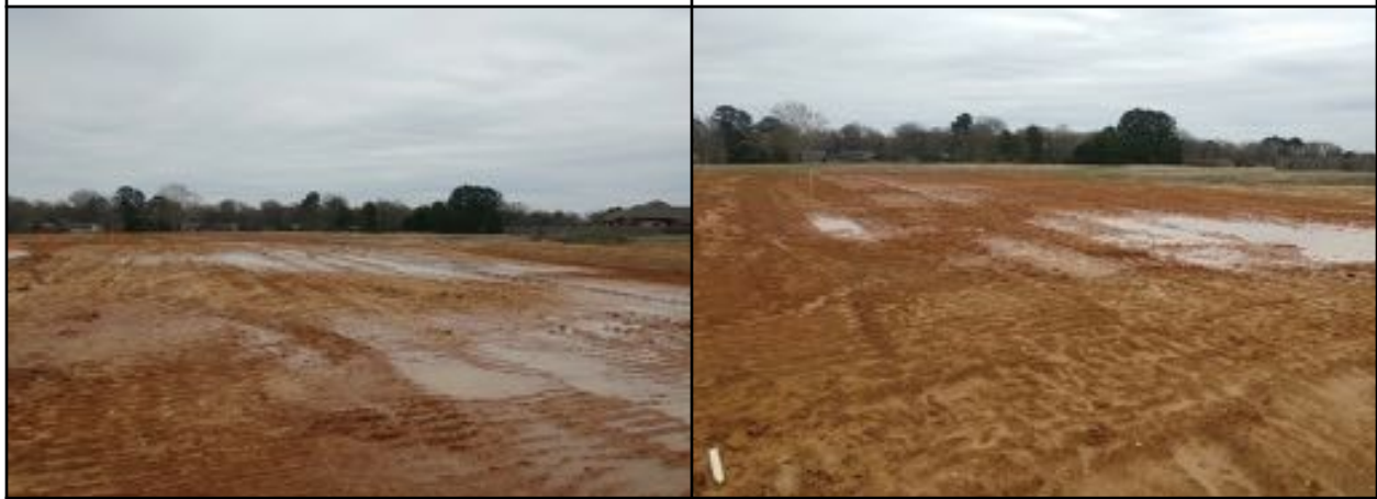
Photo # 11 View of building 6 pad
