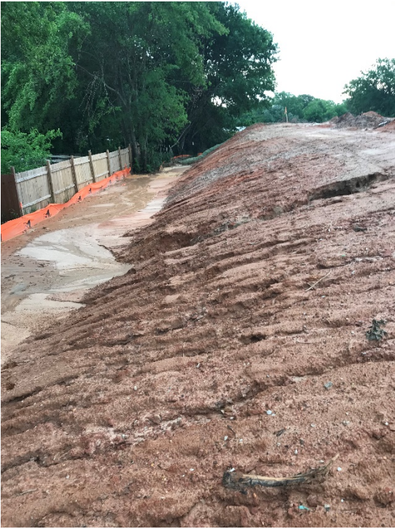
IMG 91 –Rain soaked and washed away dirt around form boards....all has to be replaced when dried out.
