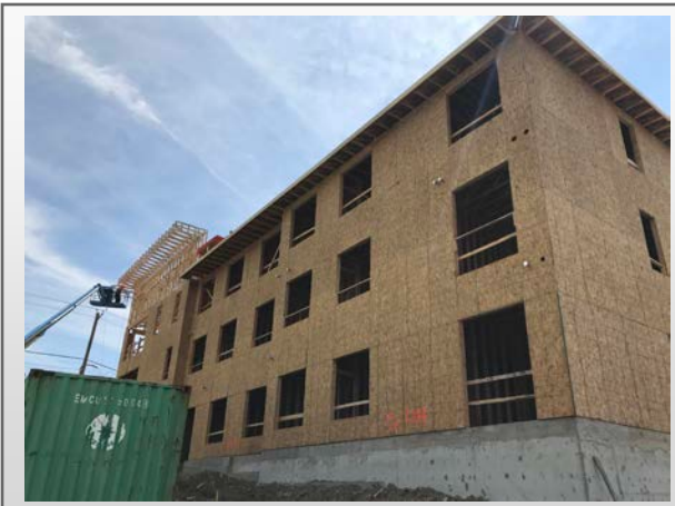
Building B Exterior
