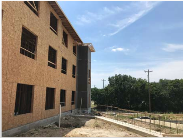
Building B Courtyard
