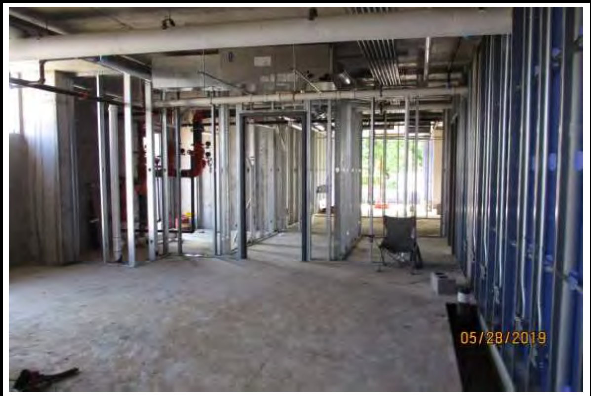
Photograph 9: Metal stud framing in Administration Area at Building "B".
