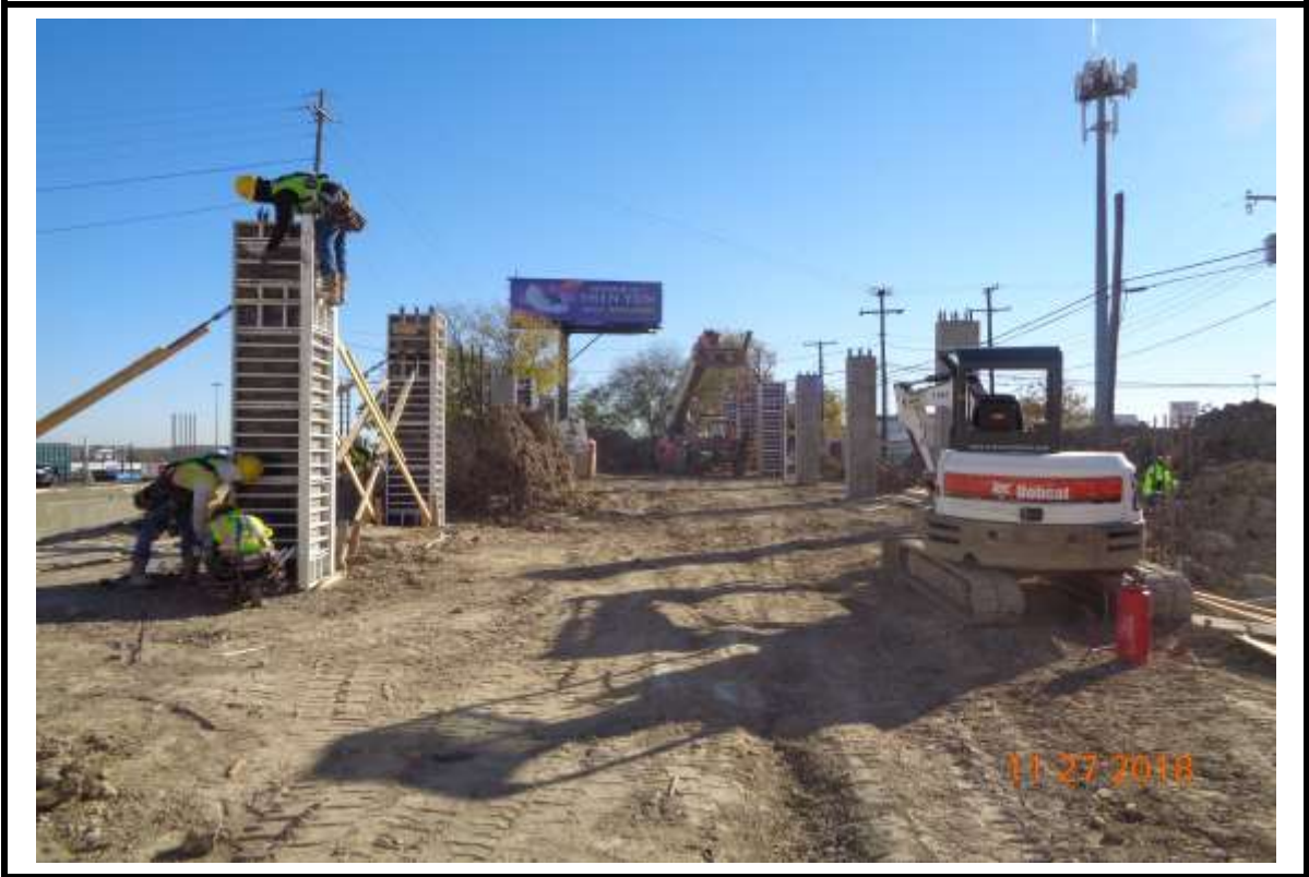
Photograph 3: Plumbing column forms at Building “B”.
