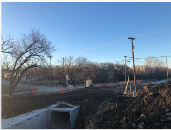
Box Culvert In Progress
