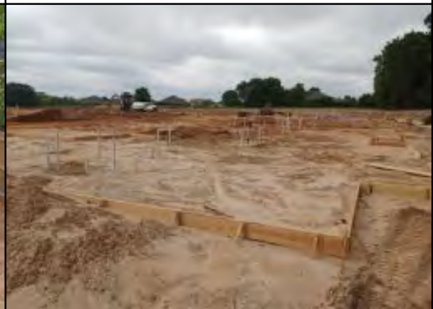
Photo # 12 Building pad 2 overview- underground plumbing complete and forms set
