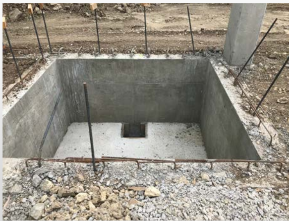
Elevator pit at Building B
