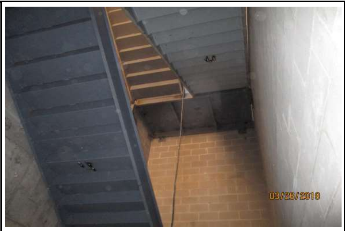
Photograph 4: Stair installation at Building "A".
