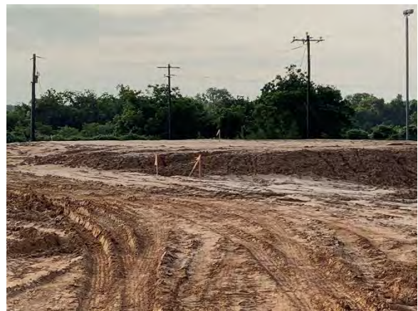
Photo 6: Pad preparation at Building 3.
