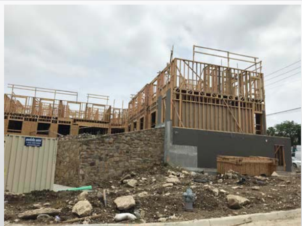
Retaining wall and stair tower – Building B
