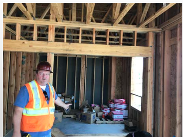
Building B Interior
