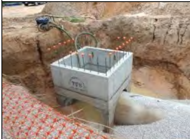
Photo # 3 Draining of storm drain utilities in-progress
