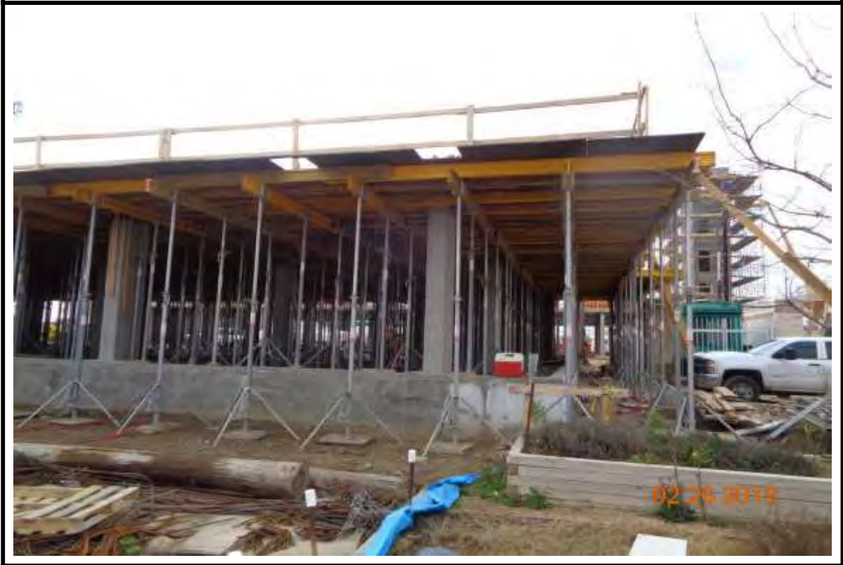
Photograph 9: Shoring ready to “wreck” at Building “B” West end.
