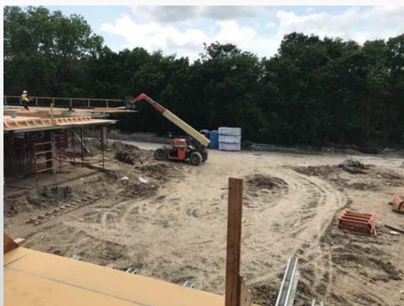
Looking West across site from Building A
