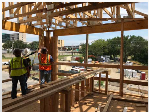
Building B C2 unit
