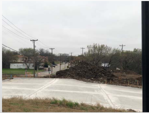
Corner of Bldg. B, Beckman Rd. looking west
