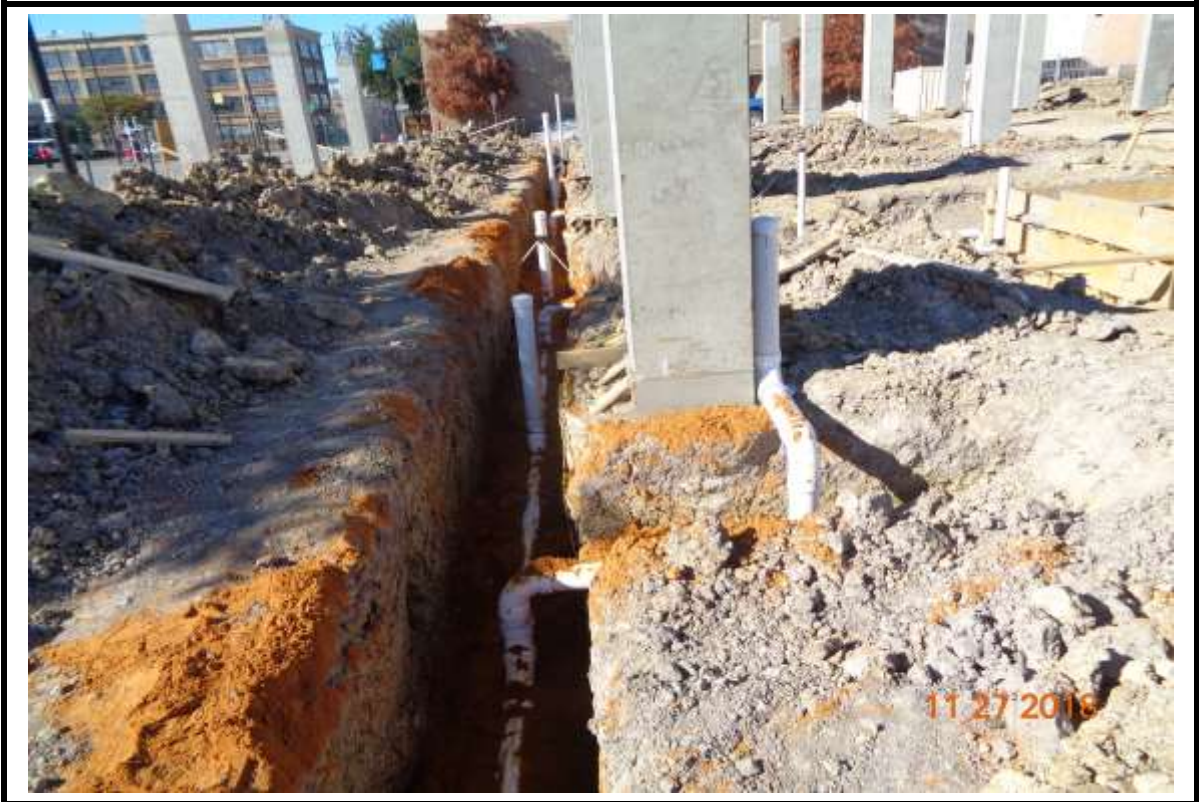
Photograph 9: Sanitary line bedded and ready for backfill.
