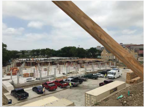
Concrete podium and concrete columns Building A
