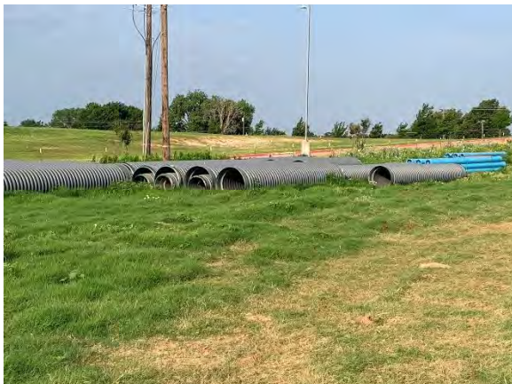
Photo 11: Stocked storm sewer piping.
