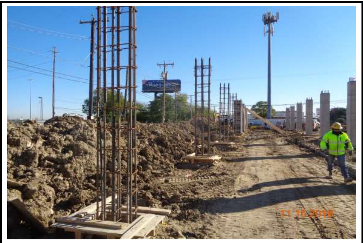
Photograph 6: Last seven columns at the North grade beam at Building "A".
