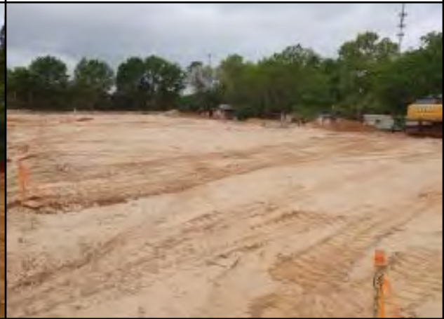
Photo # 10 Building pad 1 overview - staking has occurred
