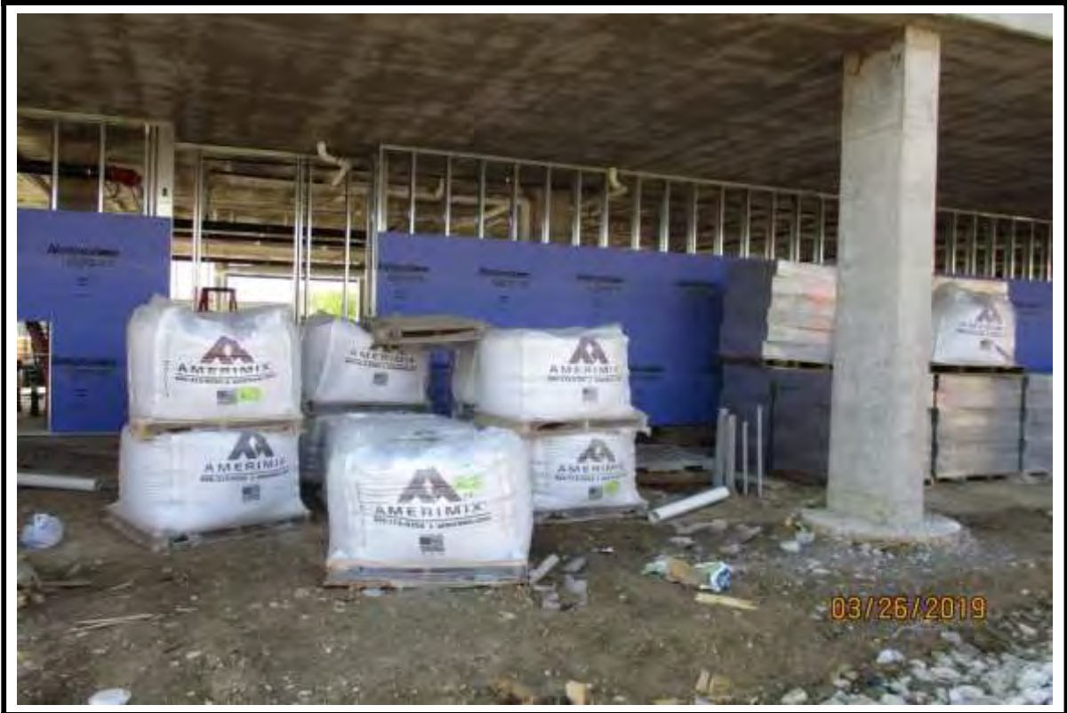
Photograph 2: Premixed mortar staged for masonry installation.
