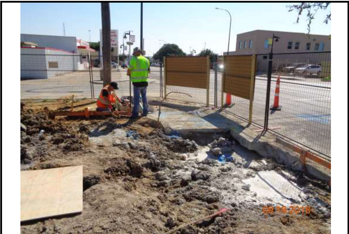
Photograph 8: City water crew relocating existing water meter.
