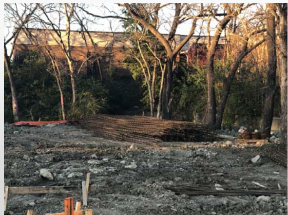
Building A rebar storage
