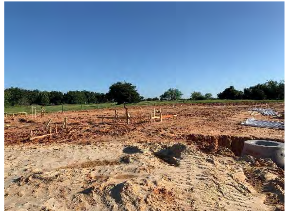
Photo 10: Completed batter board installation at Building 7.
