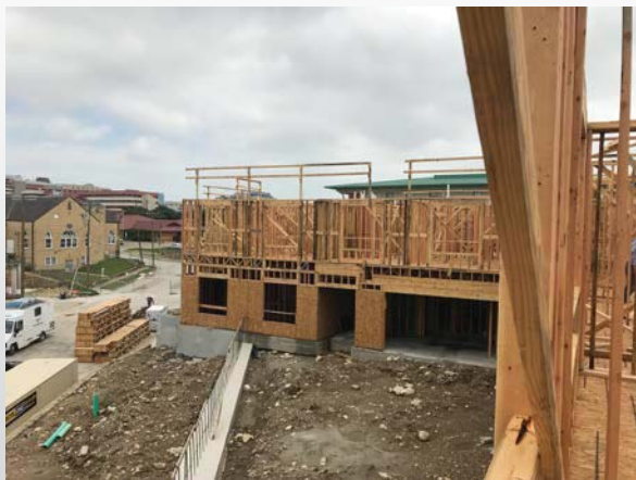
Courtyard Building B
