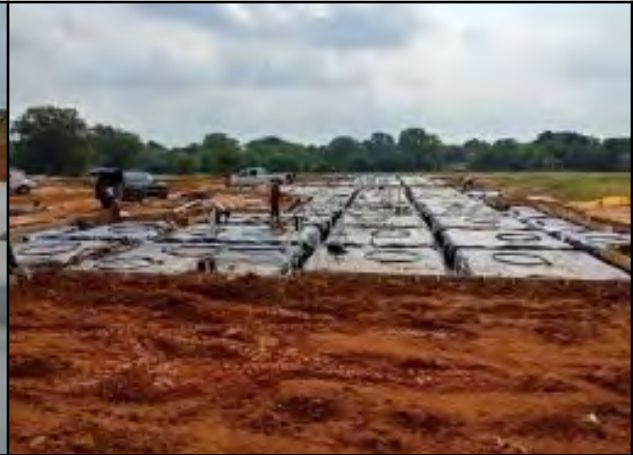
Photo # 14 Building 6 - Footings excavated and install of post-tensioned cables in-progress
