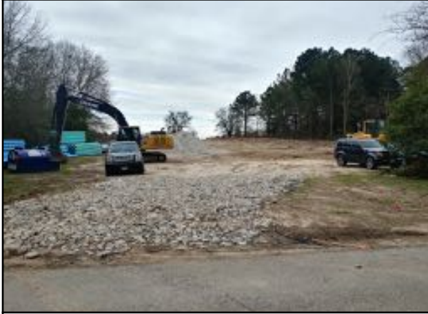
Photo # 1 Site Entrance
