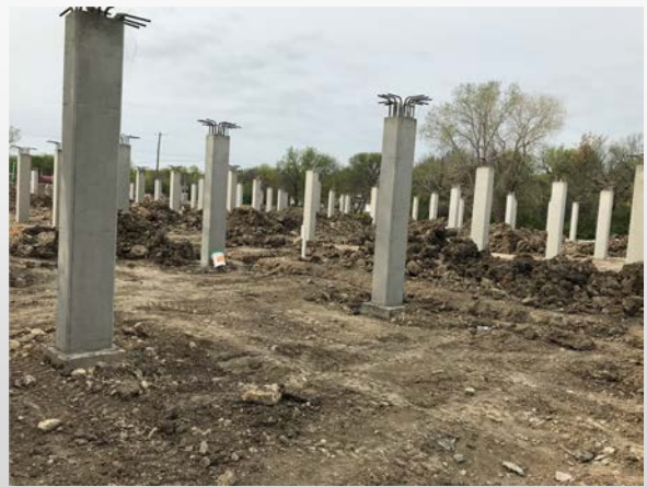
Podium columns at Building B
