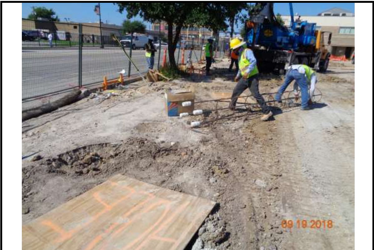
Photograph 6: Dressing a pier cage for installation.
