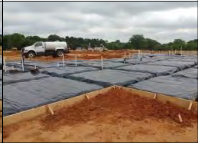
Photo # 16 Building pad 5 - Footings excavated
