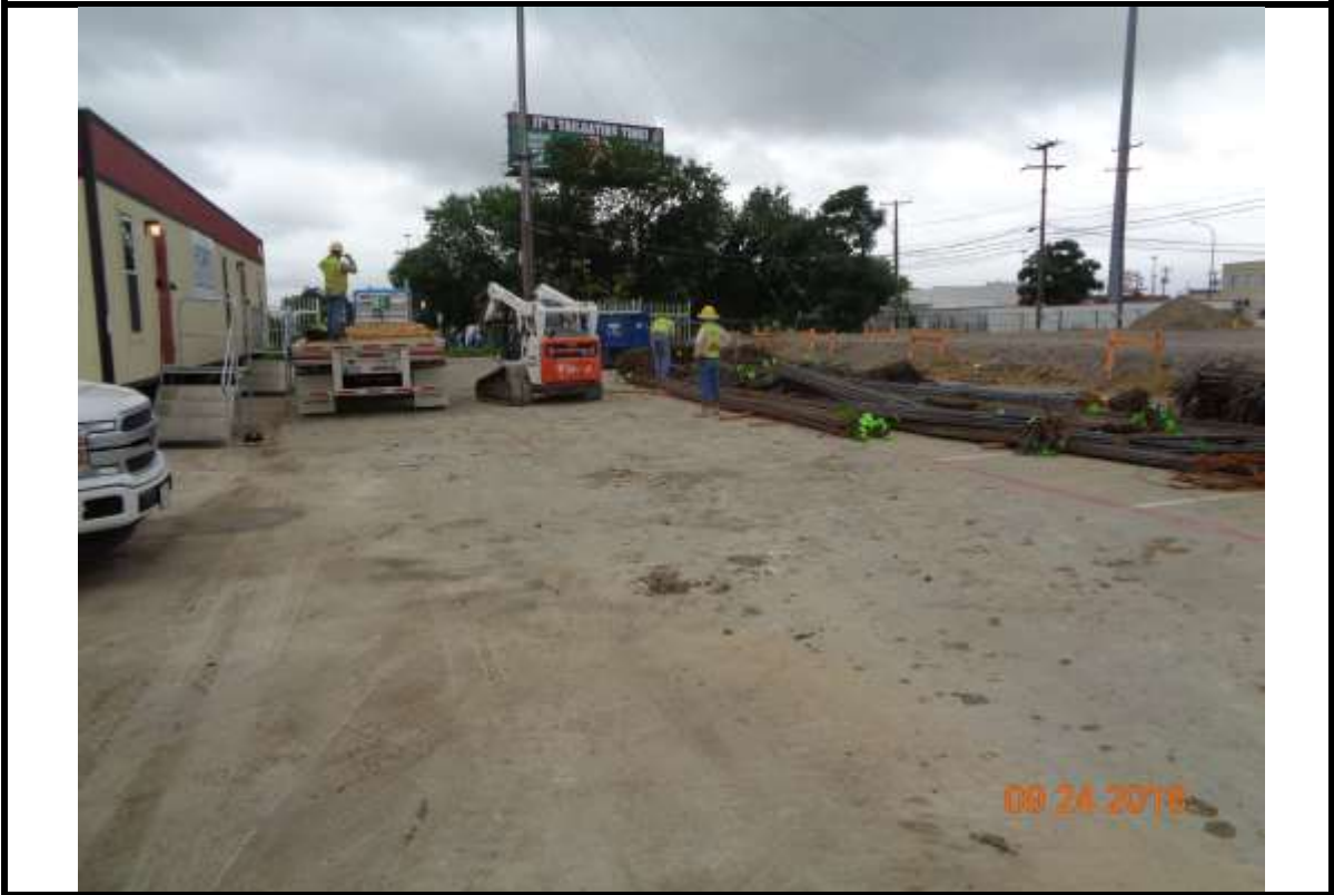
Photograph 11: Off loading grade beam reinforcing steel.
