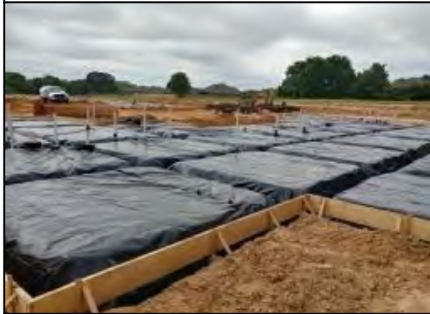
Photo # 15 Building pad 4 - Footings excavated
