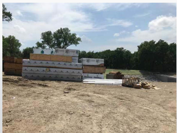
Stored Framing Material
