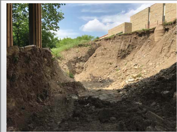
Excavation under Rosedale
