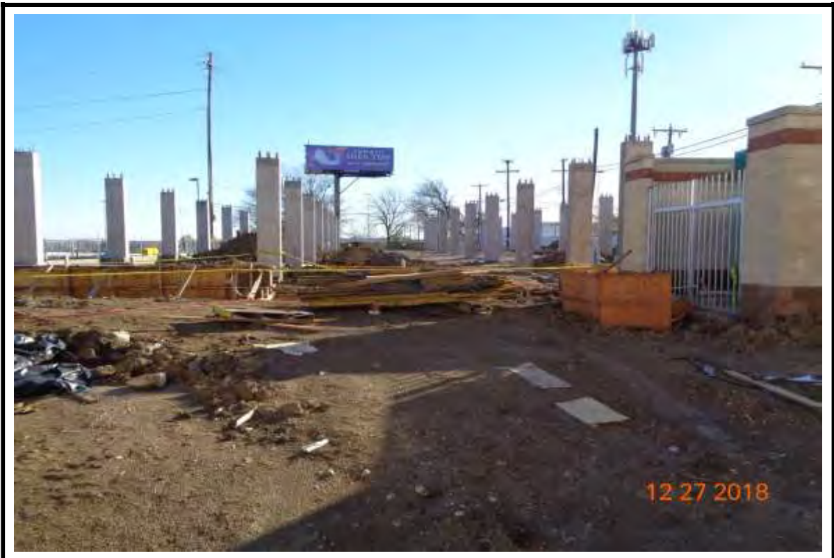
Photograph 1: Balance of grade beam forming at Building "B".
