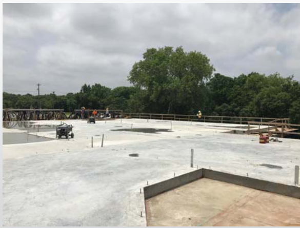
Top of Podium Building A
