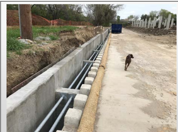
Drainage along Fire Lane
