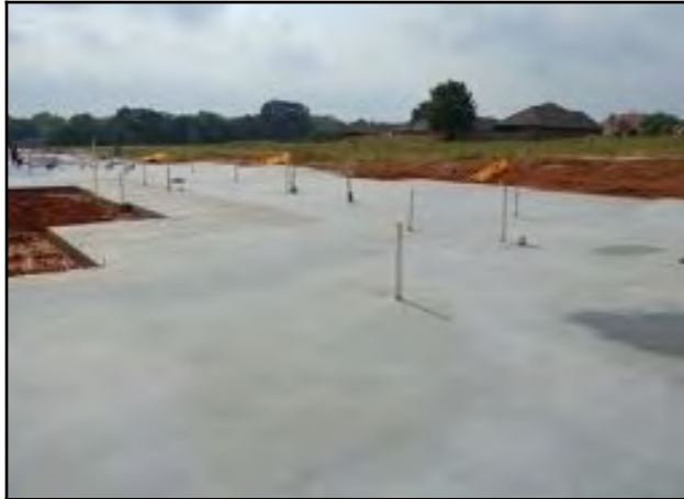
Photo # 13 Building 5 - Building slab complete
