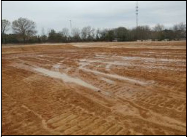
Photo # 13 View of building 8 pad
