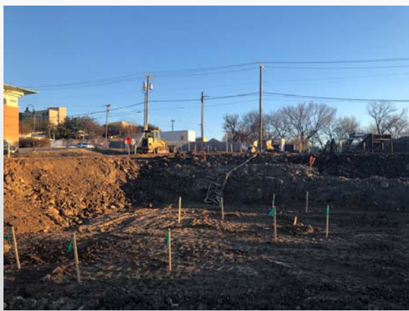
Beckman Rd. on far left building B foundation pad prep underway
