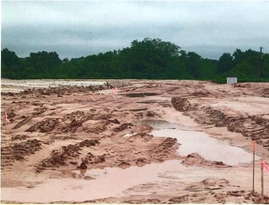
Current site status after the rain
