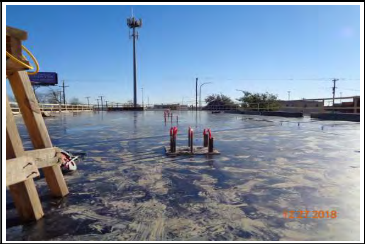
Photograph 5: Plastic faced plywood forms for Podium Deck at Building "A".
