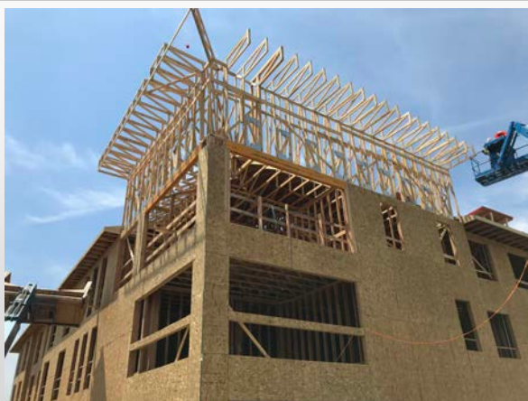
Building B Framing
