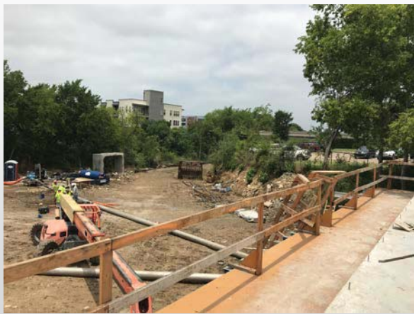
Looking North across site from Building A
