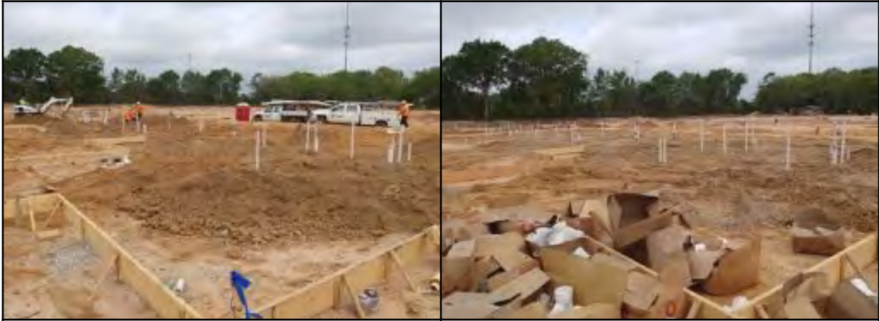
Photo # 19 Building pad 8 - Form boards set and underground plumbing complete
