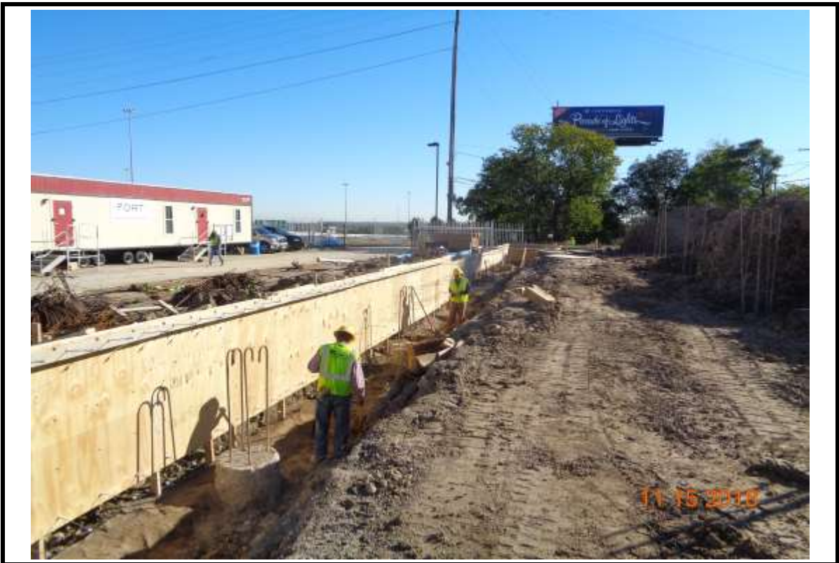
Photograph 2: Preparing beam bottom at South grade beam at Building "B".
