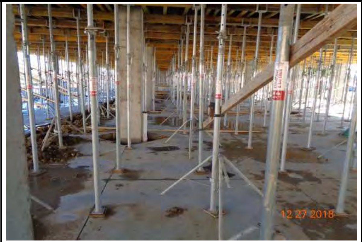
Photograph 3: Shore jacks for Podium Slab at Building "A".
