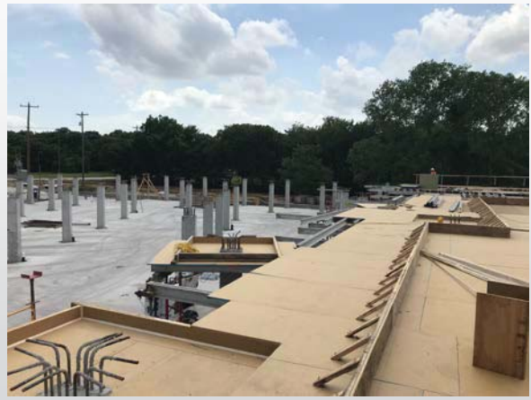
Building A Podium forming
