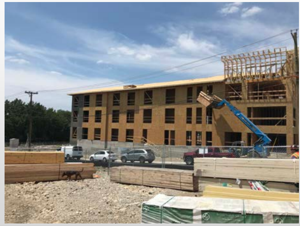
Building B Framing
