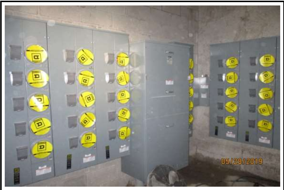
Photograph 8: Meter base installation at Building "B".
