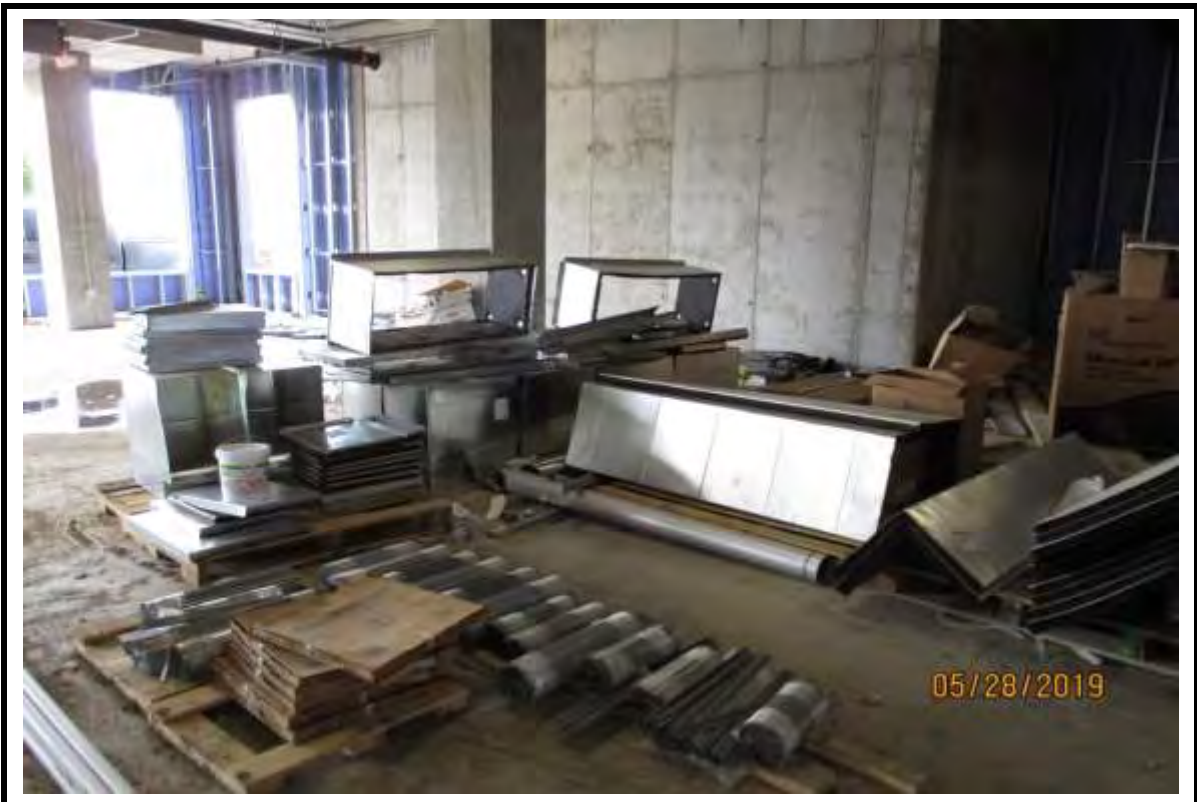
Photograph 2: HVAC duct work materials staged for installation Building "A".
