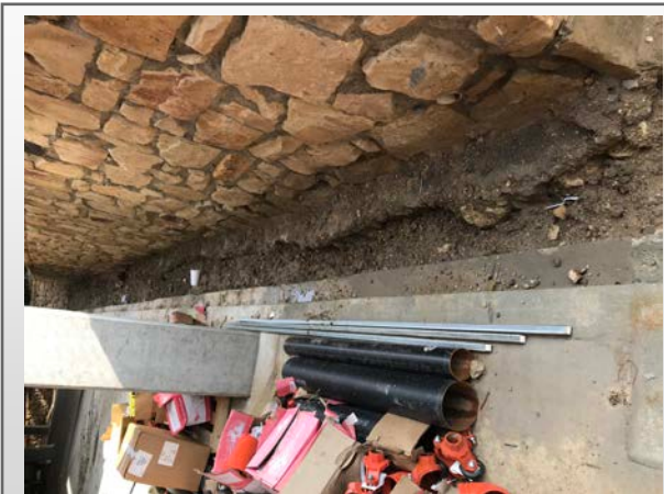
Space between retaining wall at Building A
