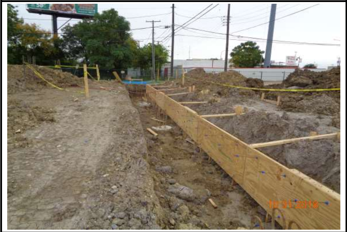
Photograph 3: Beam forms at South grade beam Building "B".
