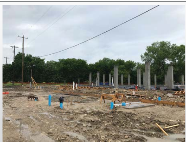
Building A columns
