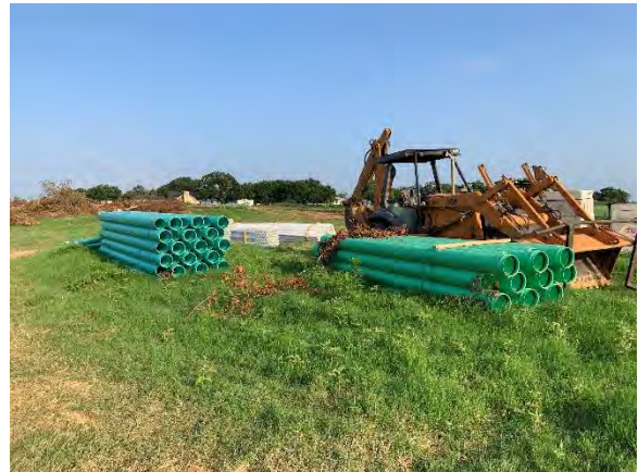
Photo 10: Stocked sanitary sewer and underslab plumbing piping.
