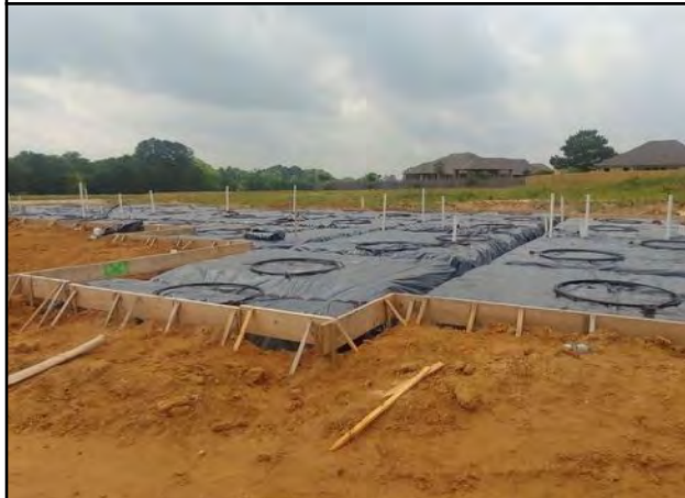
Photo # 15 Building 7 - Footings excavated and install of post-tensioned cables in-progress
