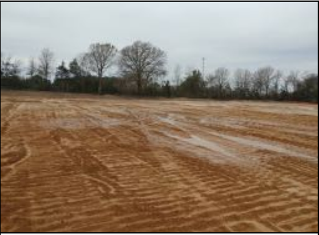
Photo # 14 View of building 9 pad
