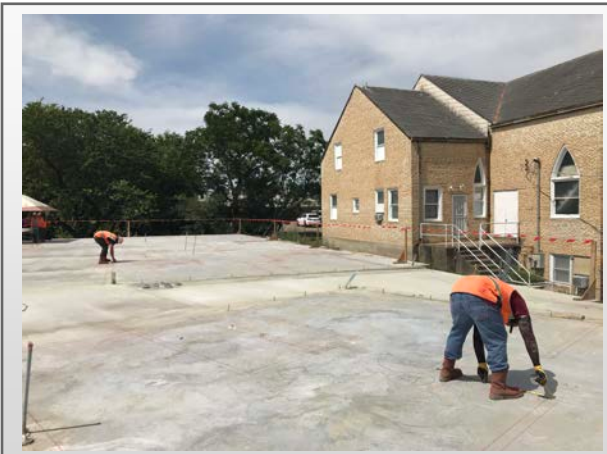
Building A Podium
