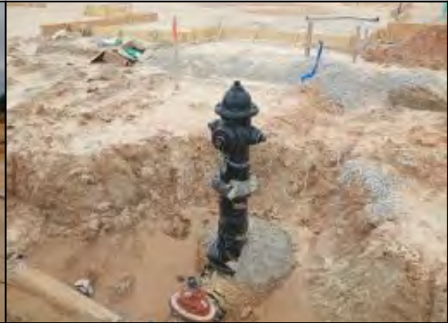
Photo # 14 Installed fire hydrant
