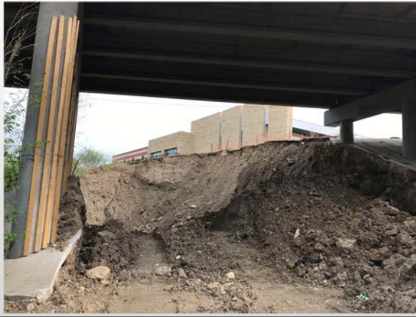
Earthwork under bridge
