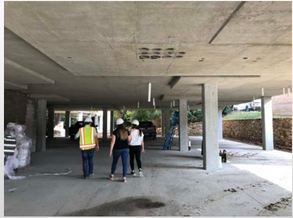
Parking level under podium at Building A
