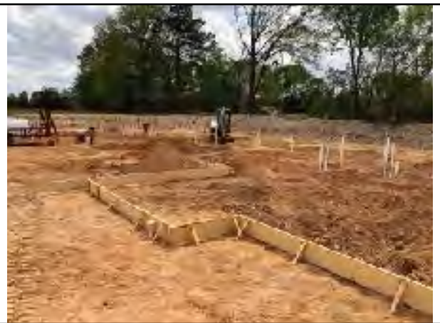
Photo # 12 Underslab plumbing complete at Building 4
