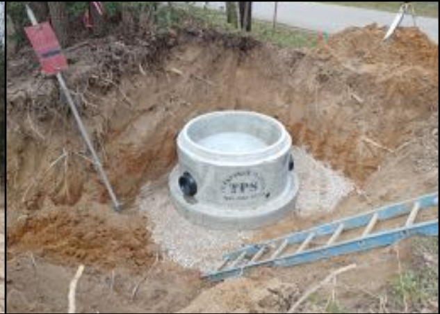
Photo # 4 View of Excavation and gravel placement for sewer manhole
