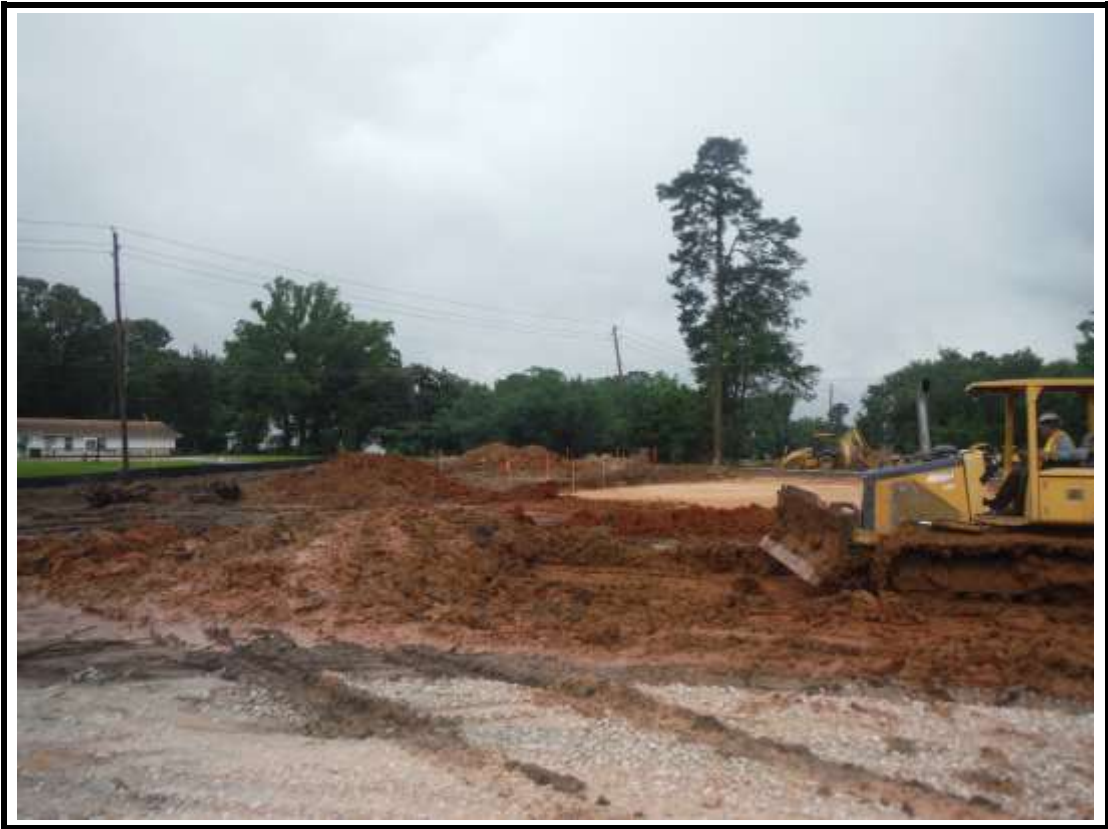
Photograph 1: Site work at entrance.
