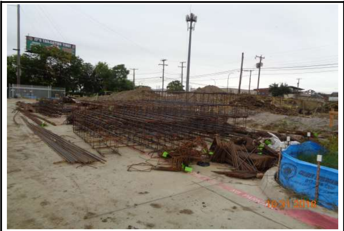
Photograph 1: Podium column and pier cap reinforcing.
