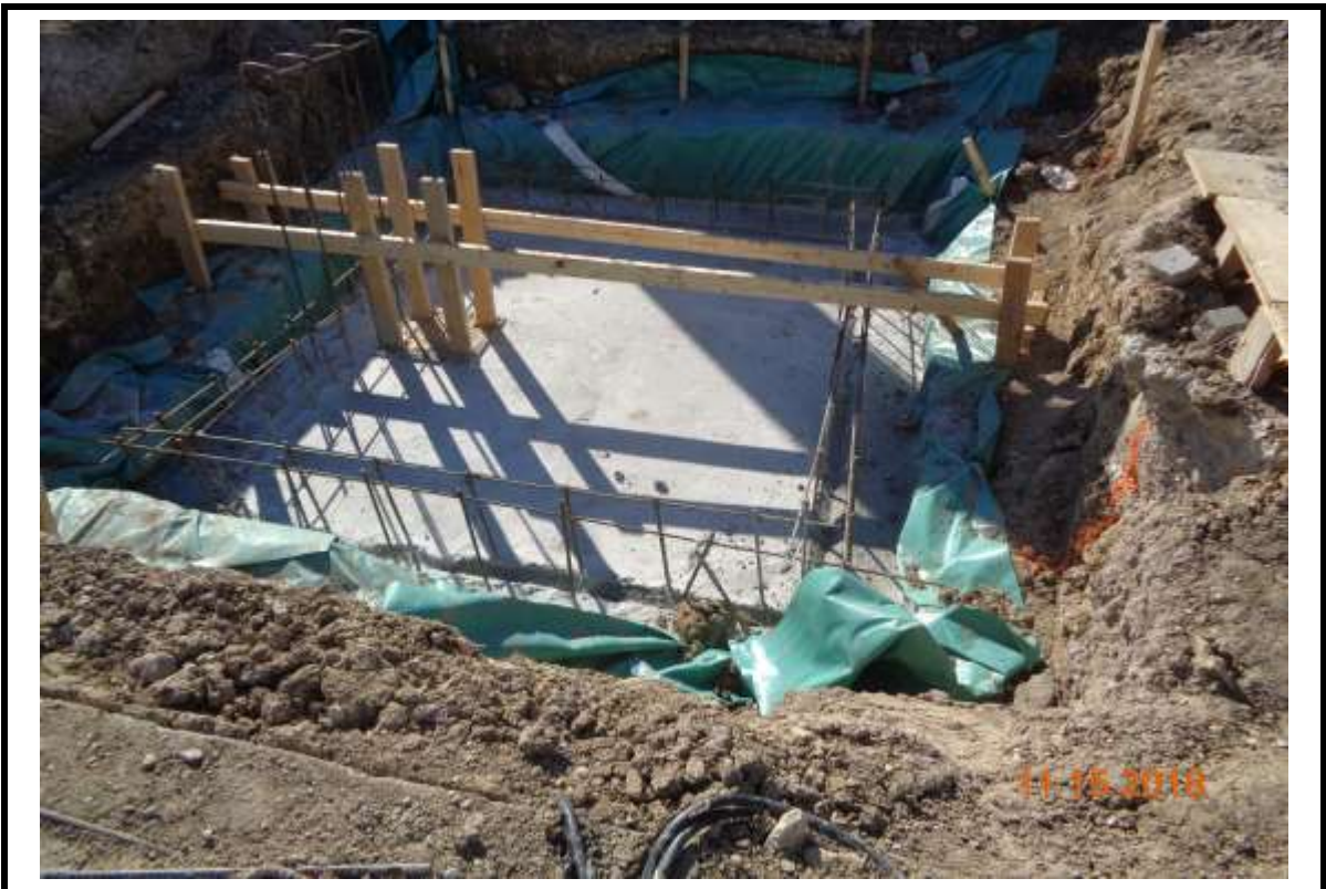
Photograph 4: Elevator pit slab at Building "A".
