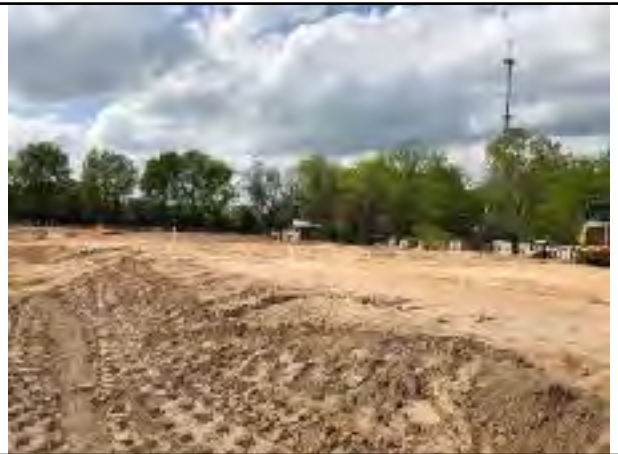
Photo # 10 View of established building pad 1
