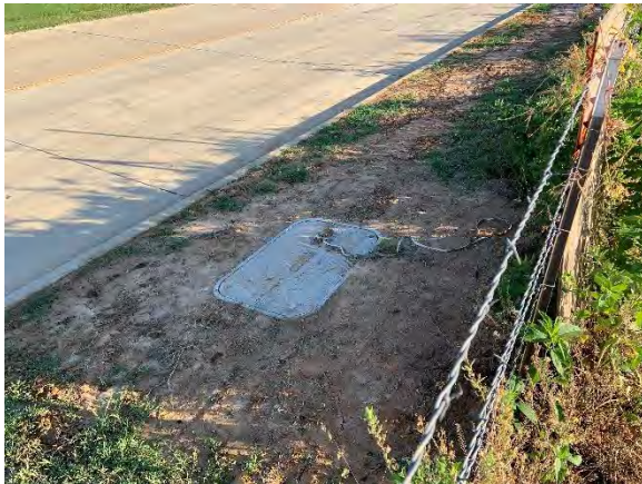
Photo 1: Completed communication box relocation along Buchanan Rd. (by others).
