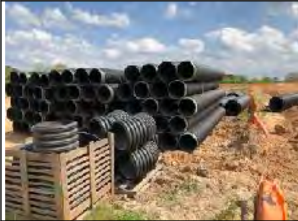
Photo # 19 Storm drainage pipe stored on site
