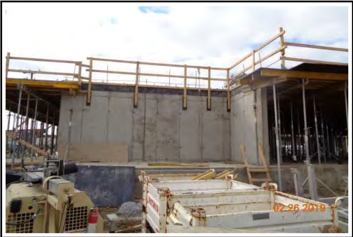
Photograph 10: Completed Stairwell wall at Building “B” East end first level.
