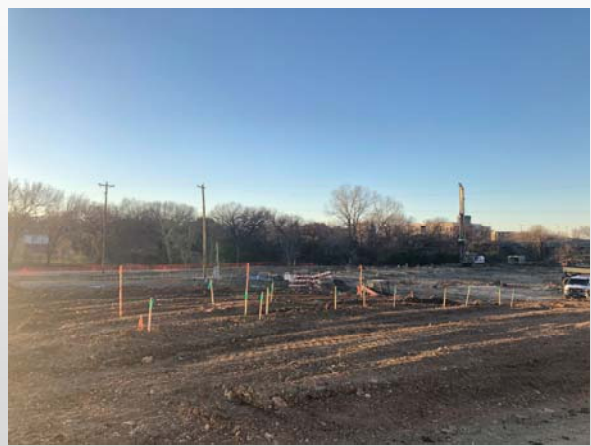
Building B staking
