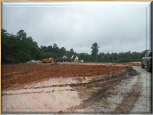
Site entrance with earth work in progress.
