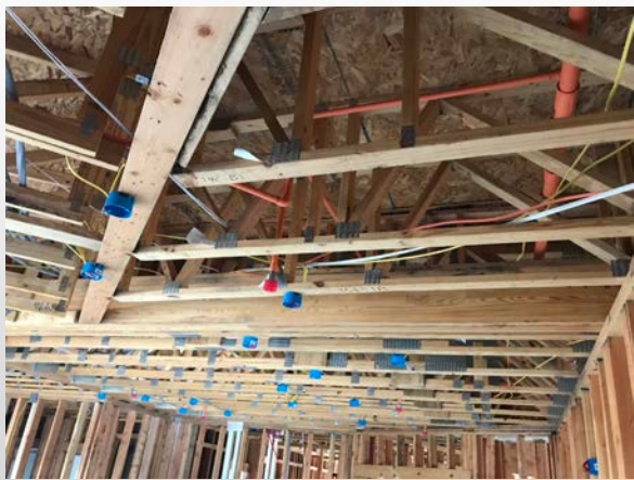
Truss space above clubhouse
