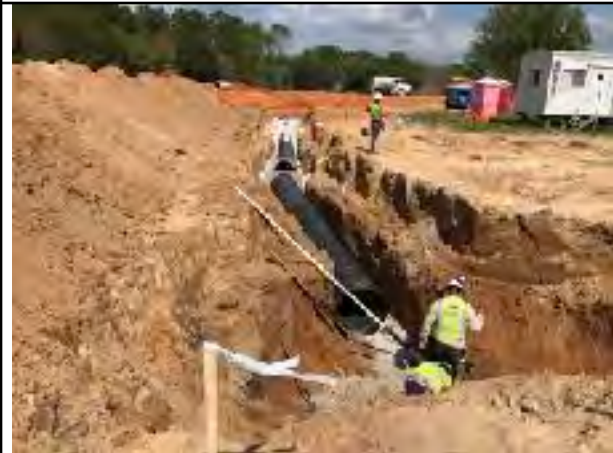
Photo # 3 Install of storm drainage in progress throughout site
