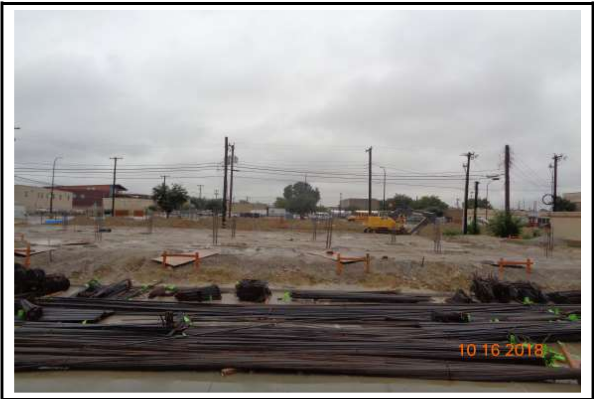
Photograph 1: Overall of site with grade beam and podium reinforcing in foreground.
