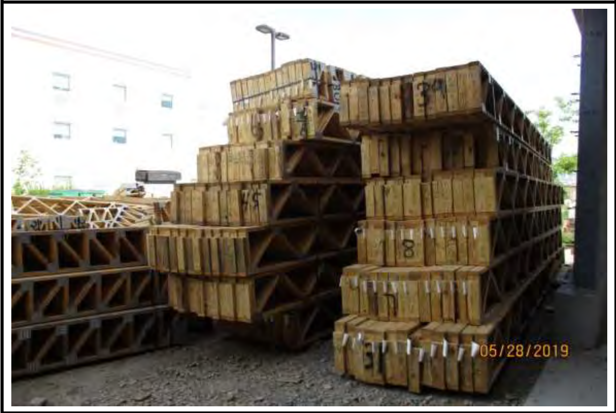
Photograph 7: Floor trusses staged for 4 th floor at Building "B".
