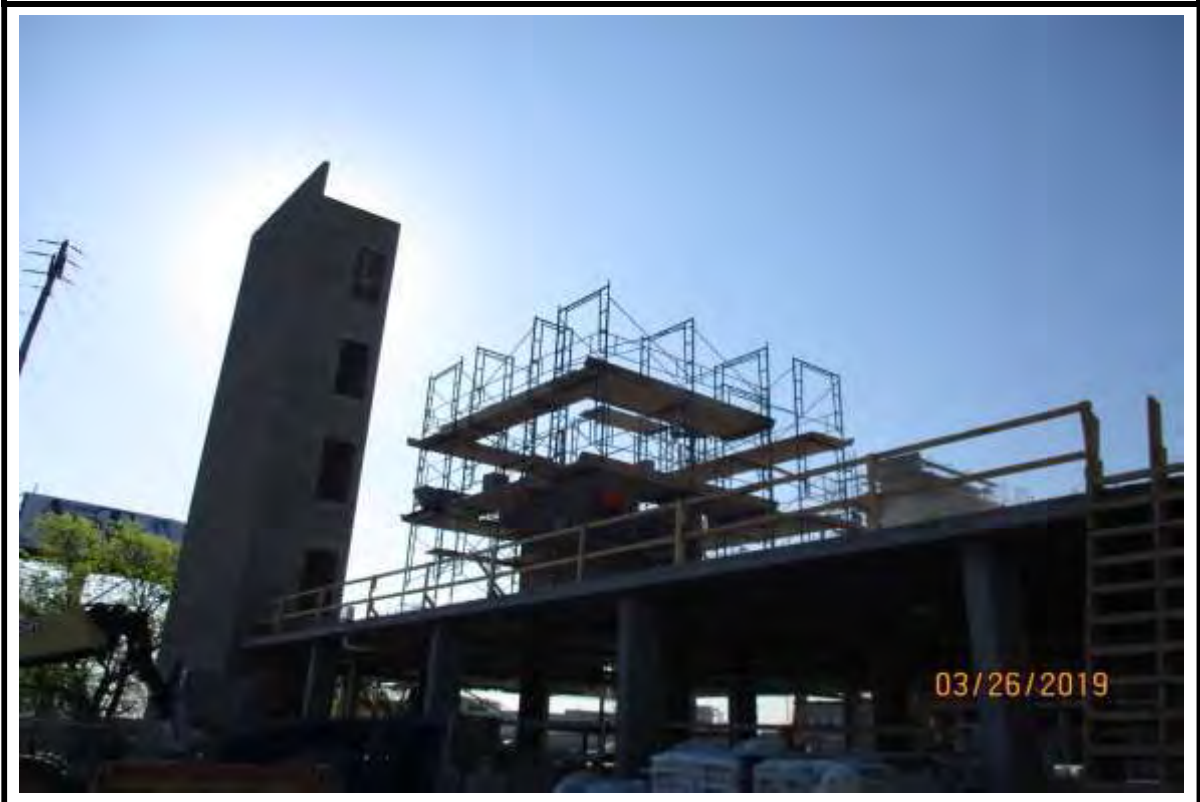
Photograph 5: Elevator shaft masonry at Building "B".
