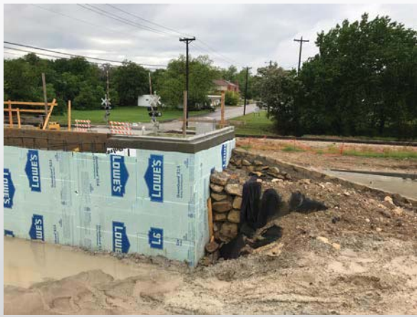
Retaining wall at Building B
