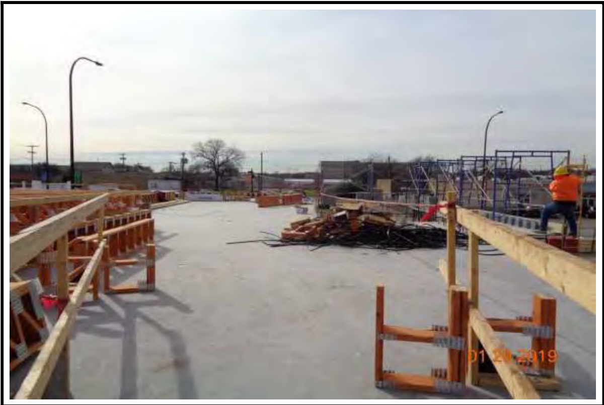
Photograph 8: Installation of sub-floor joists on Building “A” Podium Deck.
