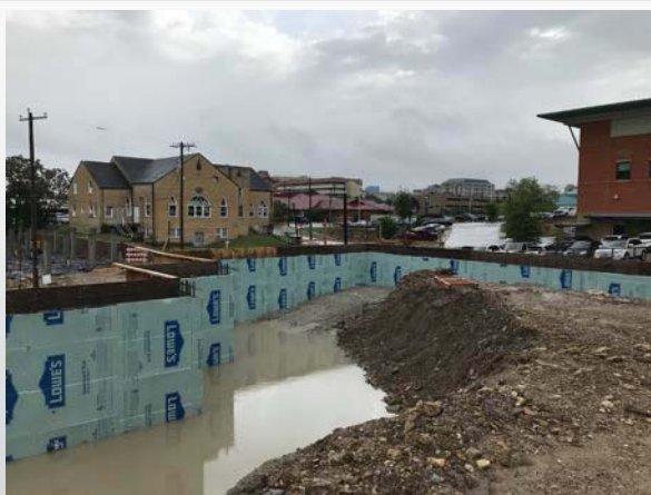
Retaining wall at B
