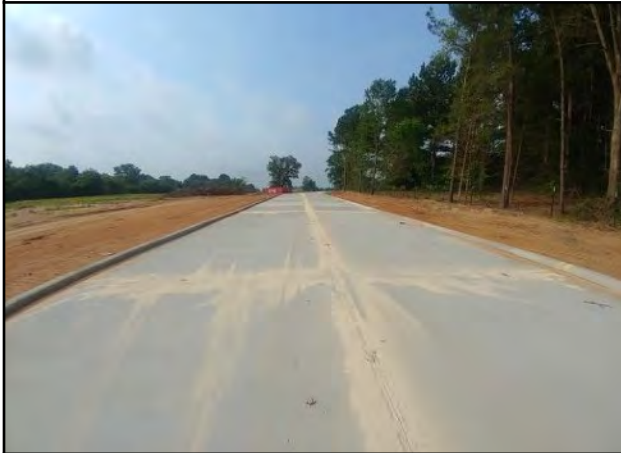
Photo # 3 View of concrete paving at Sunset Drive
