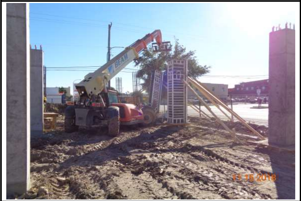
Photograph 5: Setting column forms South grade beam at Building "A".
