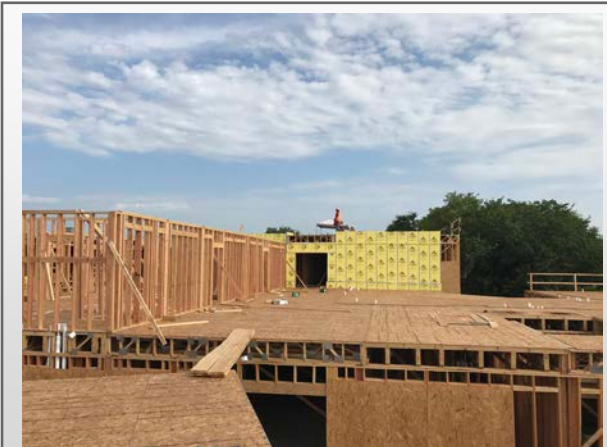
Framing at Building A
