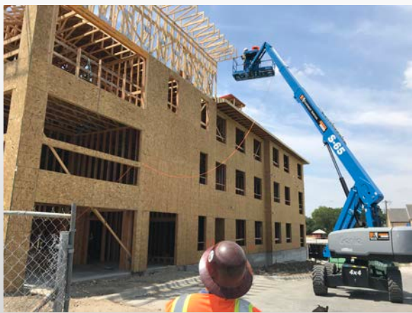
Building B Framing
