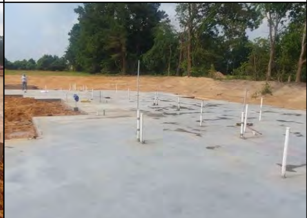
Photo # 12 Building 4 - Building slab complete
