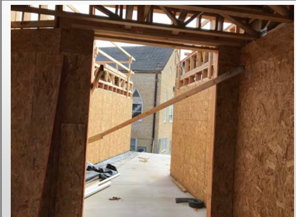
Framing on Building A
