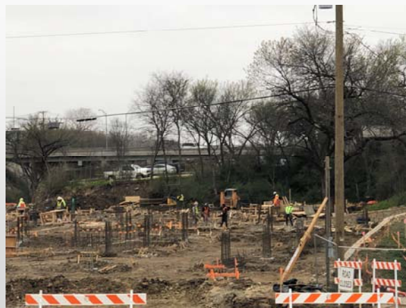
Ongoing progress at Bldg. A drilled piers
