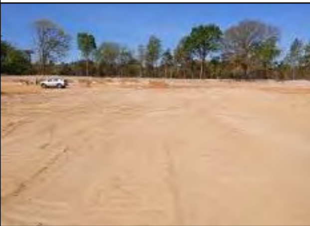
Photo # 18 View of established building pad 9
