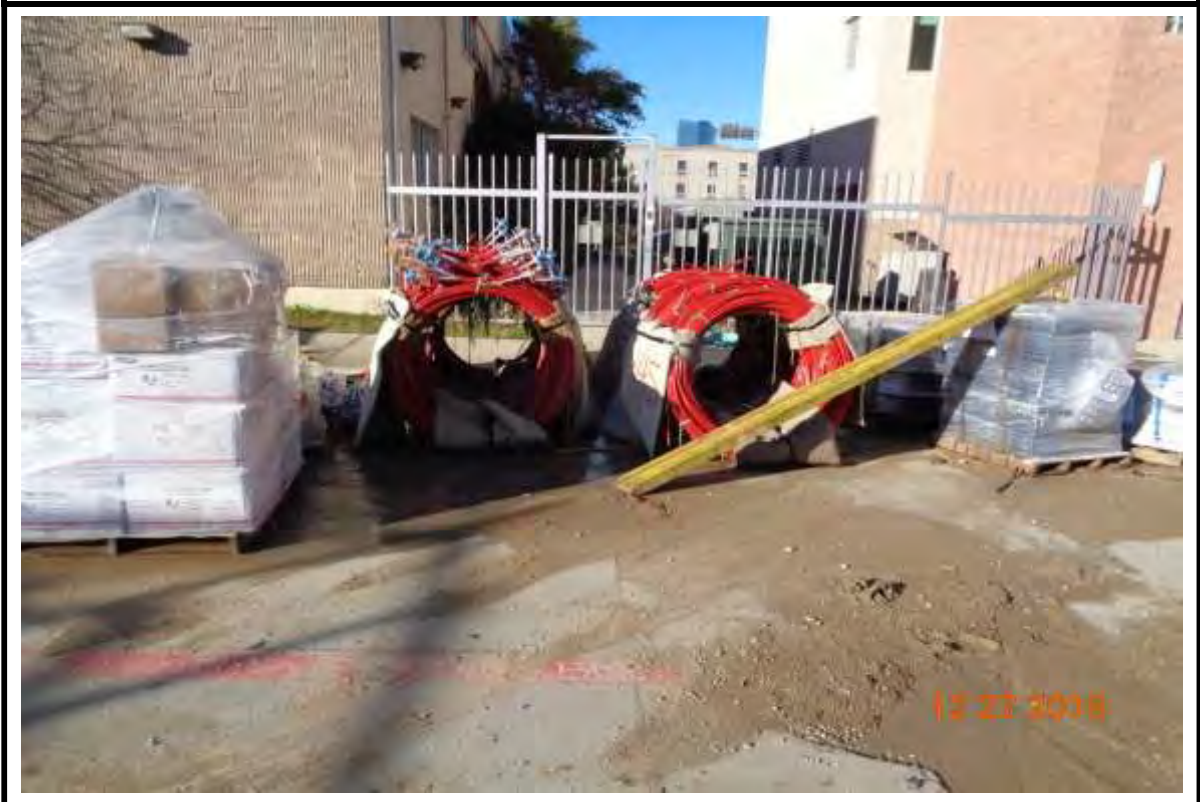
Photograph 7: Post tension tendons for installation at Building "A" Podium Deck.
