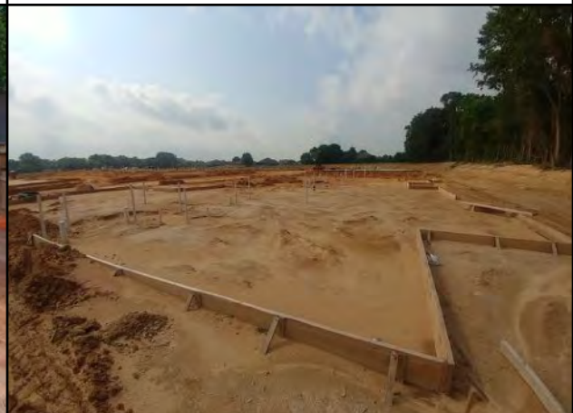
Photo # 10 Building 2 - Forms and under slab plumbing complete
