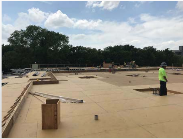
Building A Podium forming
