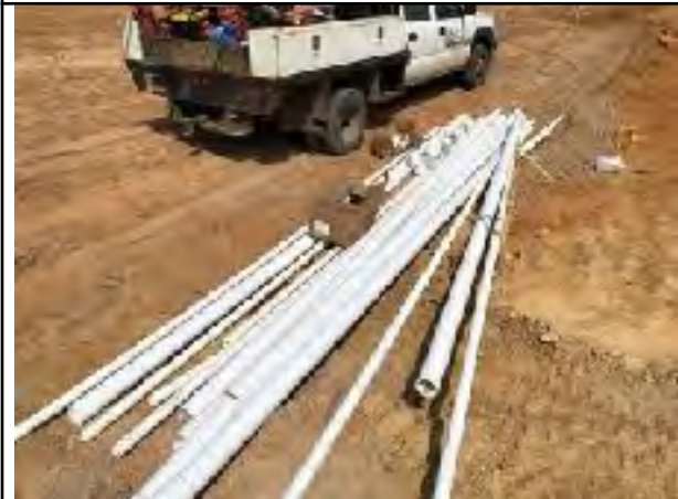
Photo # 21 PVC drainage pipe stored on site
