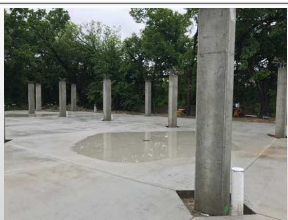
Building A parking
