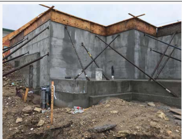
Building B Stair walls
