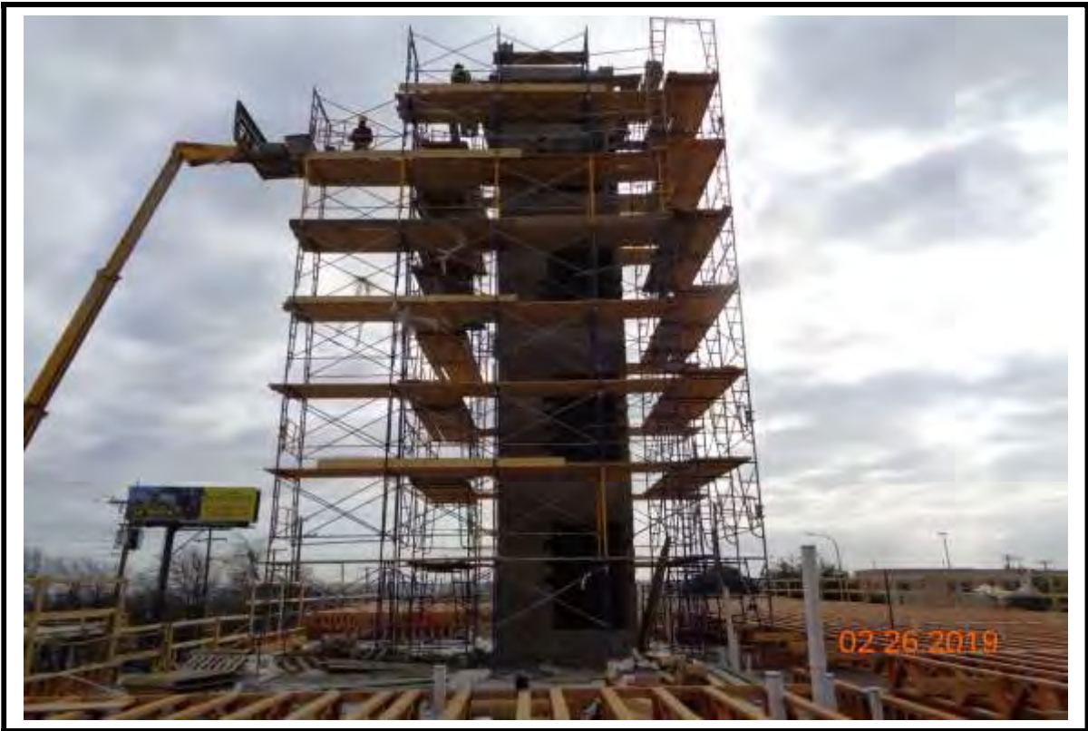
Photograph 2: Elevator shaft top-out at Building "A".
