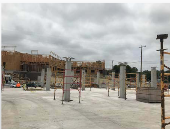
Columns – Building A
