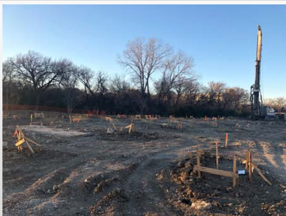
Building A Drilling piers in progress
