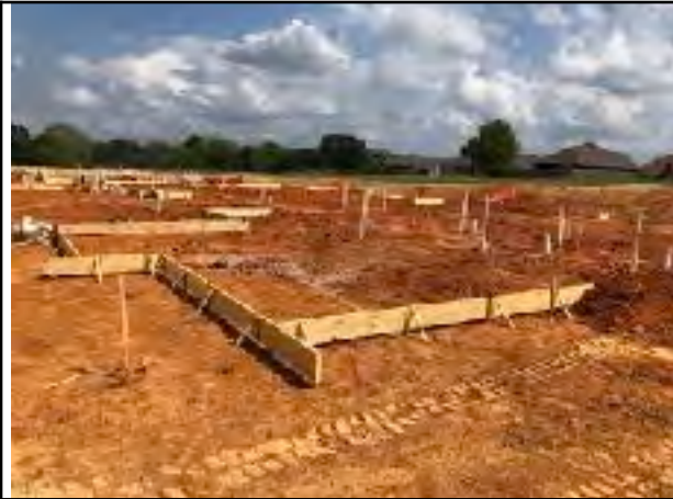
Photo # 13 Underslab plumbing complete at Building 5
