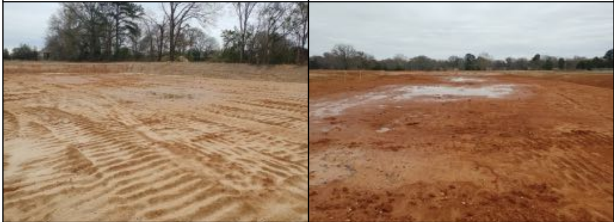
Photo # 9 View of building 4 pad
