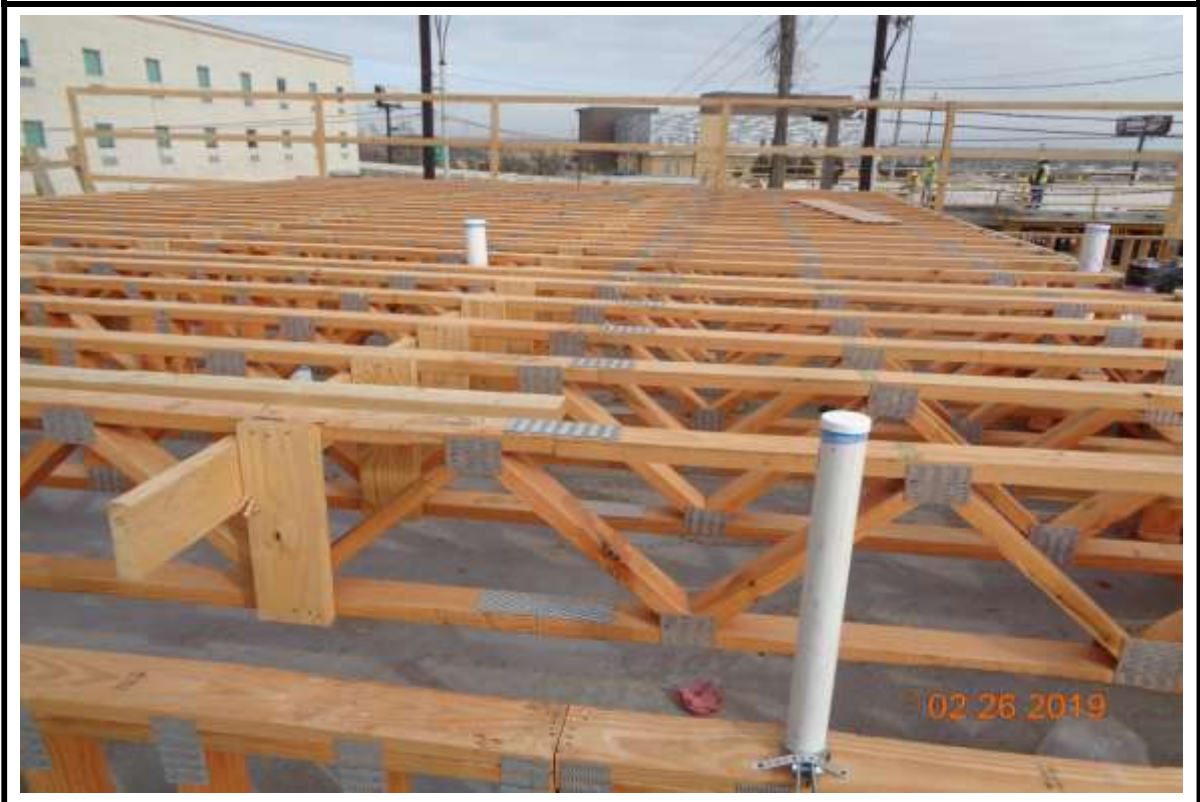
Photograph 7: 2 nd Level floor structure over Podium Deck at Building "A".
