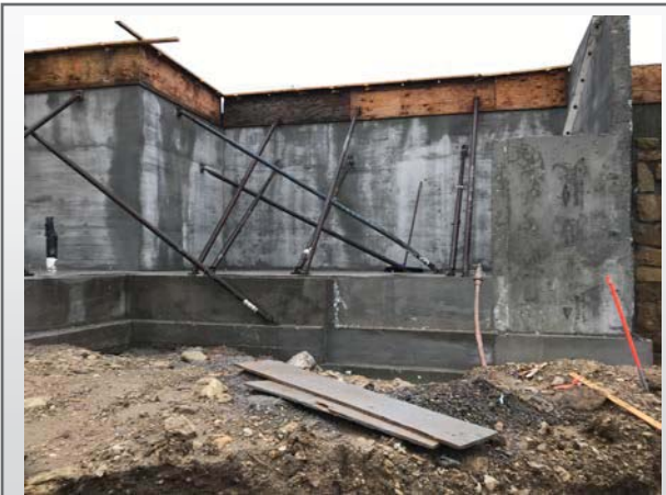
Building B Stair walls
