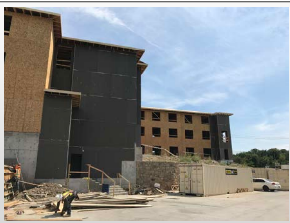
Building B Exterior
