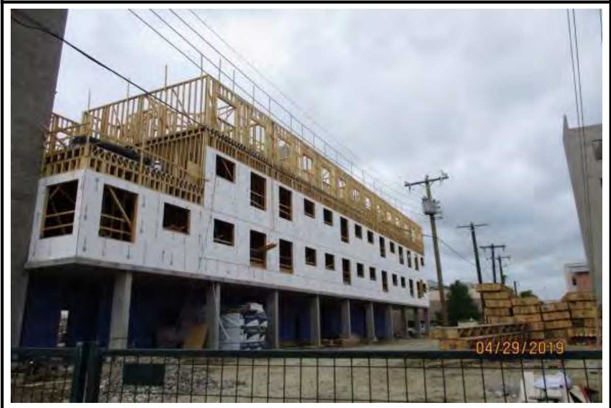
Photograph 5: Wood framing to 4 th floor at Building "A".
