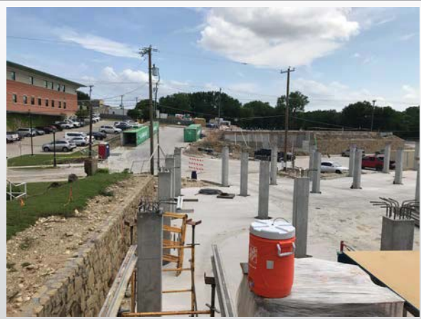
Building A along retaining wall
