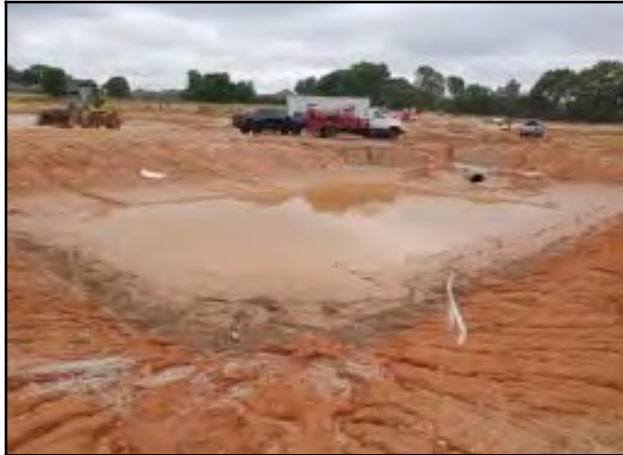
Photo # 7 Detention pond overview
