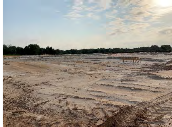
Photo 8: Completed surveying and corner staking at Building 12.
