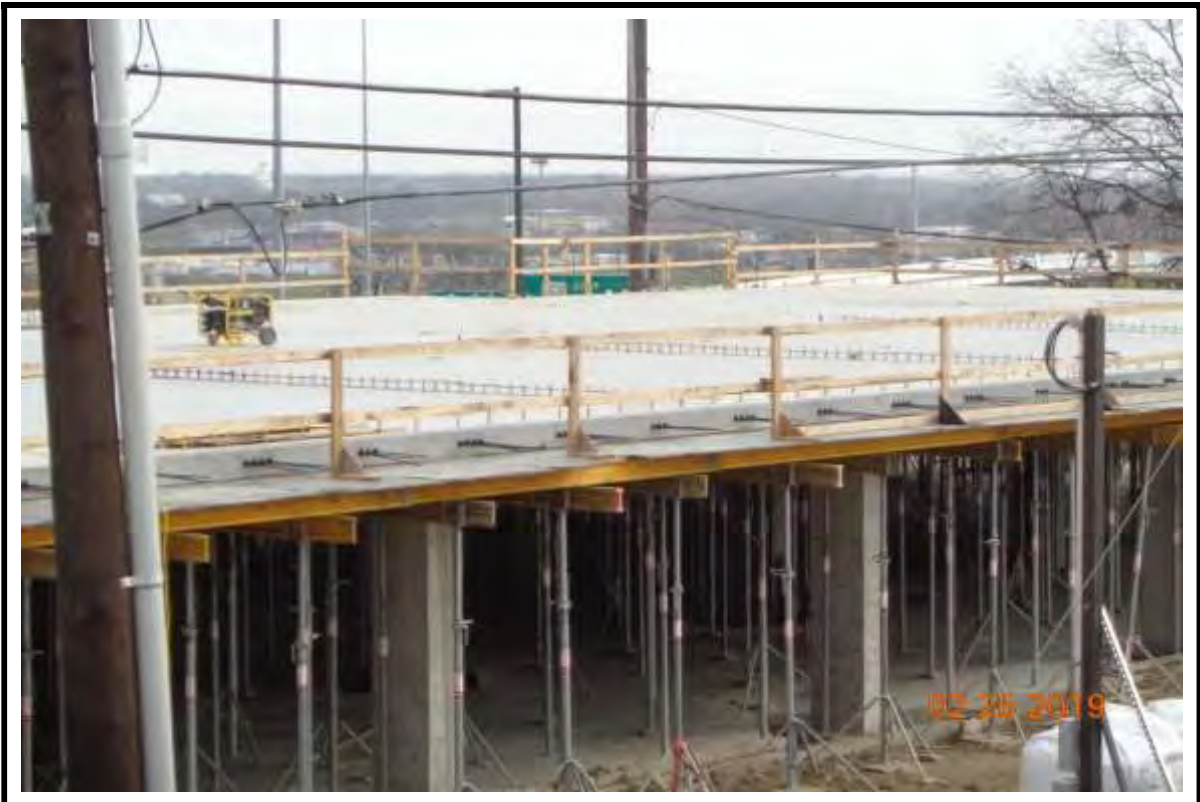
Photograph 8: Building "B" Podium Deck with concrete placed and finished.
