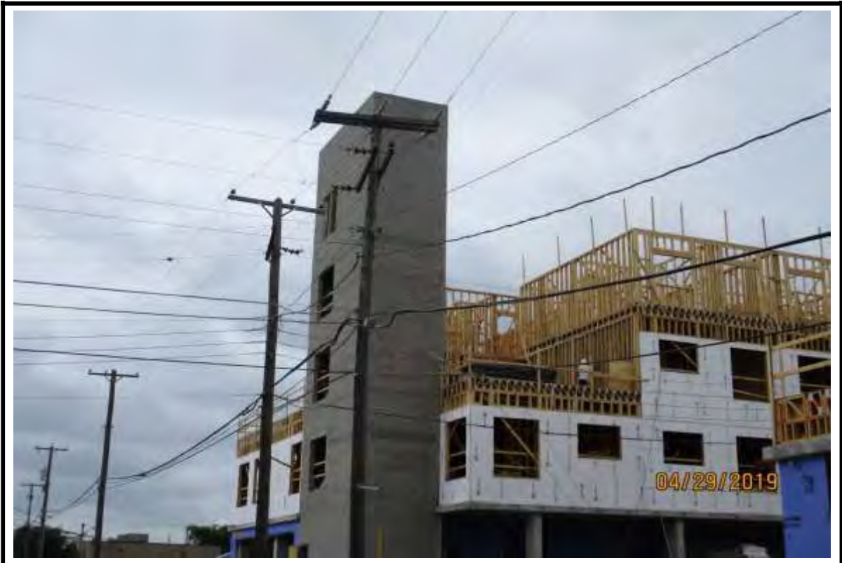
Photograph 1: CMU stair tower with wood framing on podium at Building “A”.
