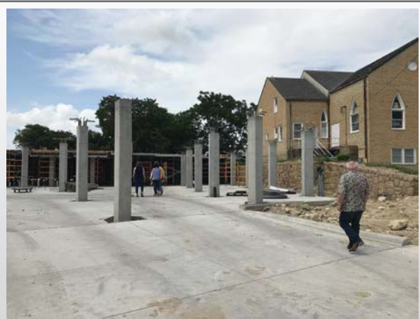
Building A columns
