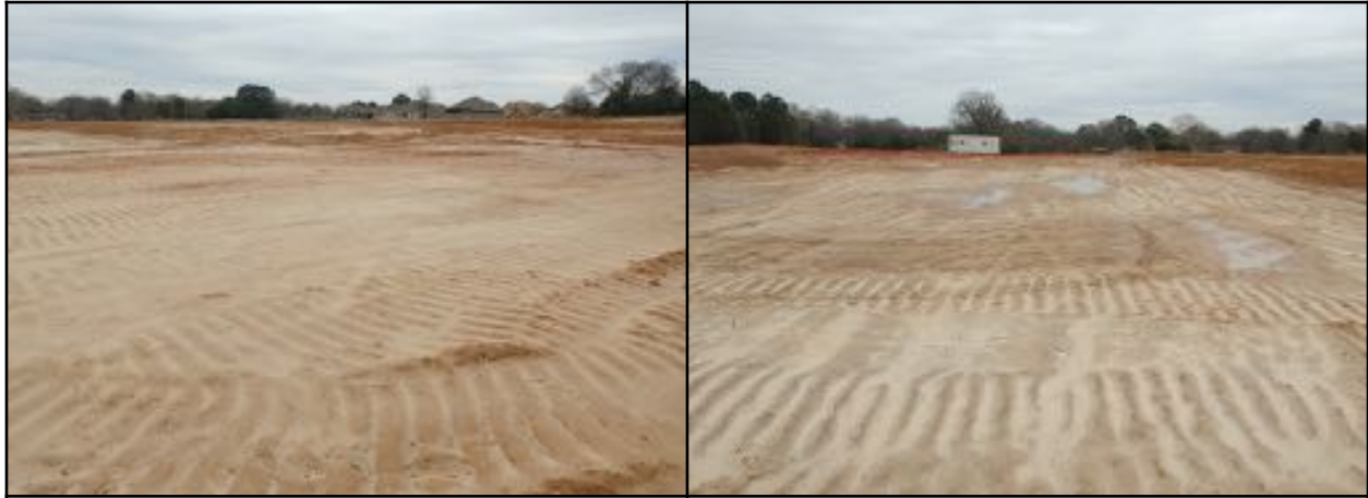
Photo # 7 View of building 2 pad
