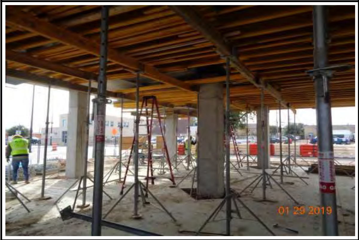
Photograph 7: Demolition of Building “A” Podium Deck forms.
