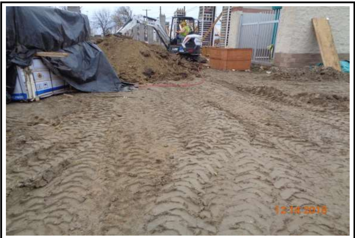
Photograph 2: Wet excavation between Buildings "A" and "B".
