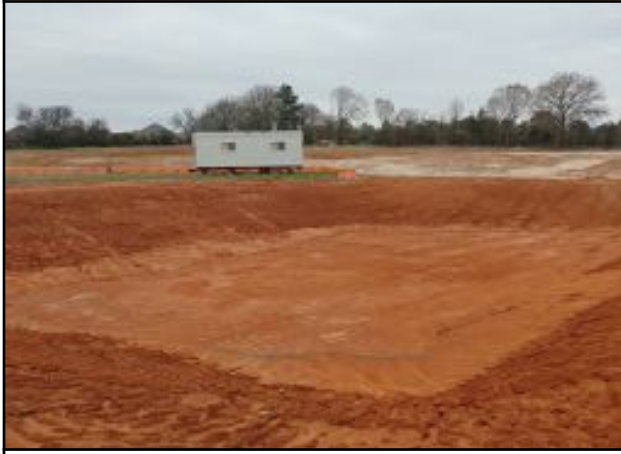
Photo # 5 Site Overview and Detention Pond
