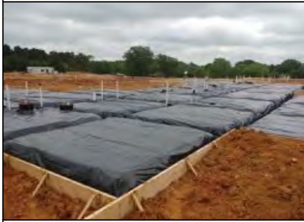
Photo # 17 Building pad 6 - Footings excavated
