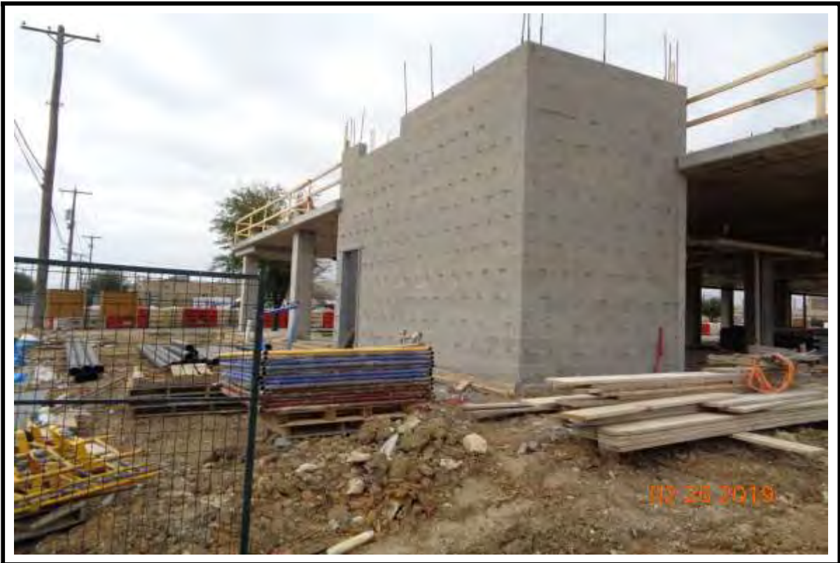
Photograph 6: Start of East masonry stairwell at Building “A”.
