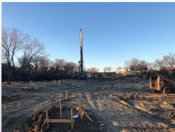
Building A Drilling piers in progress
