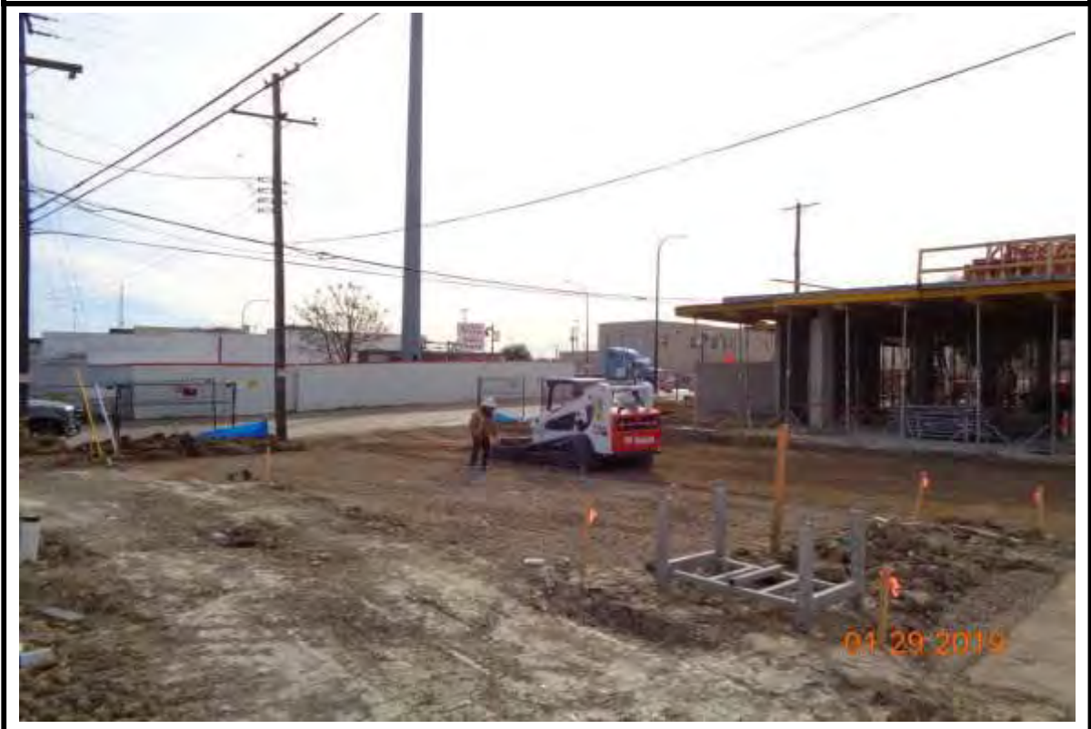
Photograph 5: Grading for continuation of paving between Buildings "A" and "B".
