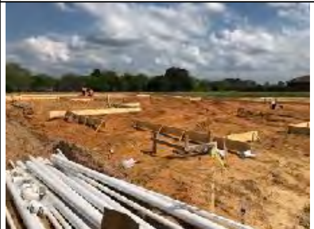
Photo # 16 Forming of slab in progress at Building #7
