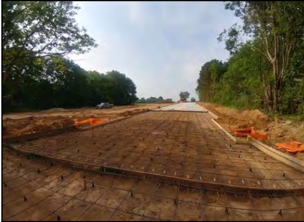
Photo # 1 Rebar and expansion joint rods in-place
