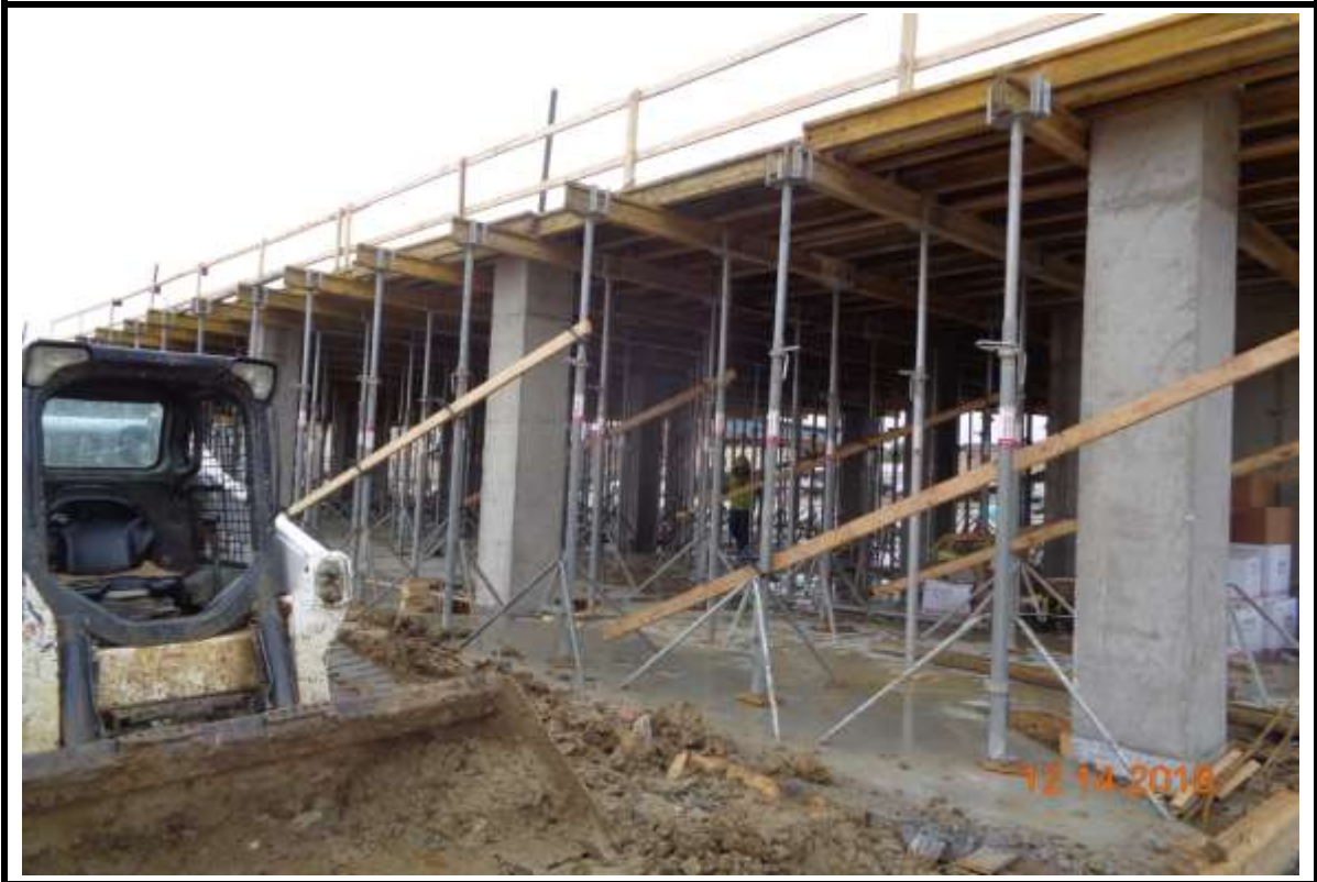
Photograph 5: Podium Deck forming at Building "A".
