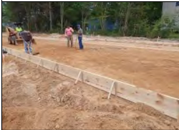
Photo # 5 Forms placed for futures driveway pours
