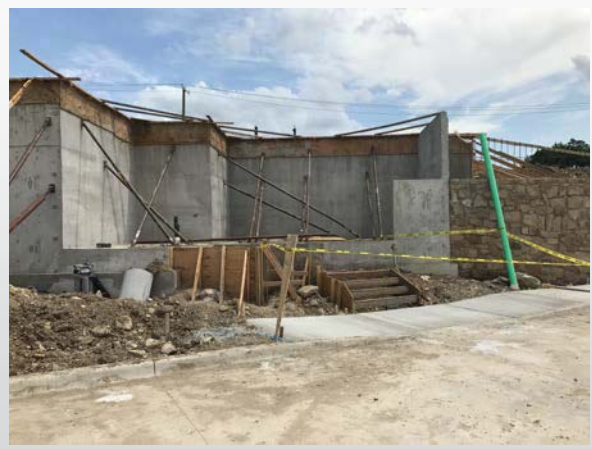
Stair tower foundation
