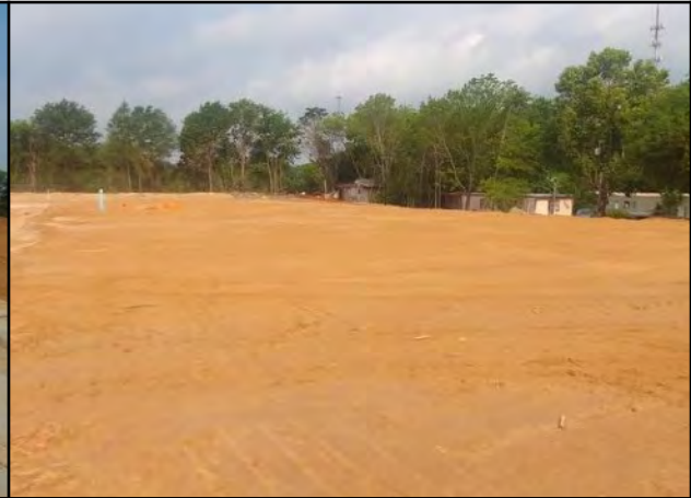
Photo # 8 View of building pad 1 - Pad established
