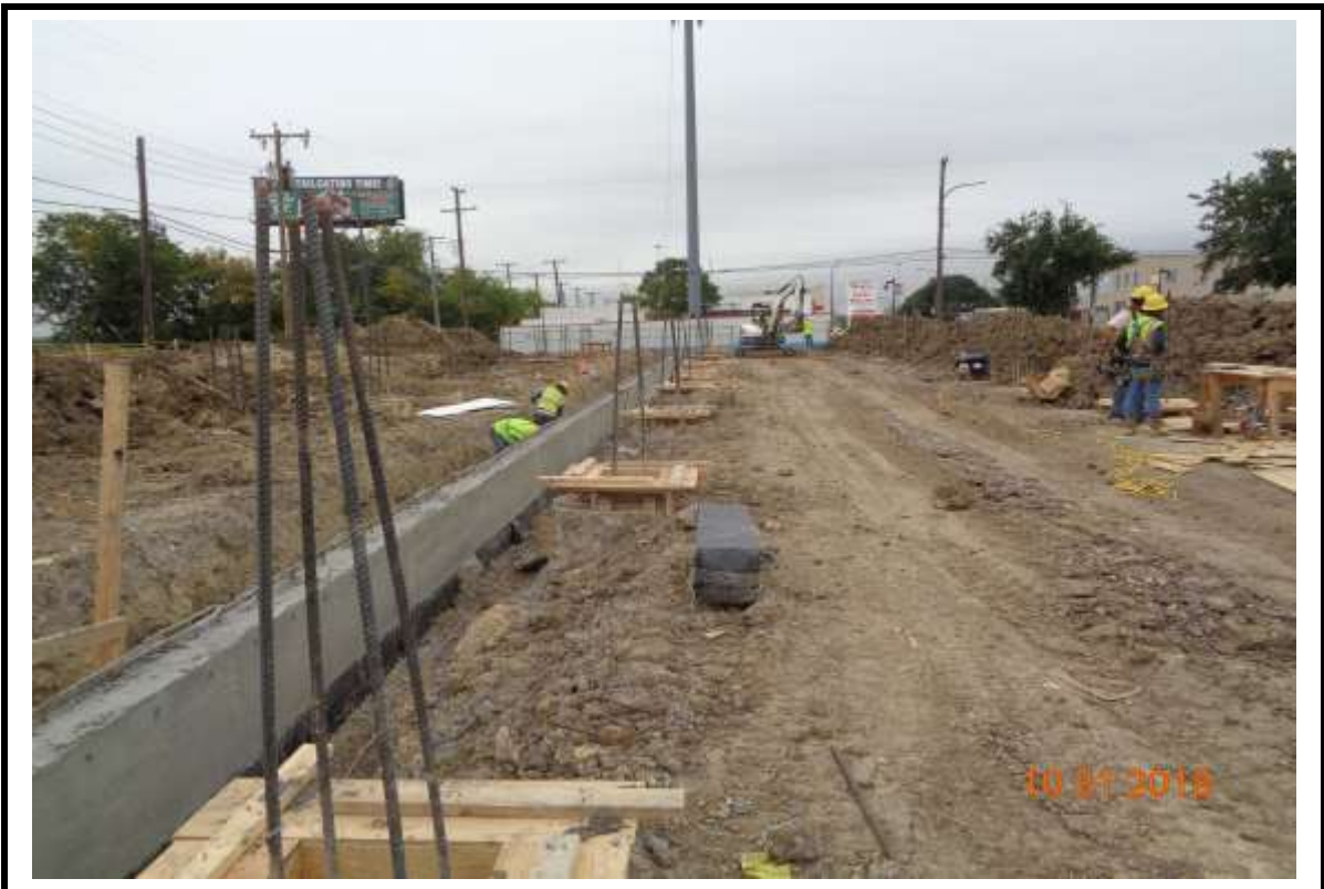
Photograph 6: Podium column line ready for vertical reinforcing.
