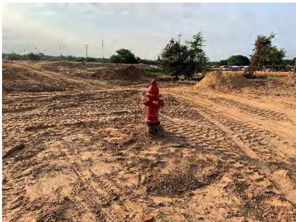
Photo 3: Fire hydrant installation at interior of site.
