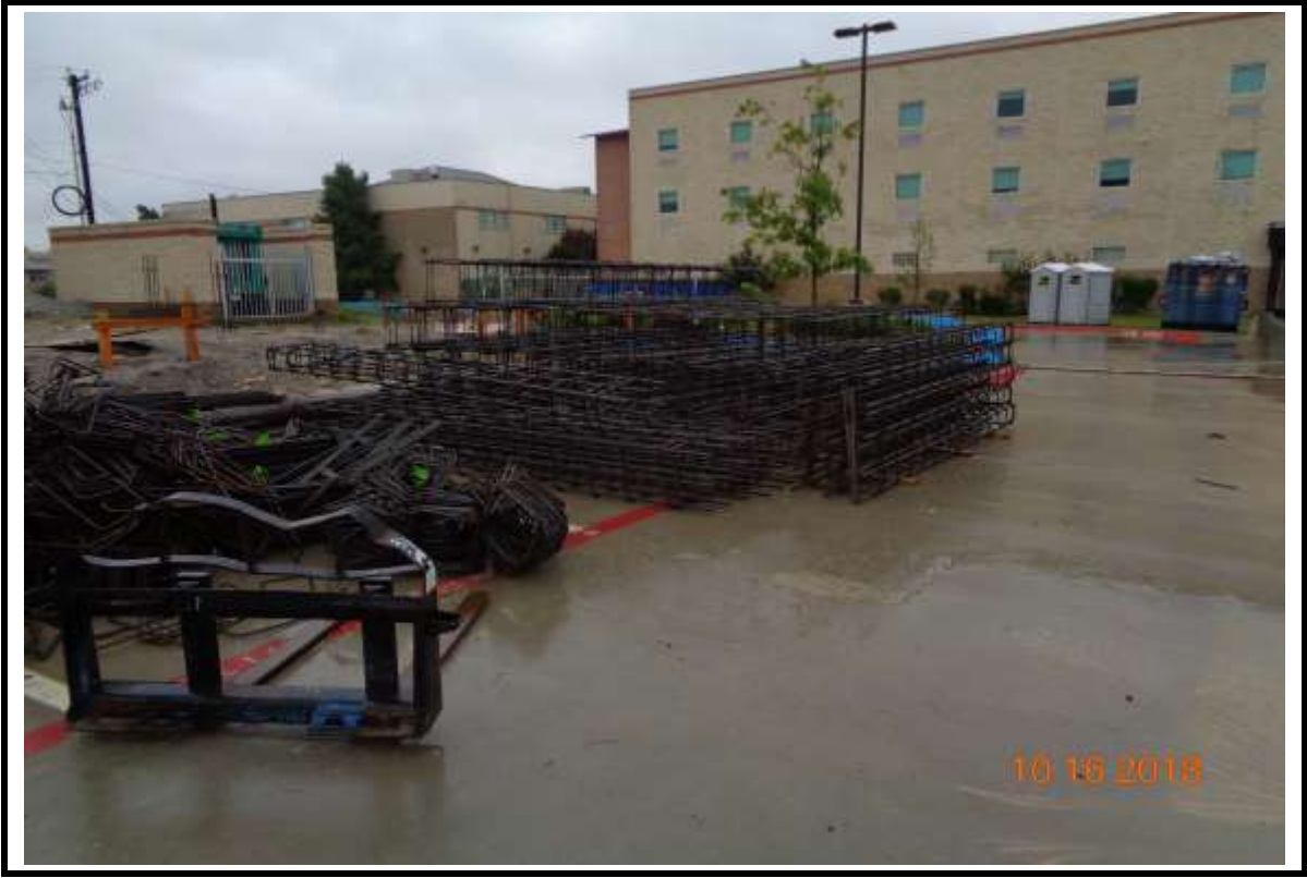
Photograph 2: Podium column reinforcing cages.
