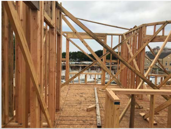
Second floor framing – Building B
