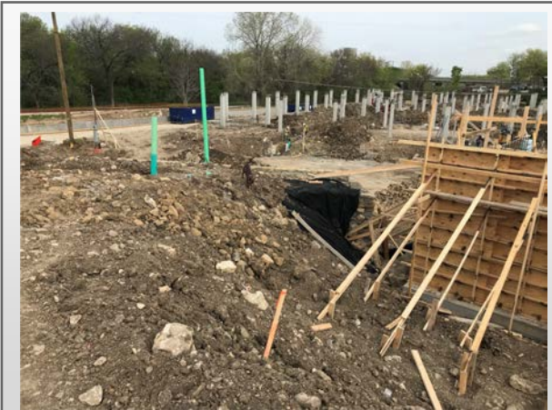
Foundation for Building B
