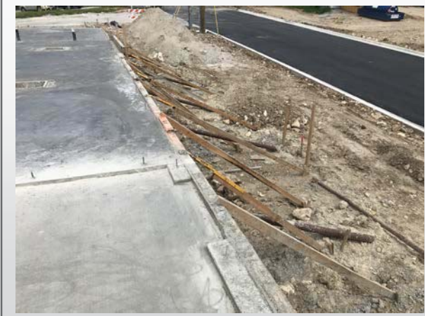
Building B Foundation along Mistletoe
