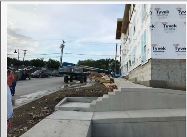
Concrete Handicap Ramp
