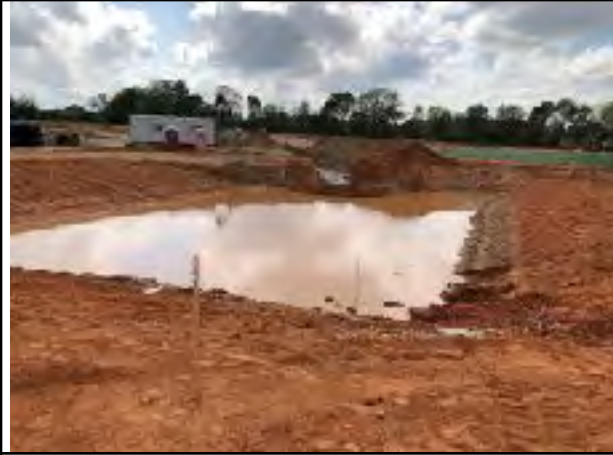
Photo # 7 View of completed pond excavation
