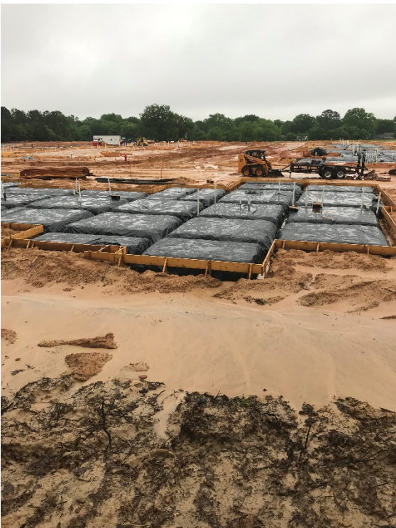
IMG 91 –Rain soaked and washed away dirt around form boards....all has to be replaced when dried out.
