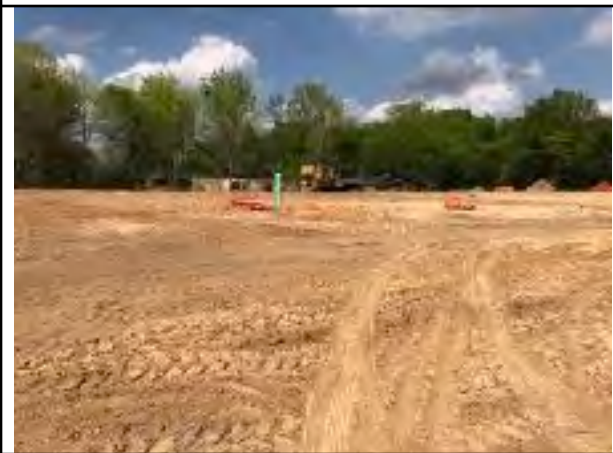
Photo # 11 View of established building pad 3
