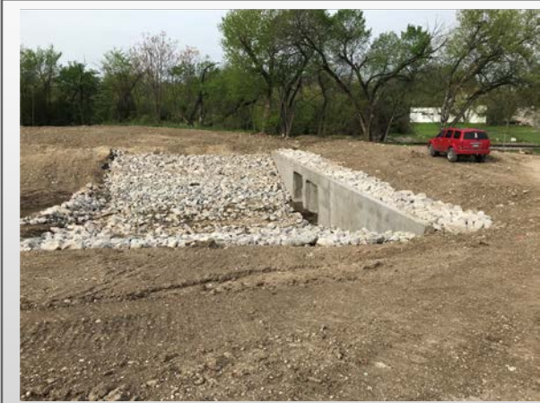
Headwall Construction
