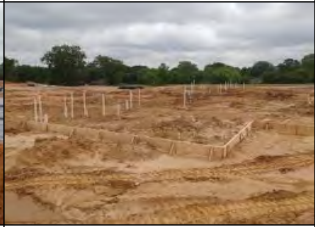
Photo # 18 Building pad 7 - Form boards set and underground plumbing complete
