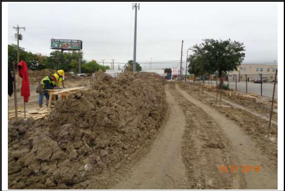
Photograph 9: Beam spoils to be moved to haul-off area.
