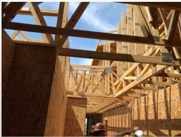
Building B Interior Framing
