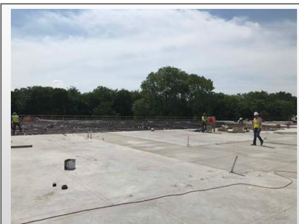
Building A Podium
