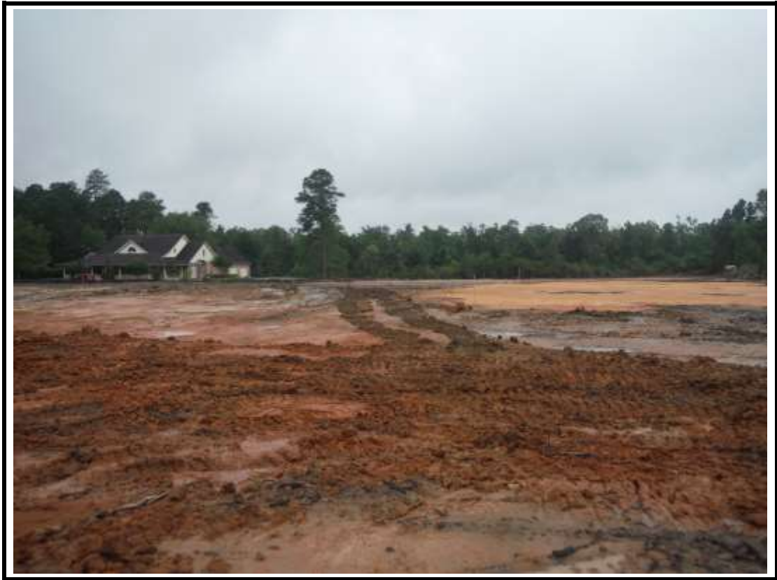
Photograph 5: Site work towards rear of property.
