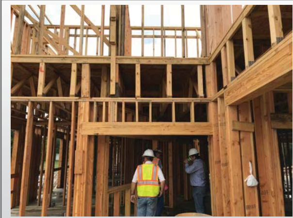
Clubhouse Framing at entry – Building B
