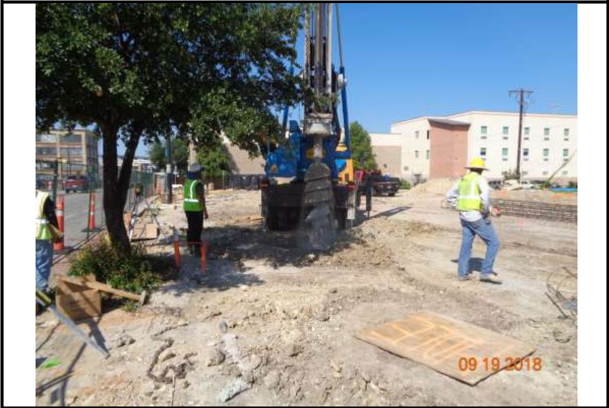
Photograph 5: Removing soil spoils from the drilled shaft.
