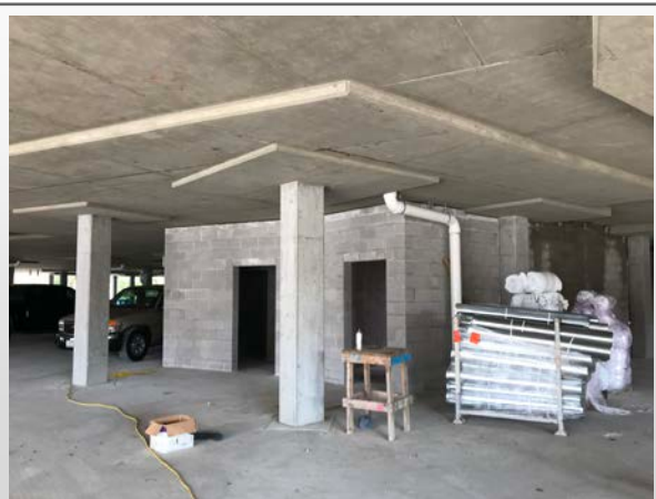
Parking level under podium at Building A
