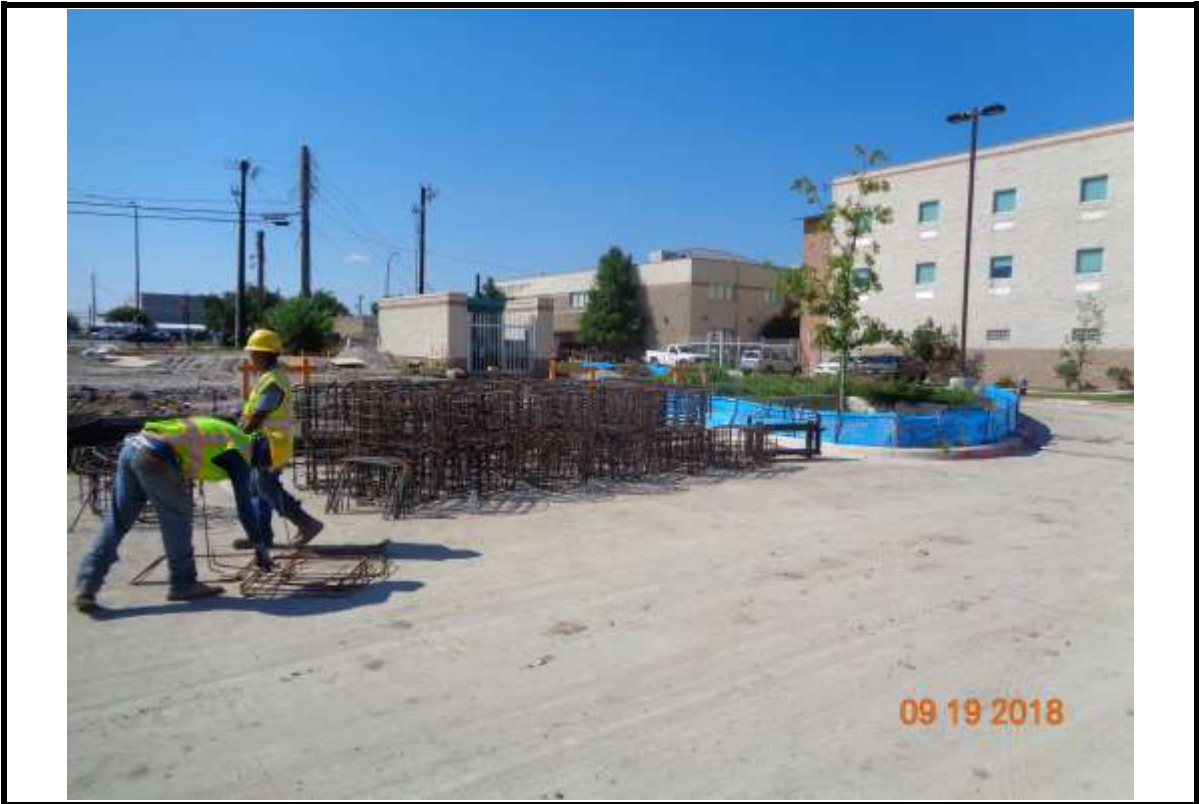
Photograph 1: Tying pier cap reinforcing.
