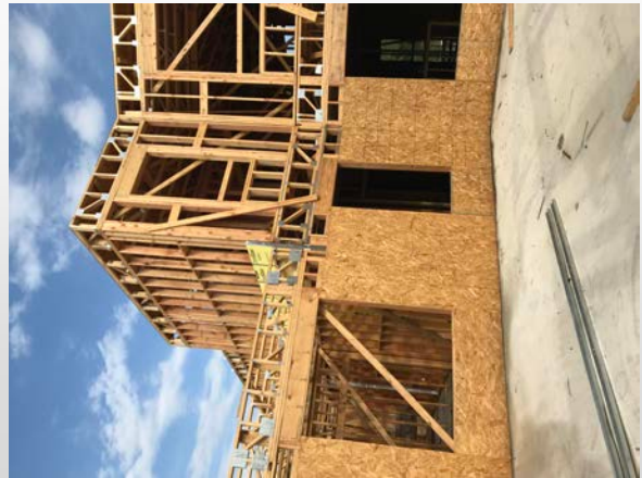
Unit framing above podium at Building A
