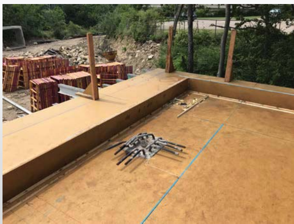
Building A Podium Forming
