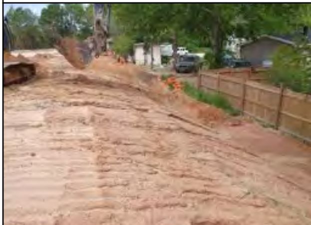
Photo # 11 North end of building pad 1 shaping for water run-off in-progress
