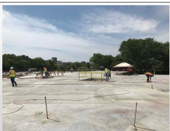
Building A Podium
