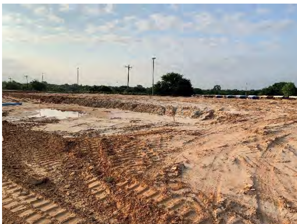
Photo 5: Pad preparation at Building 2.
