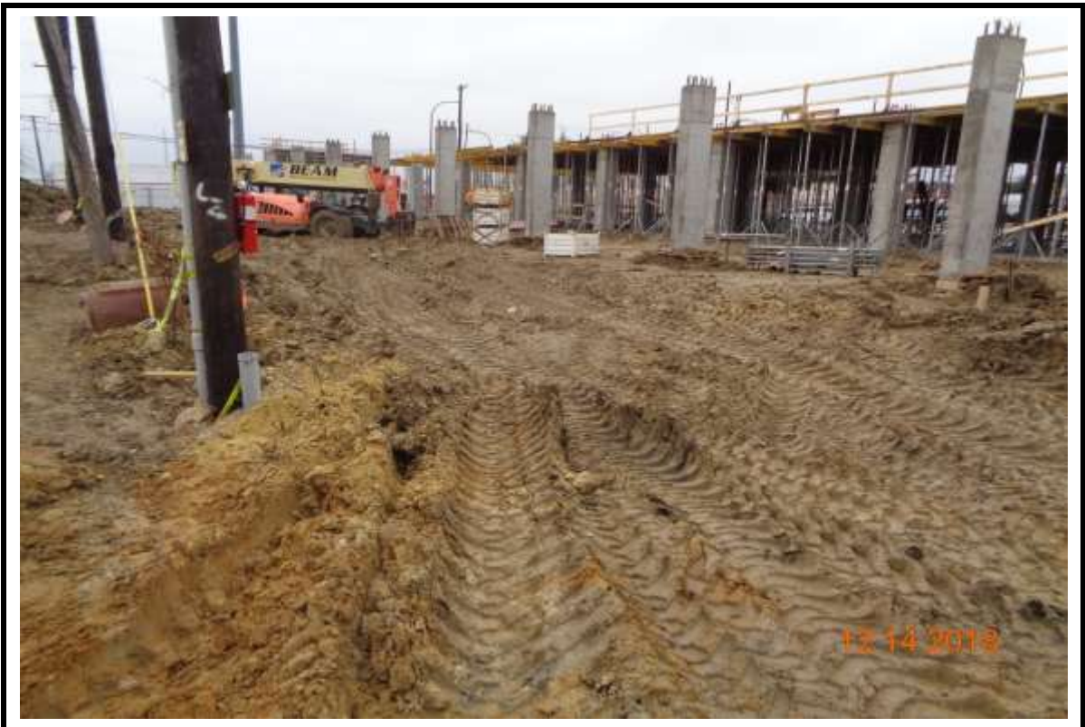
Photograph 4: Balance of columns at Building "A".
