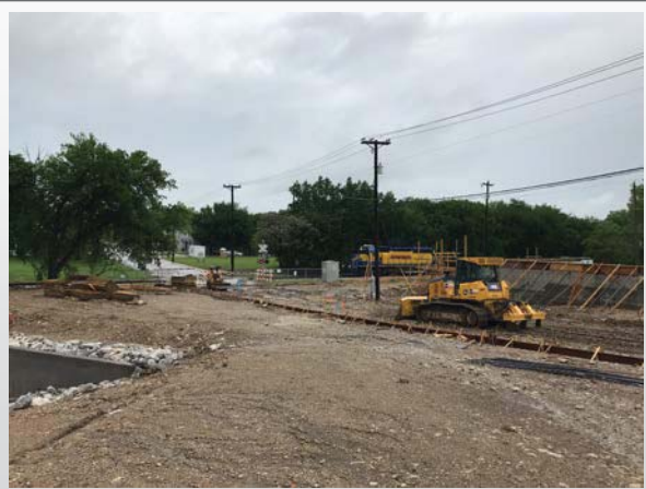
Mistletoe and the west corner of Building B
