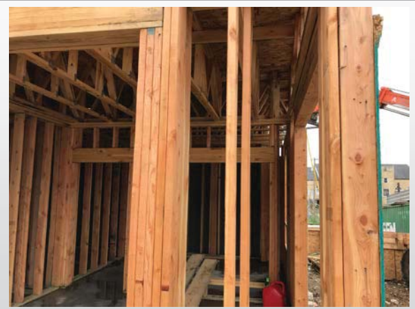
First floor framing – Building B
