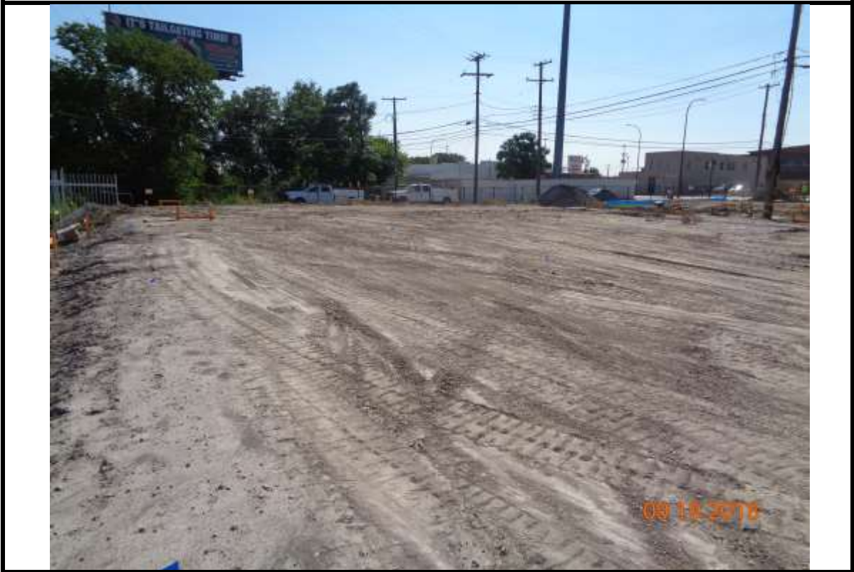
Photograph 3: Pad "B" ready for piers.
