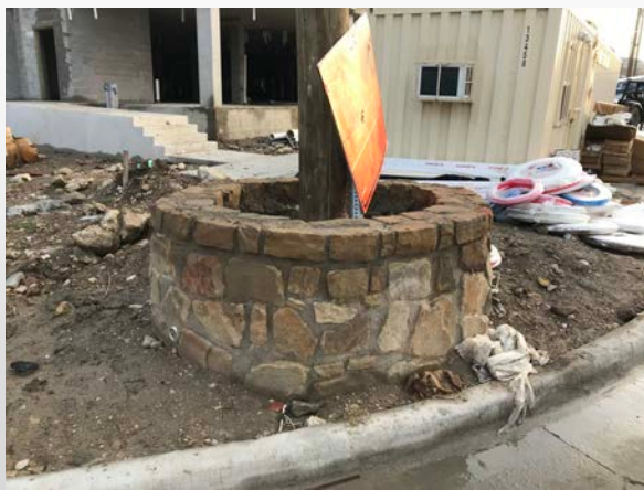
Retaining Wall at Existing Telephone Pole
