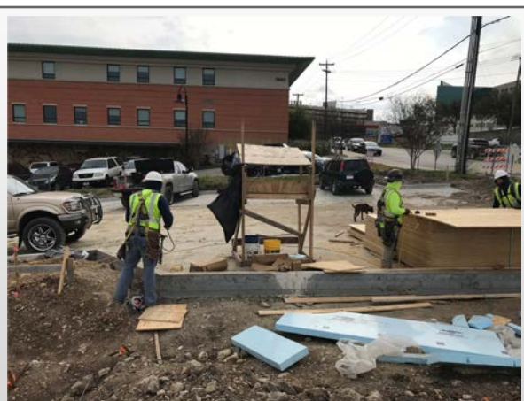
Foundation for Building B
