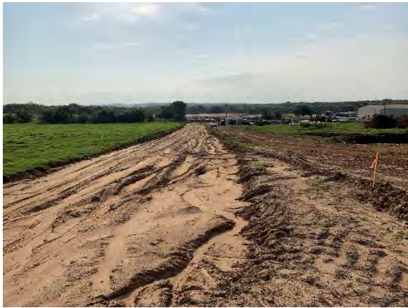
Photo 1: Progress at main entry drive off Buchanan Road.
