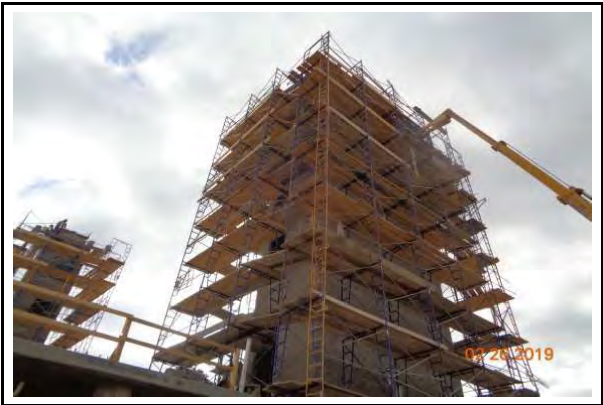
Photograph 1: CMU stair well top-out at Building "A".
