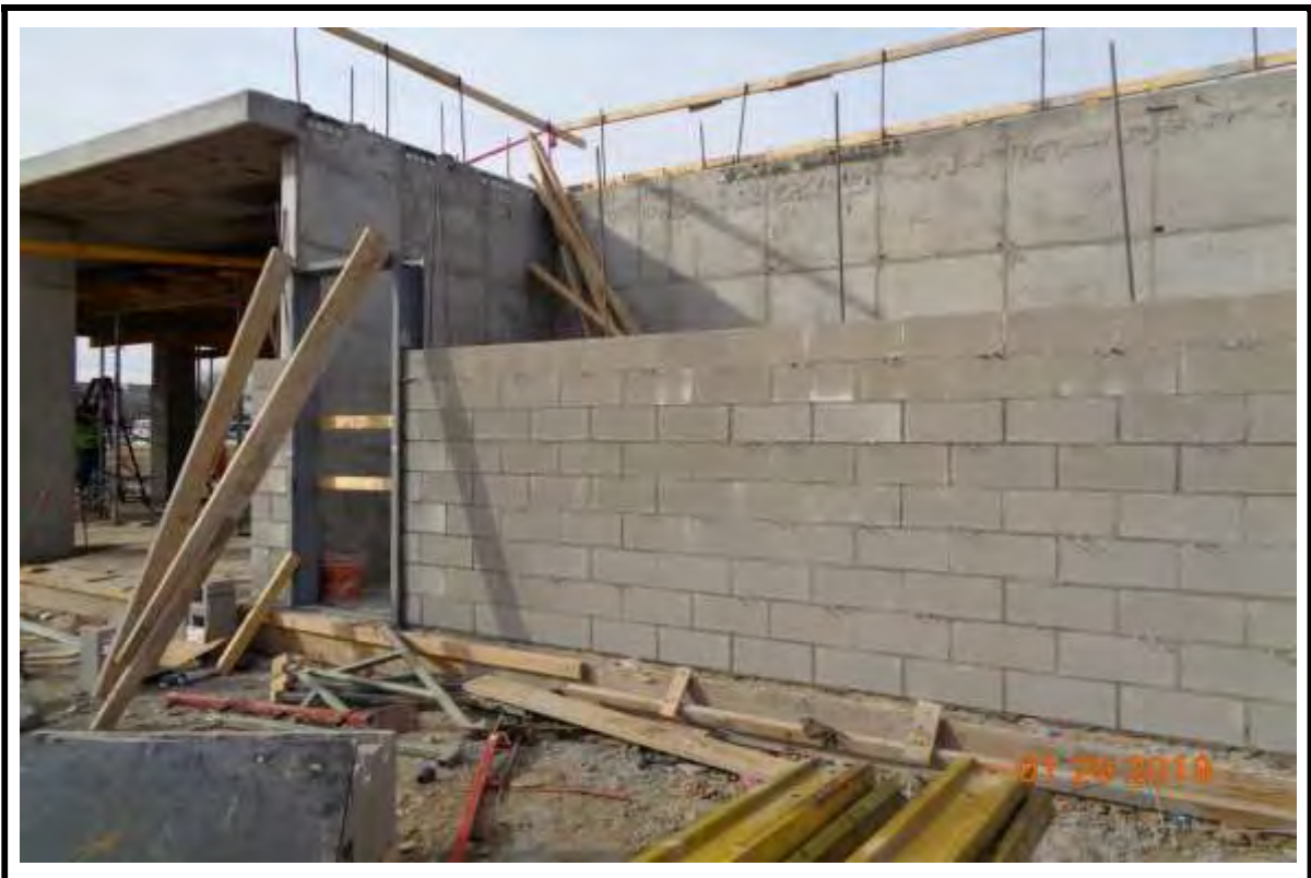
Photograph 6: Start of Masonry stairwells at Building "A".
