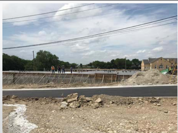
Repaired Mistletoe and Building B Foundation
