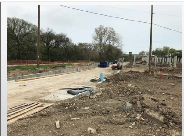
Concrete Fire lane
