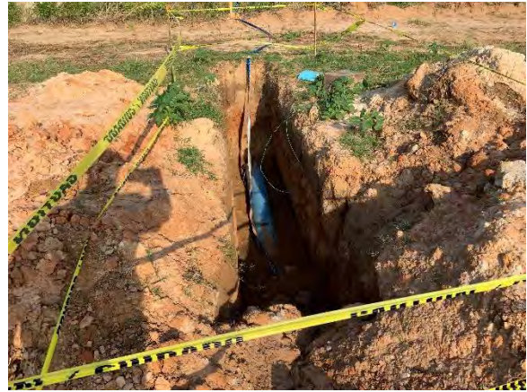
Photo 2: Water main installation at north side of site.
