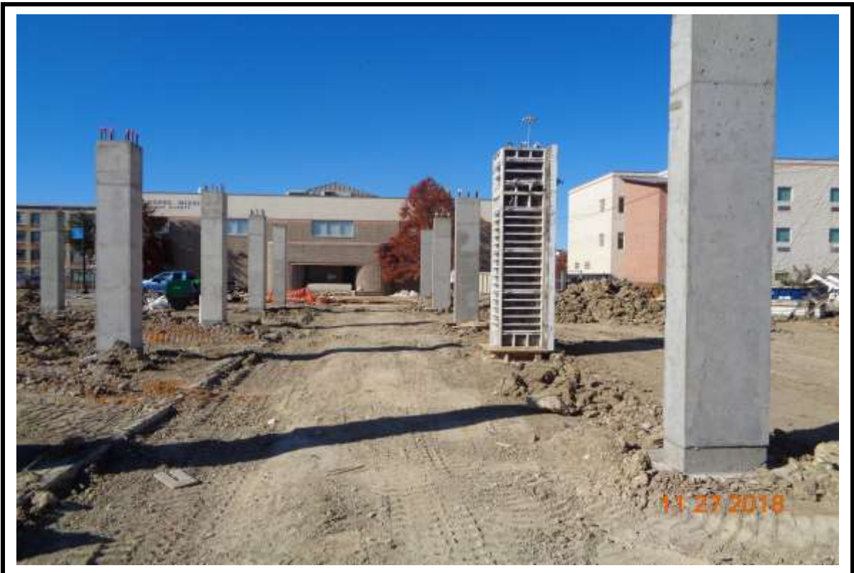
Photograph 10: Podium columns at Building "B".
