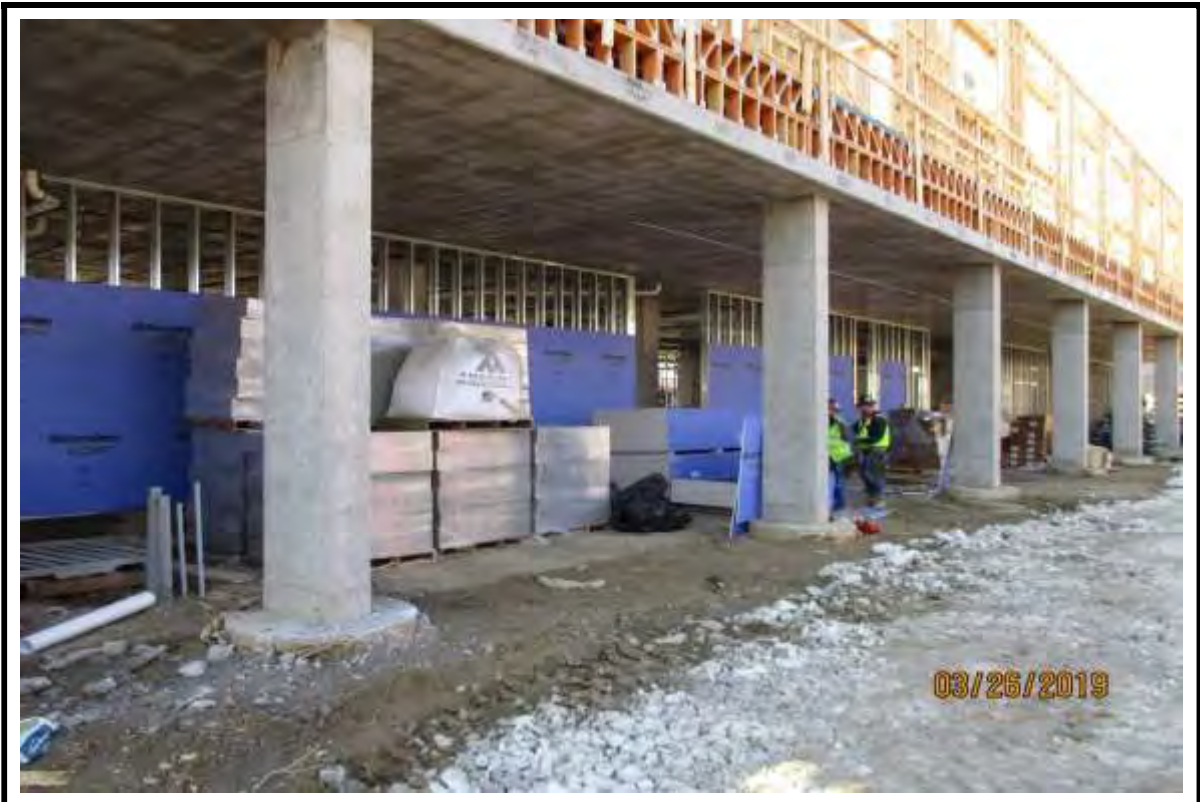
Photograph 10: Sheathing staged for installation, Metal wall framing beyond.
