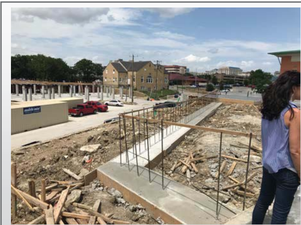
Foundation for Sound wall
