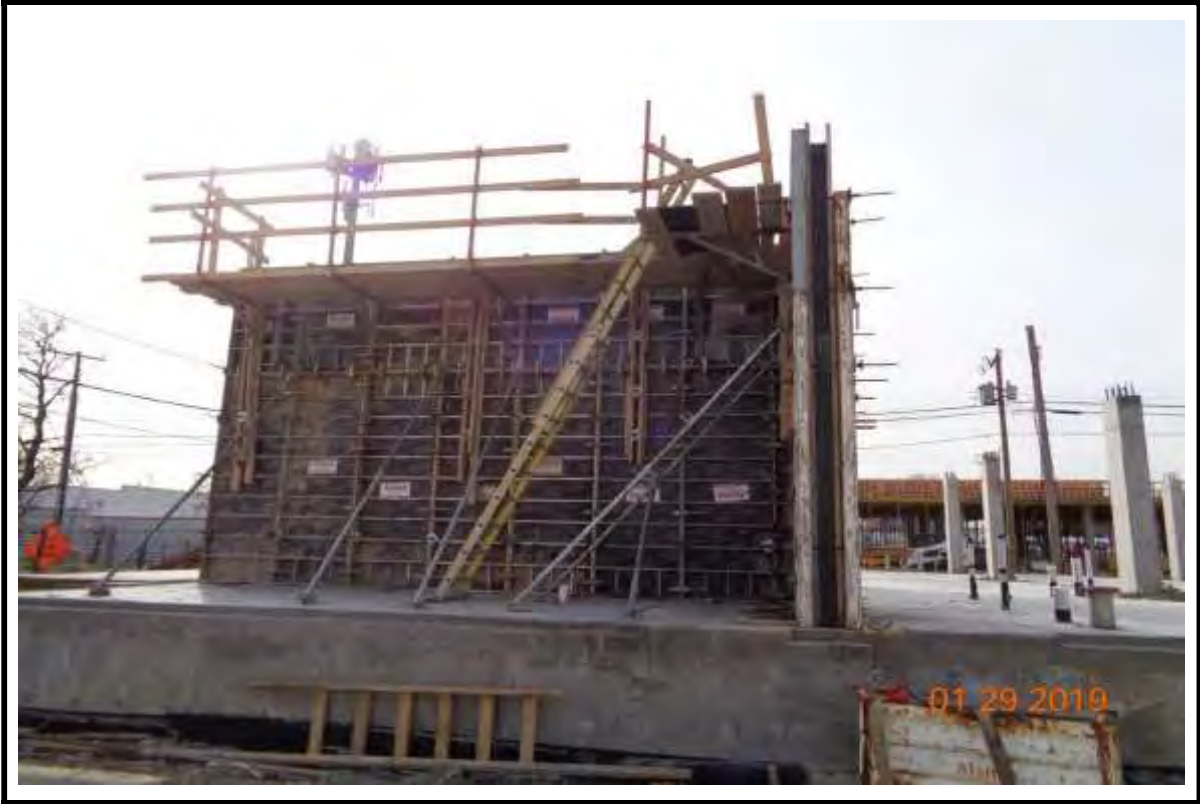
Photograph 10: Completed Stairwell wall at Building "B" East end.
