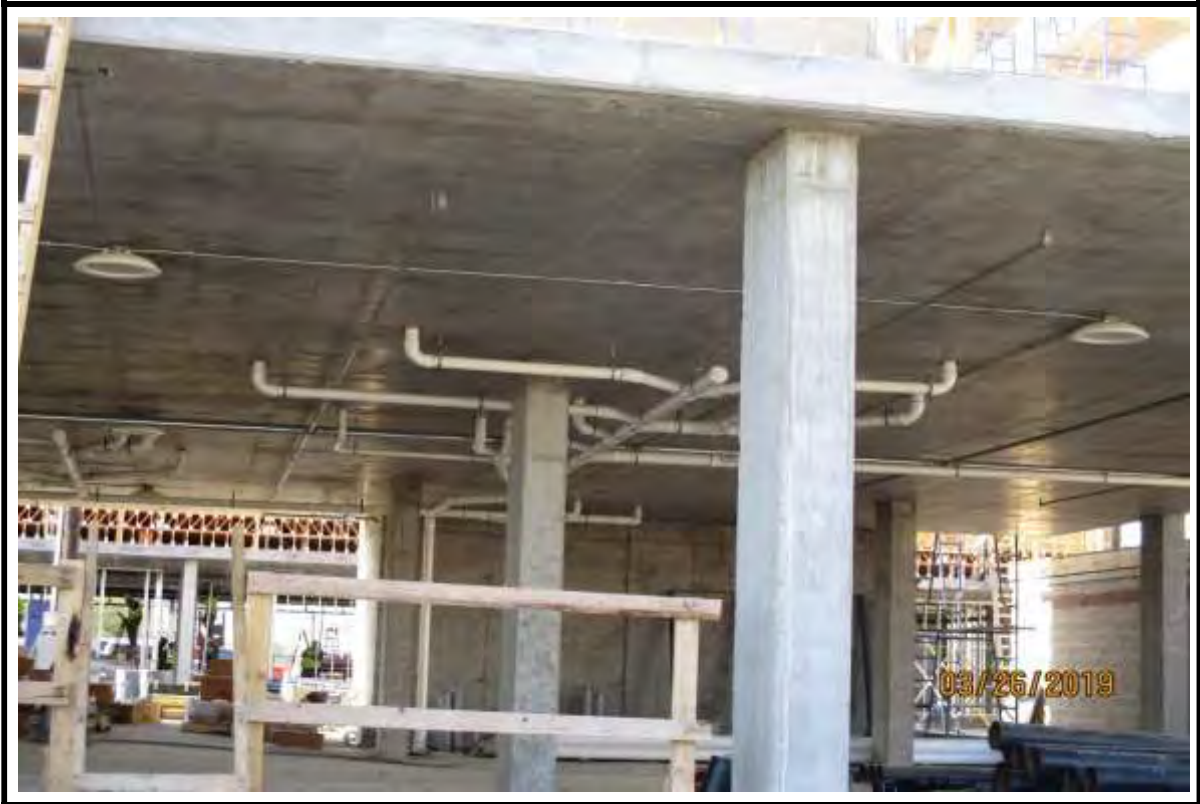
Photograph 9: Utilities Rough-in at Building "B".
