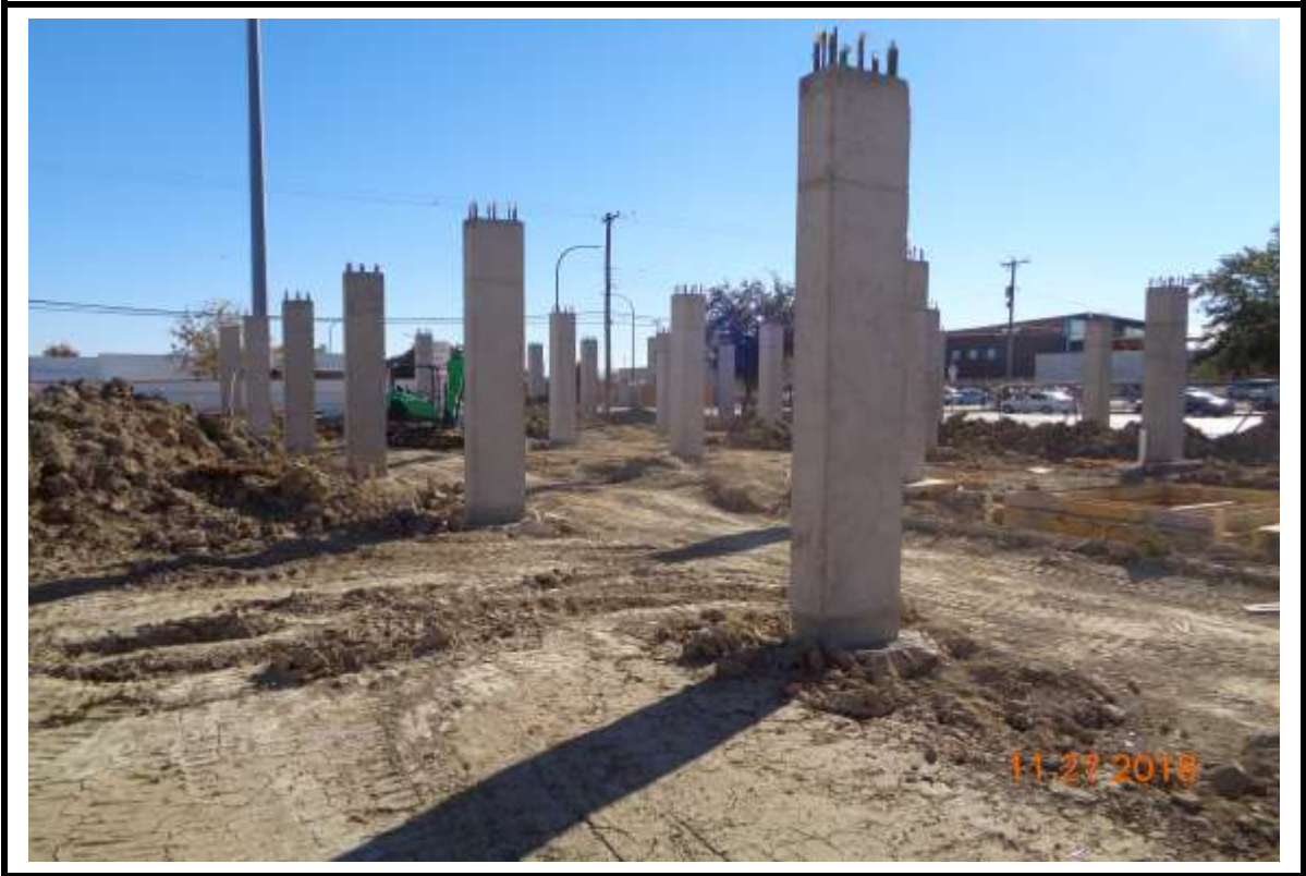
Photograph 7: Podium columns at Building "A".
