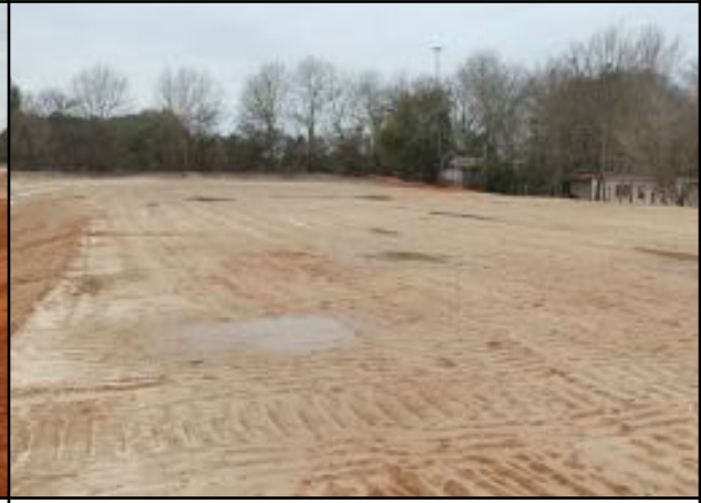
Photo # 6 View of clubhouse and building 1 pad
