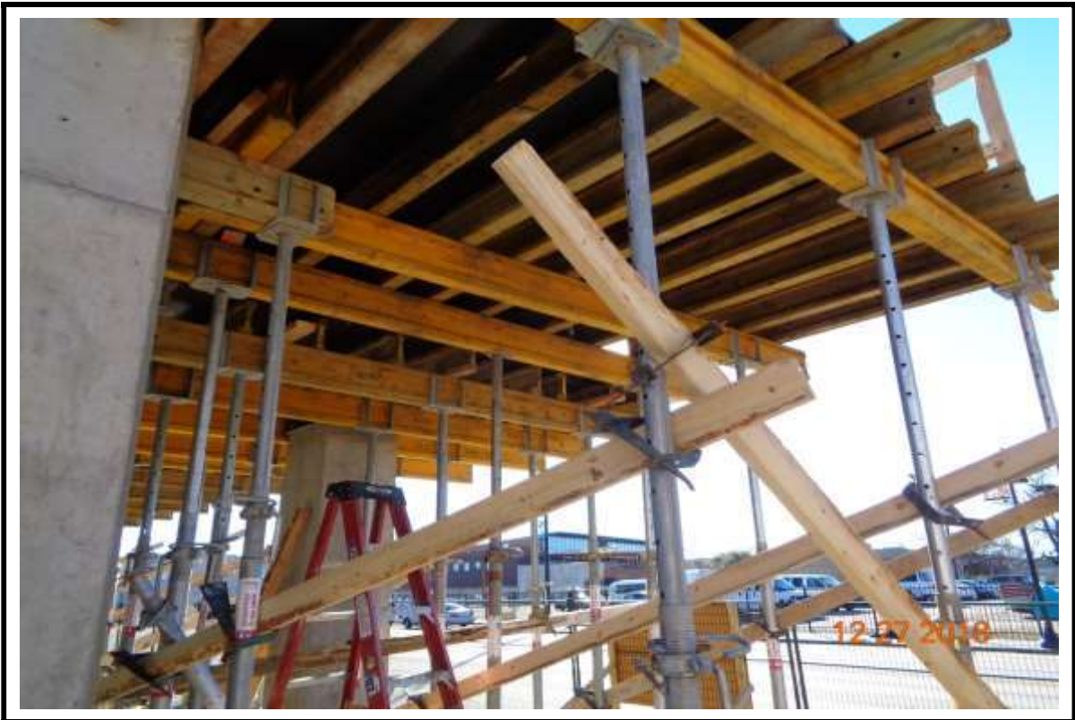
Photograph 6: Timber beam for support at Building "A" Podium Deck.
