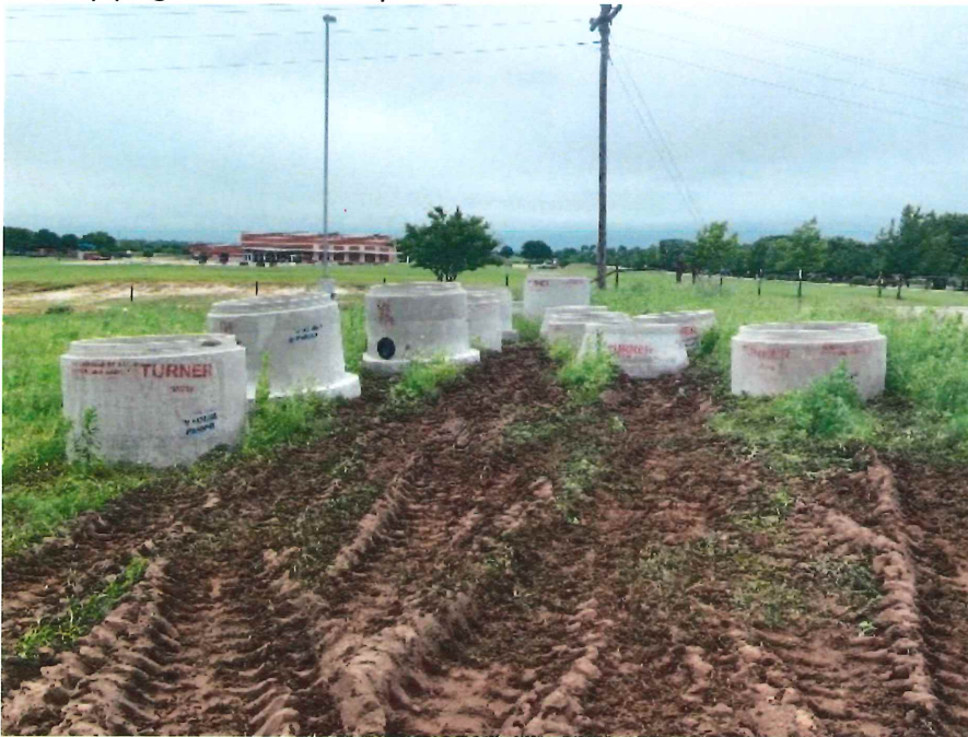
Sewer piping on-site and ready for installation.
