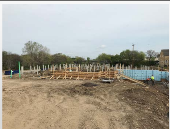
Foundation for Building B
