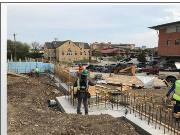
Foundation for Building B
