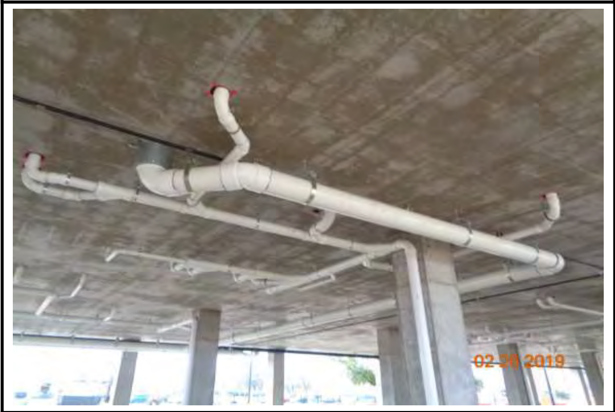
Photograph 3: Under podium sanitary and storm piping at Building "A".
