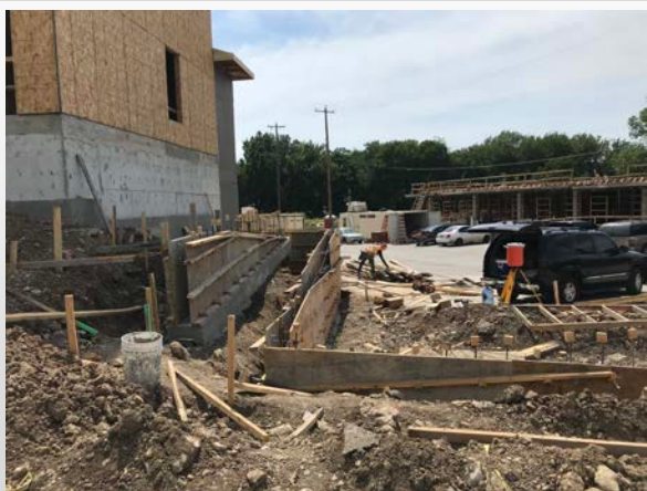
Building B HC ramp
