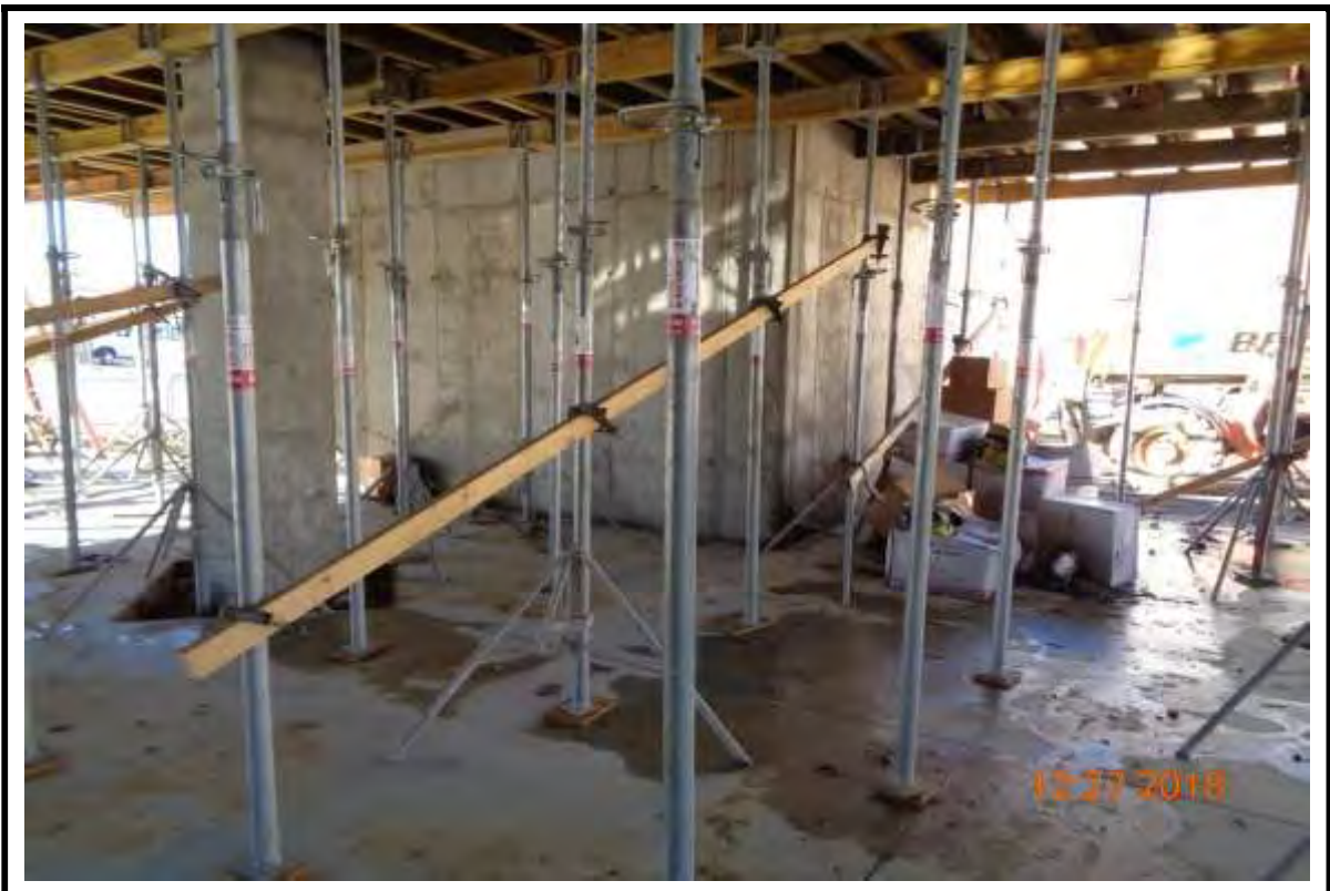
Photograph 4: Cast in place walls at Building "A".
