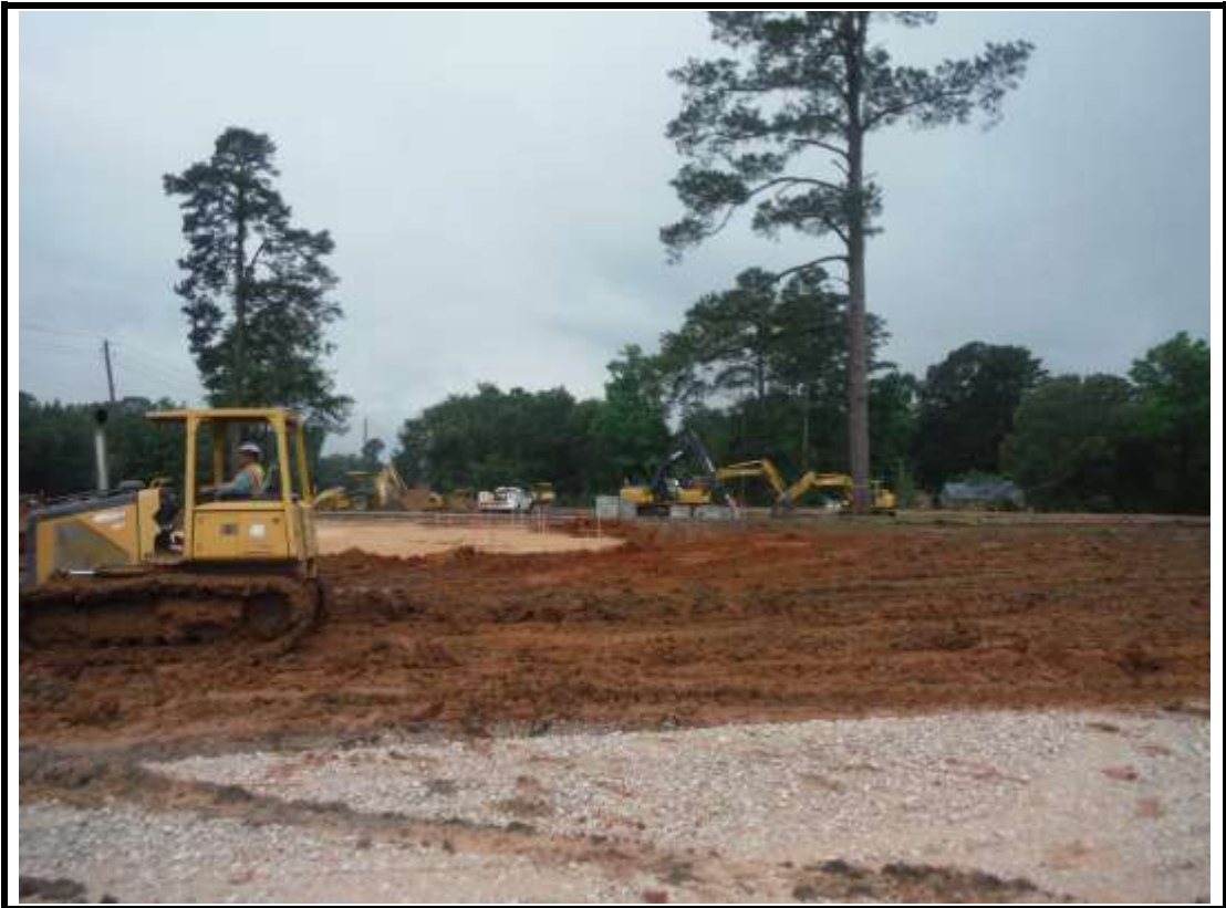
Photograph 2: Site & pad work on Clubhouse.
