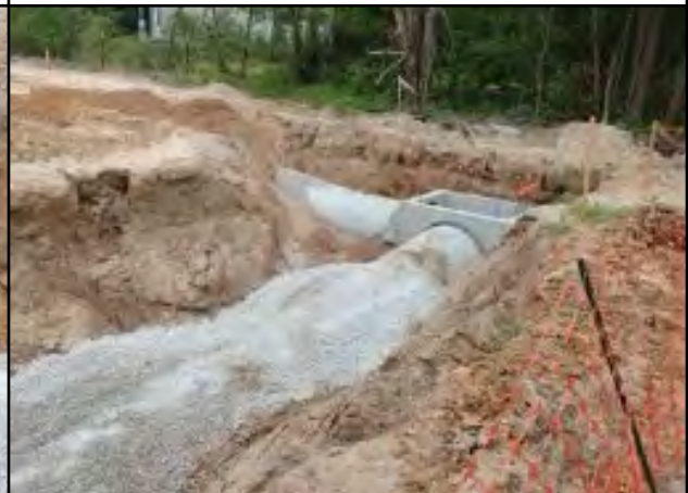
Photo # 4 Backfill of storm utilities underway
