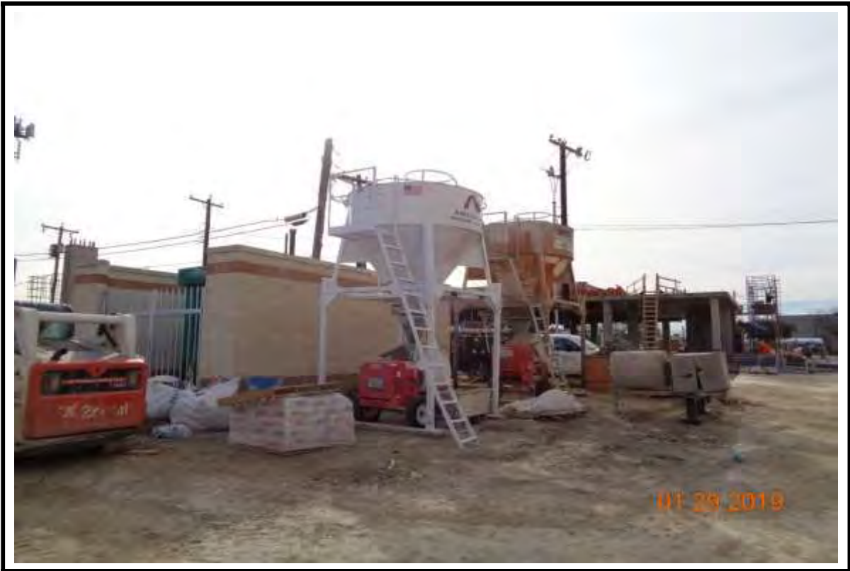
Photograph 2: Onsite batch plant to control Masonry strength and color.
