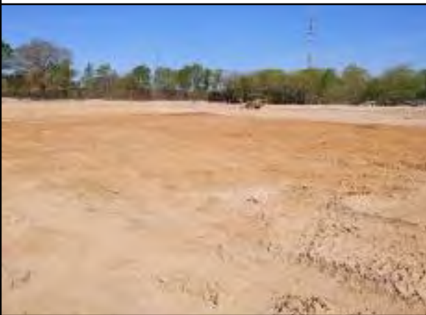
Photo # 17 View of established building pad 8
