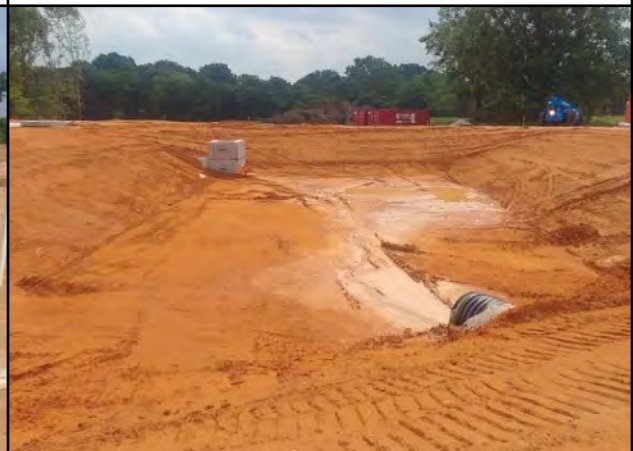
Photo # 18 Detention pond established with storm drain lines connected
