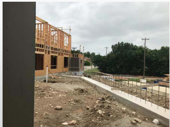
Courtyard Building B
