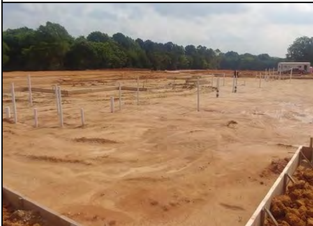
Photo # 11 Building 3 - Forms and under slab plumbing complete
