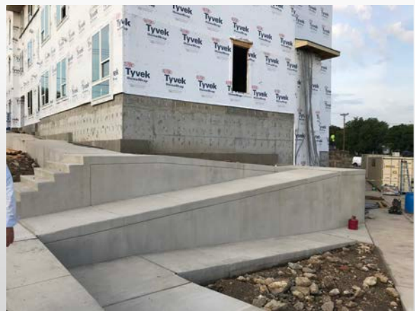
Concrete Handicap Ramp
