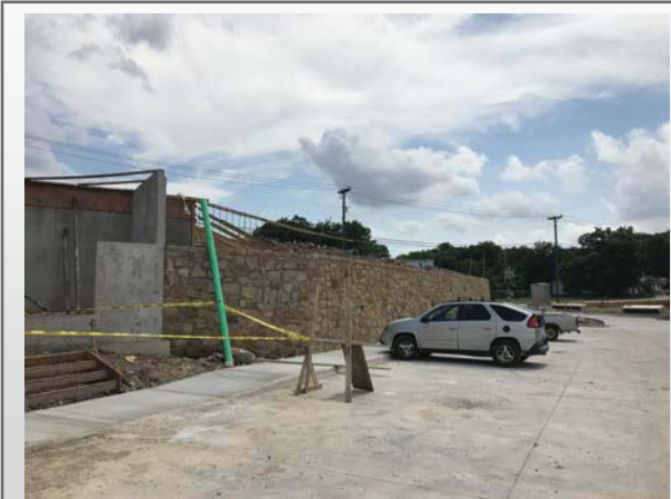
Gravity wall at Building B
