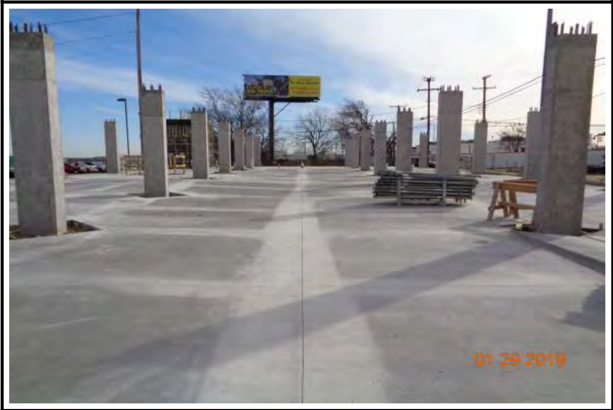
Photograph 3: Finished podium columns and paving at Building "B".
