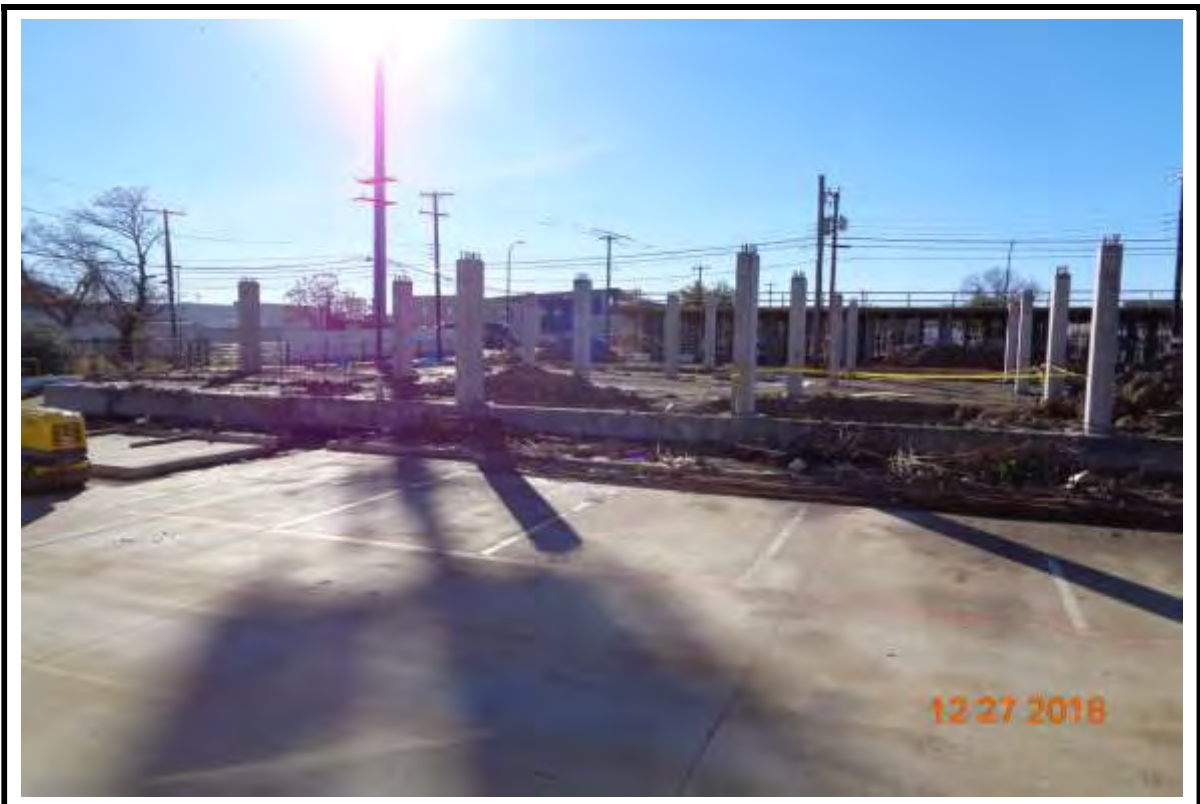
Photograph 10: Completed Podium columns at Building "B" East end.
