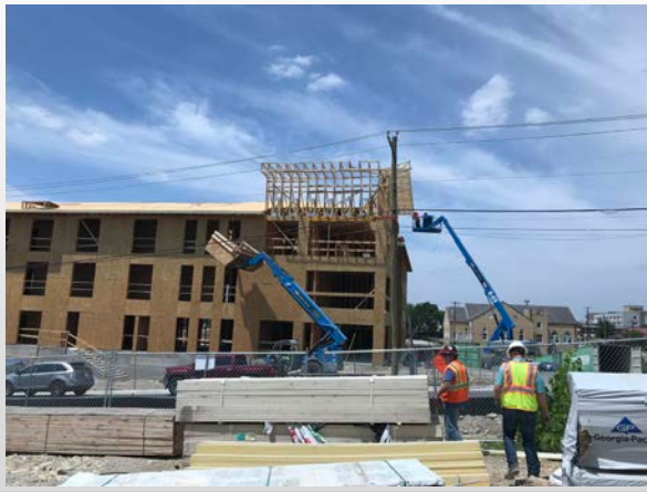
Building B Framing
