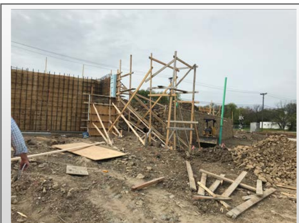
Foundation for Building B
