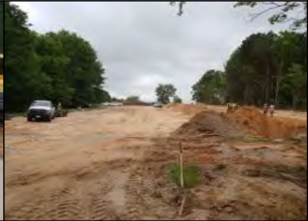
Photo # 2 Site entrance overview
