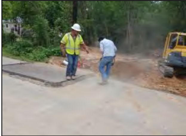
Photo # 1 Utility tie-ins in-progress
