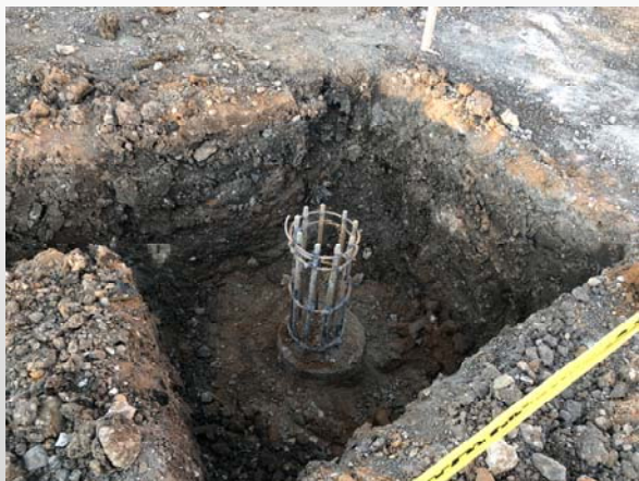
Building A Drilling pier completed at this location.
