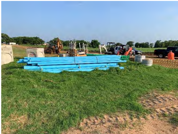
Photo 9: Stocked water piping.
