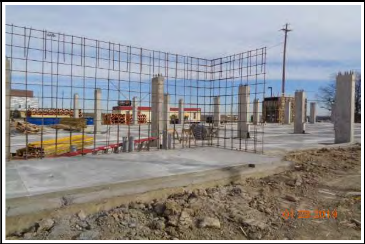
Photograph 9: Cast-in-place wall reinforcing at Building "B" West end.
