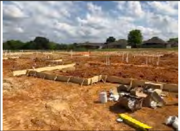
Photo # 14 Underslab plumbing complete at Building 6
