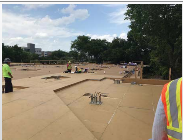
Building A Podium forming
