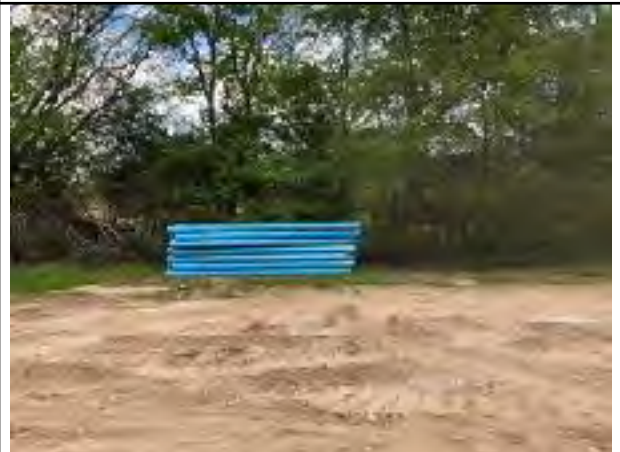
Photo # 22 PVC water pipe stored on site
