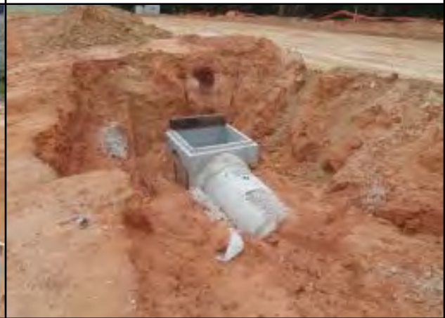
Photo # 6 Storm drain backfill expected soon
