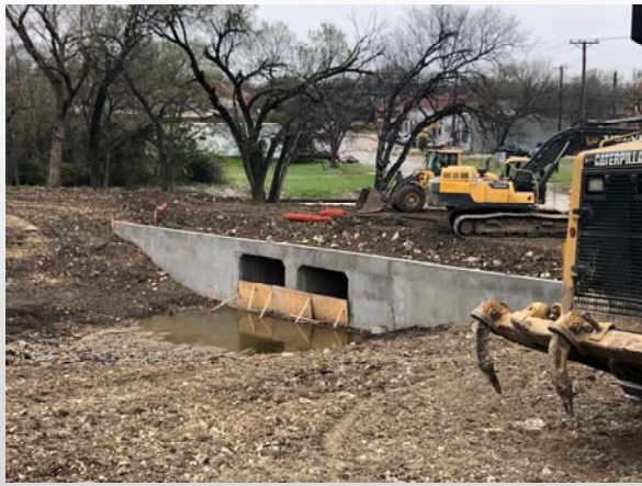
Offsite box culvert completed final grading underway
