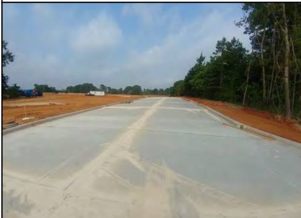
Photo # 5 View of concrete paving at Sunset Drive
