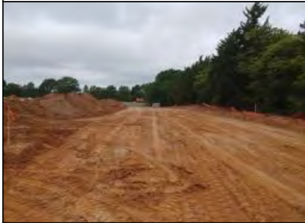
Photo # 9 Future Driveway Near detention pond - form placement to occur soon
