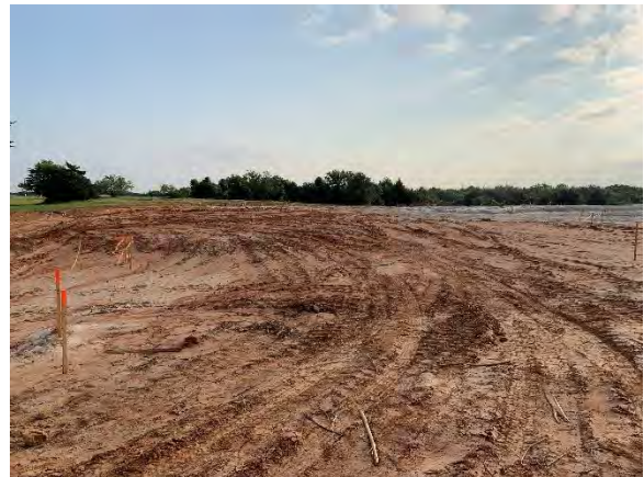
Photo 4: Rough grading progressing at interior paving areas.
