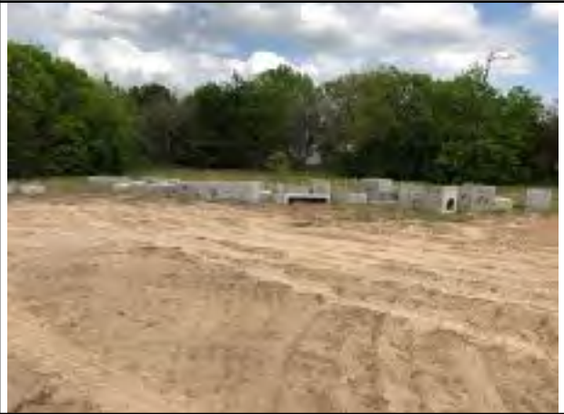
Photo # 20 Storm drainage manholes stored on site
