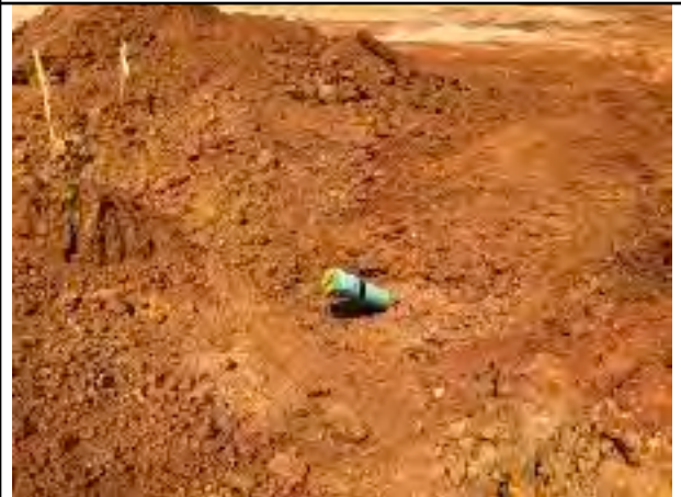
Photo # 4 Detail of sanitary sewer stubs near building 5
