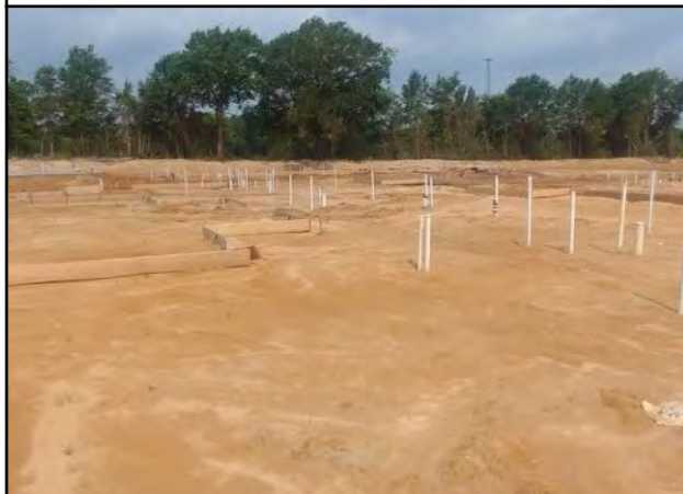
Photo # 17 Building 9 - Concrete forms and under slab plumbing complete
