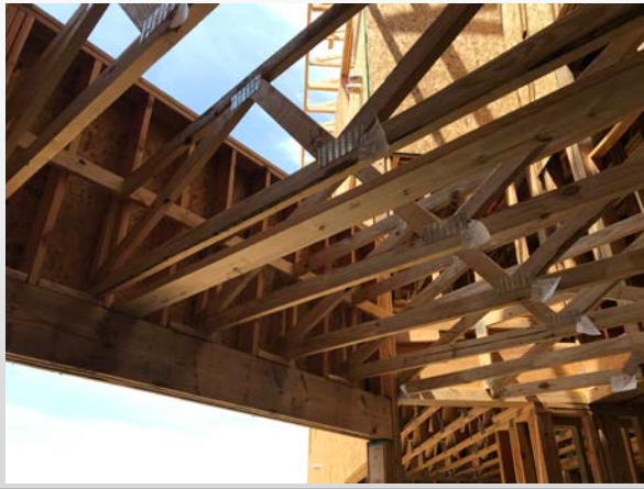
Building B Interior
