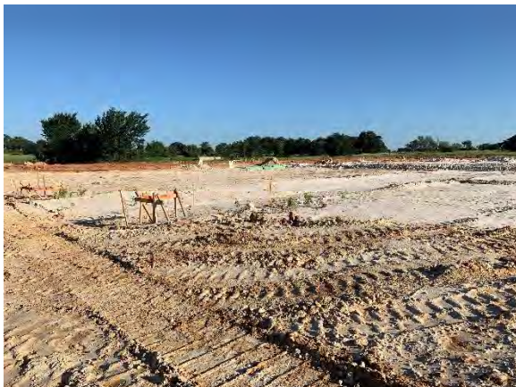
Photo 11: Completed batter board installation at Buildings 4 & 11.
