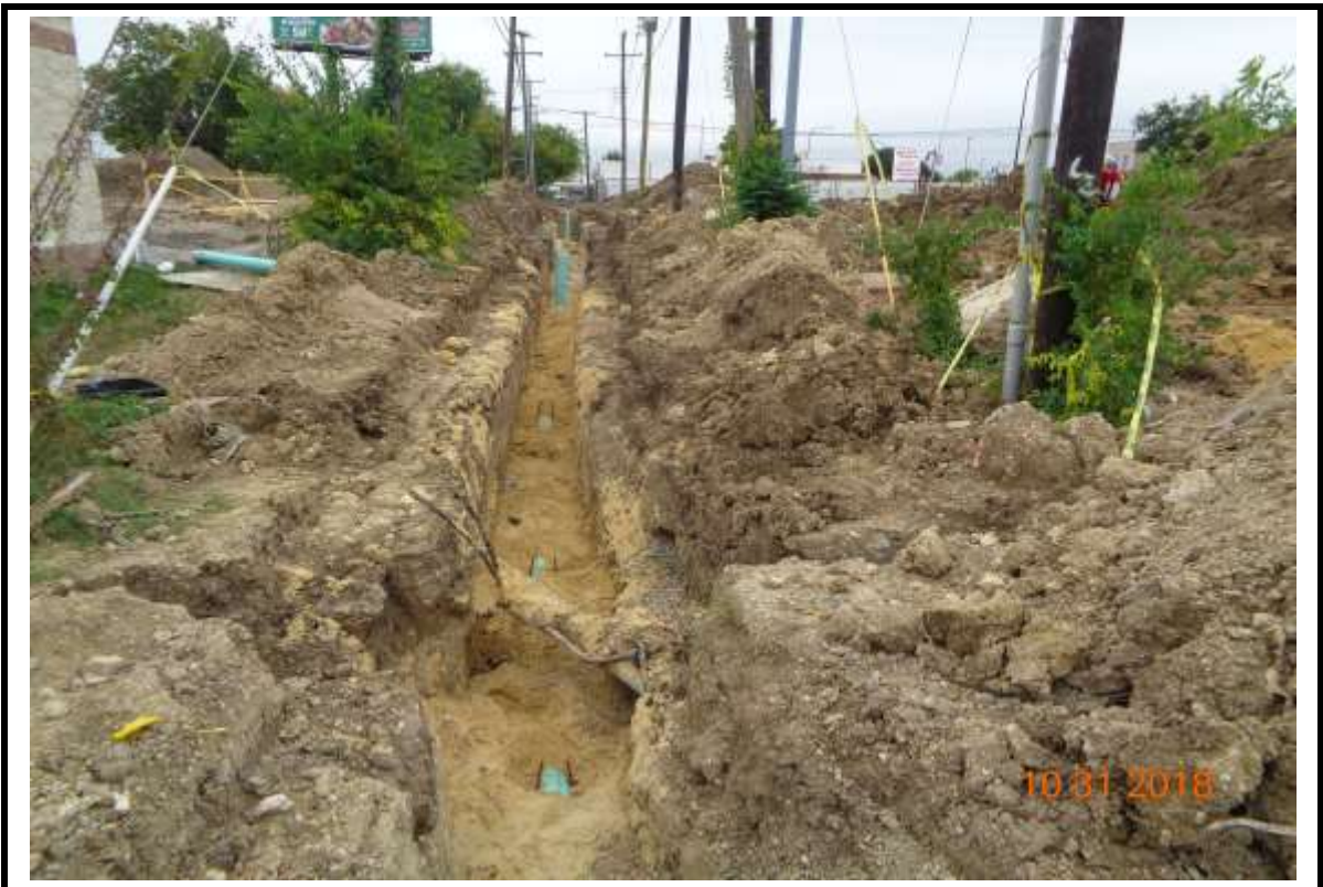
Photograph 4: Sanitary line at driveway.
