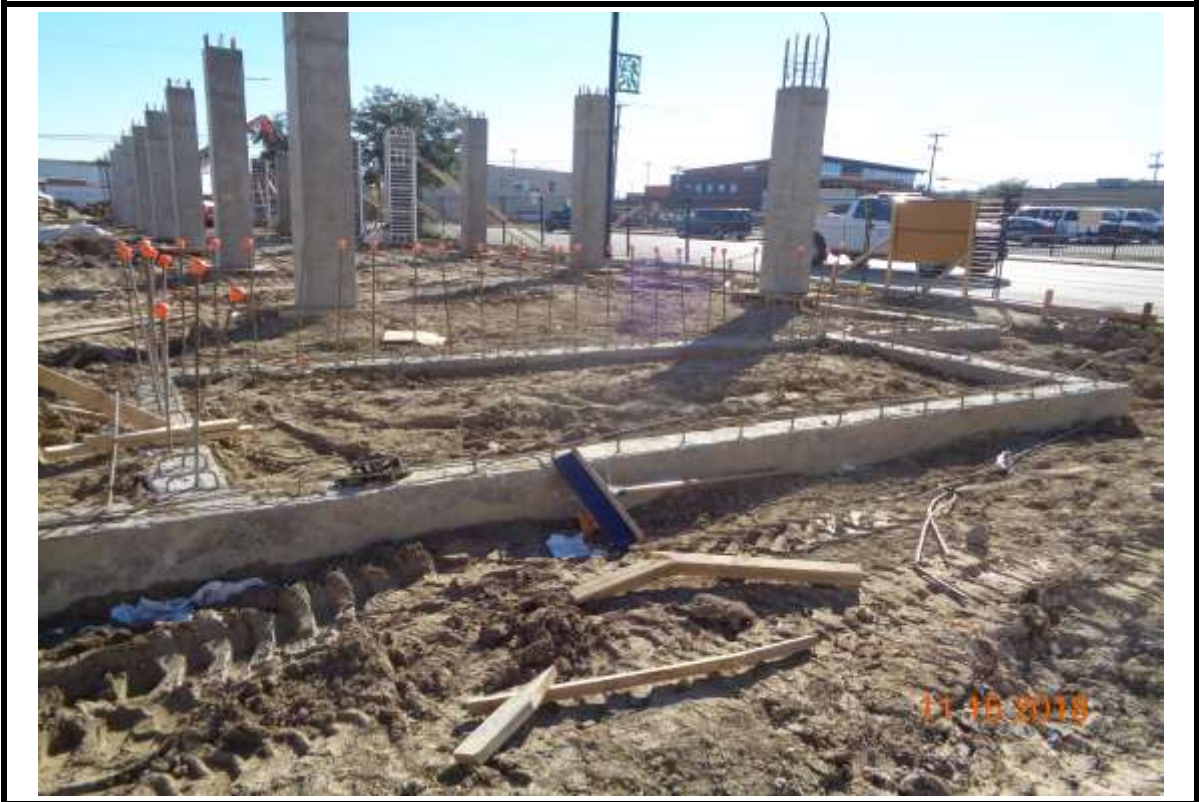
Photograph 3: West stairwell grade beams at Building "A".
