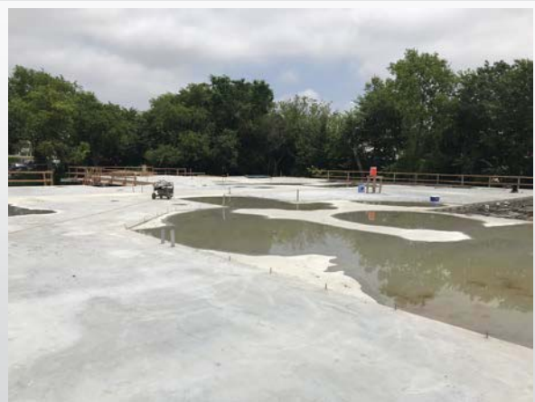
Top of Podium – Building A
