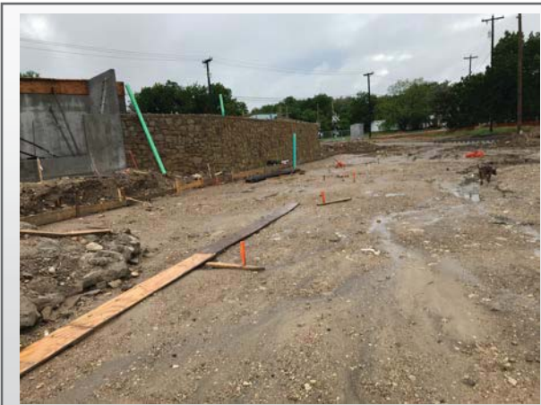
Gravity wall and parking lot between buildings
