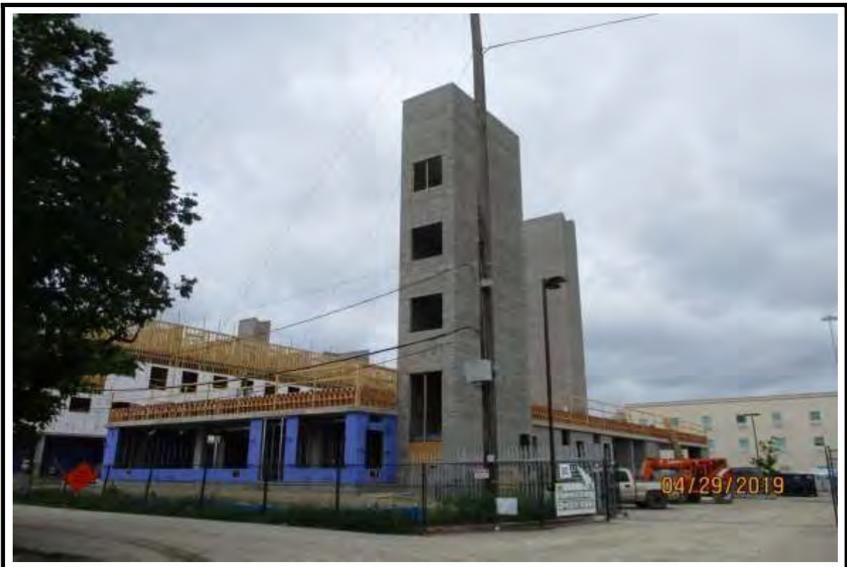
Photograph 6: CMU stair towers and wood framing starting at Building "B".
