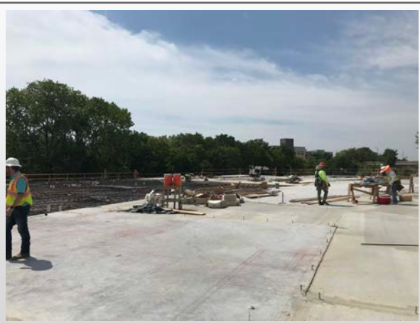
Building A Podium
