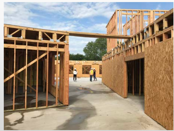
Courtyard Framing on Building A
