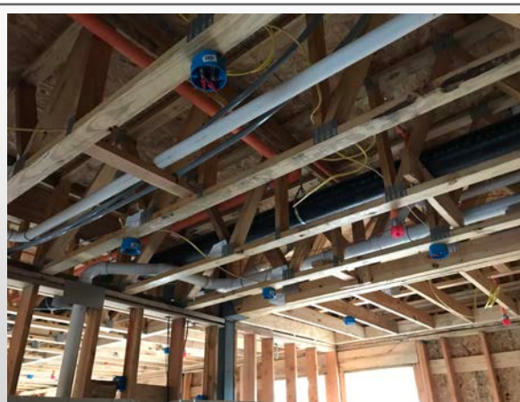
Truss space above clubhouse
