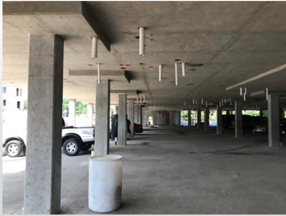
Parking level under podium at Building A
