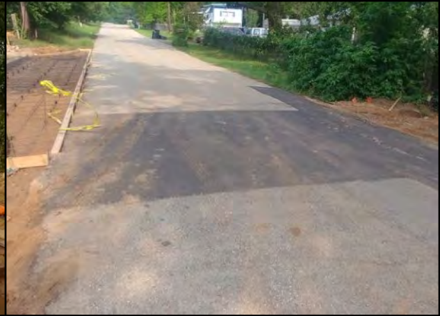
Photo # 2 Completed utility tie-ins at Lindale Cemetery Road
