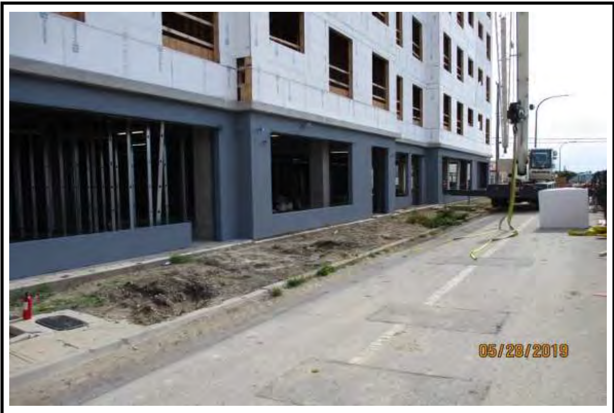
Photograph 4: 1 st floor waterproofing at retail area of Building "A".
