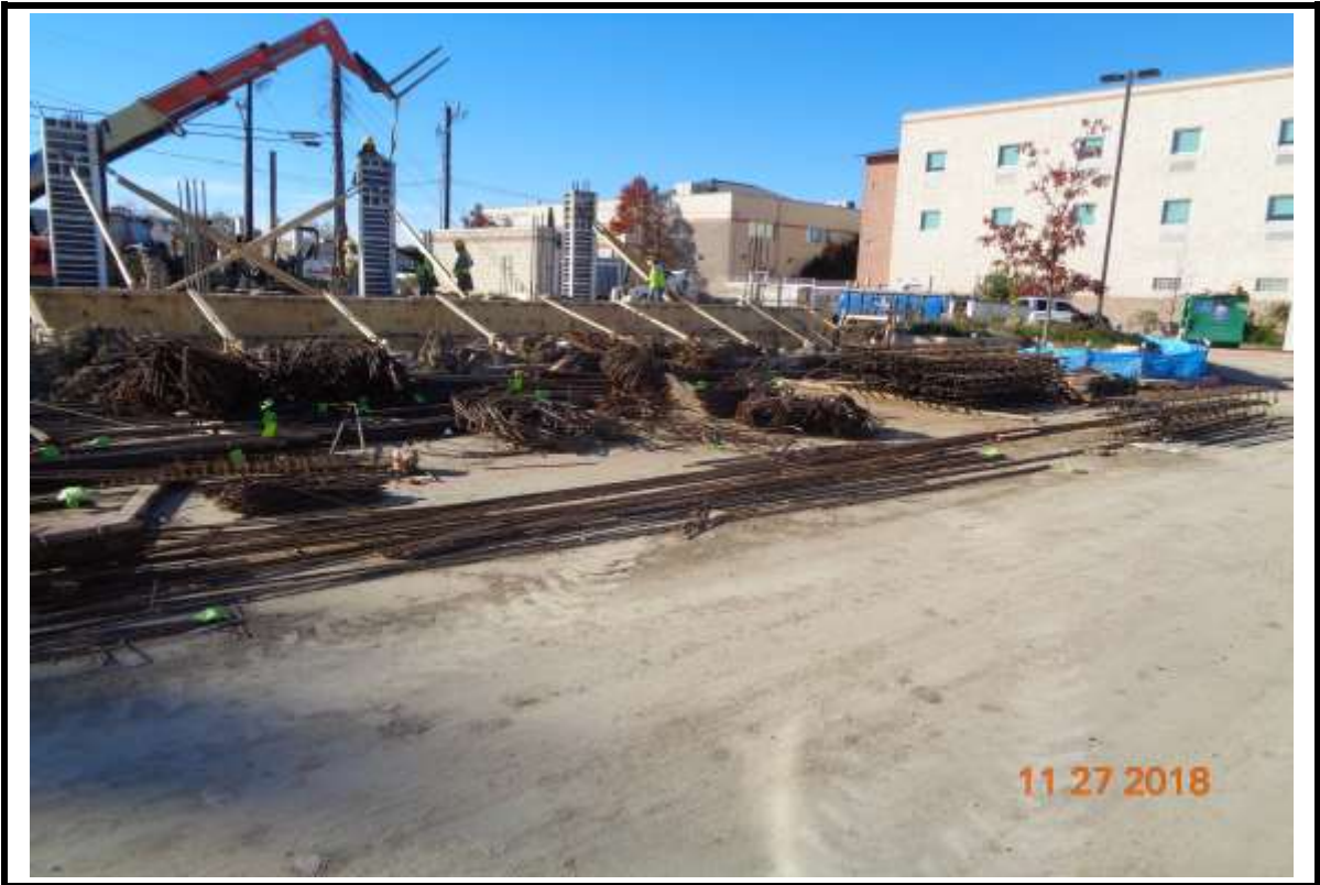
Photograph 1: Column and Podium reinforcing at Building "B".
