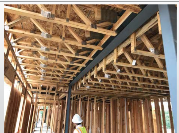
Steel Structural framing – Building B Provide intumescent paint on steel
