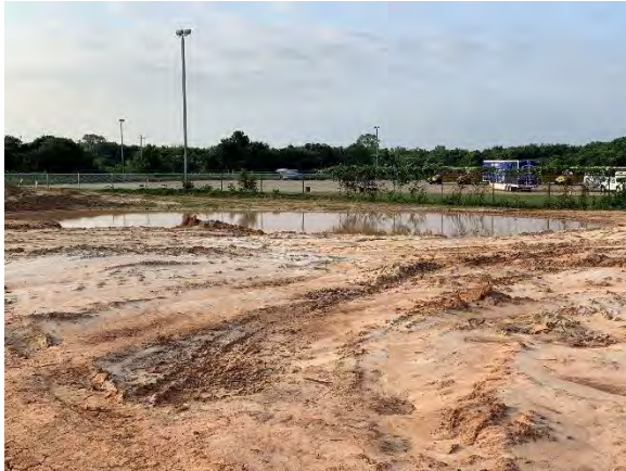
Photo 7: Progress at detention pond on west side of site.
