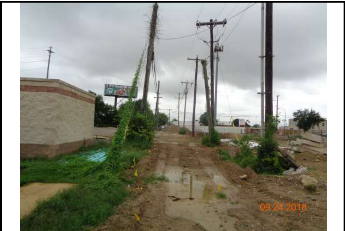
Photograph 12: Abandoned right-of-way between Buildings "A" and "B".
