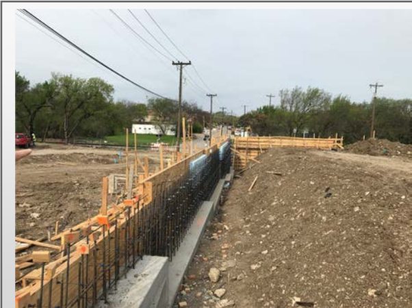
Foundation for Building B
