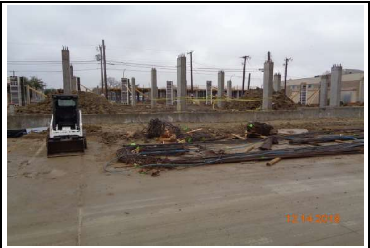
Photograph 1: Completed columns at Building "B".
