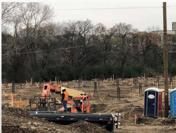
Bldg. A drilled piers with rebar
