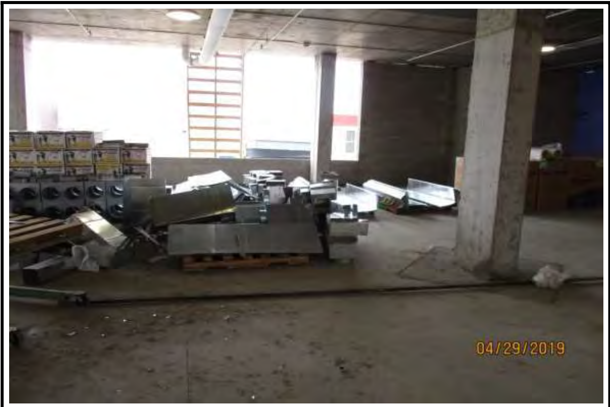
Photograph 8: Duct work ready for installation at Building "B".
