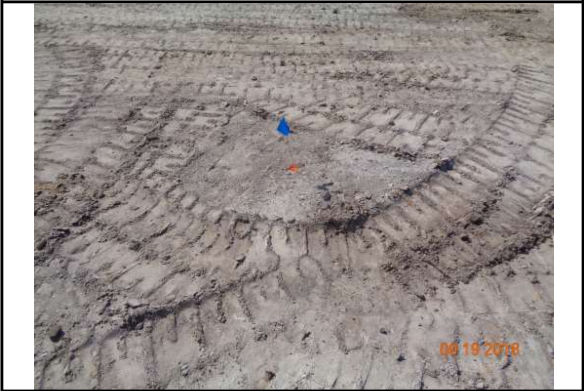
Photograph 7: Pier spotted for layout and starting grade.
