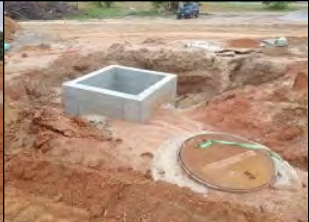
Photo # 8 Completed manhole and ström drain nearing completion
