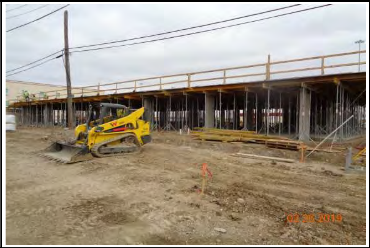
Photograph 5: Regrading for continuation of paving between Buildings “A” and “B”.
