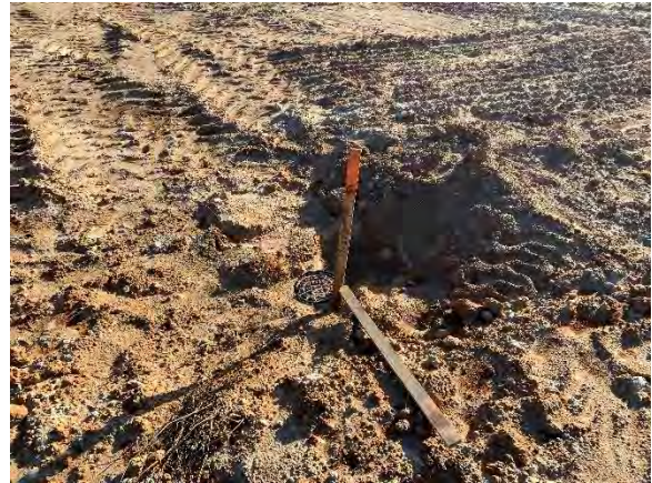
Photo 2: Completed water main tie-in at west side of site.
