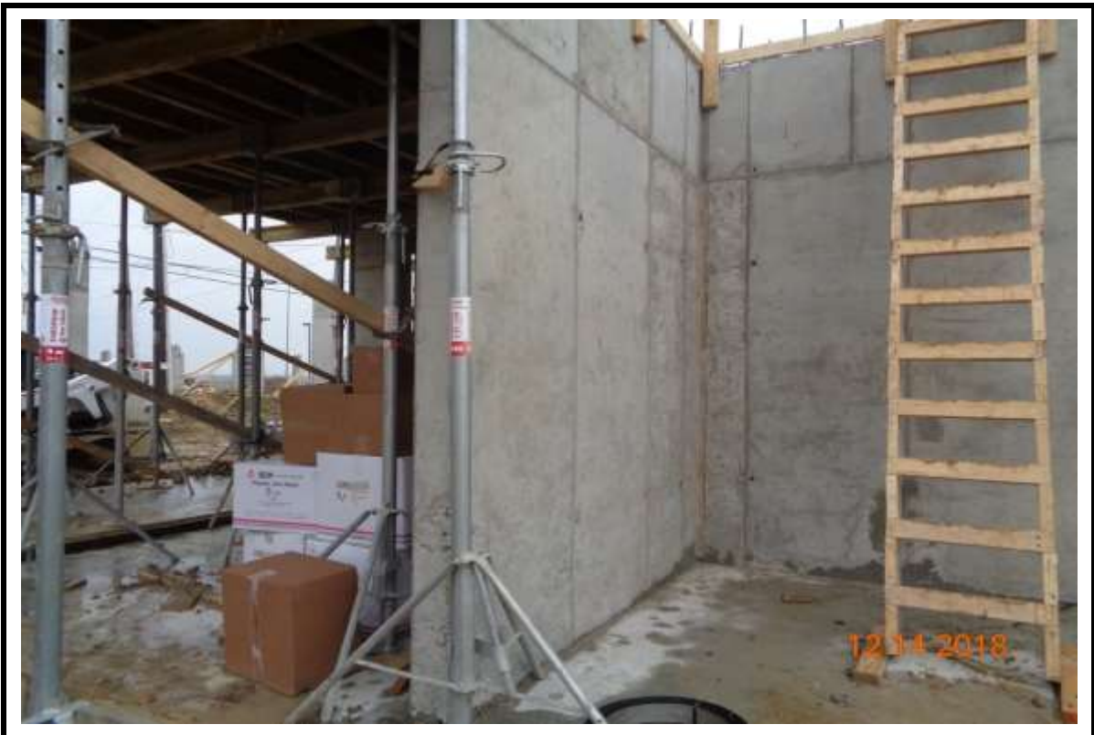
Photograph 6: Poured in place walls at stairwell in Building "A".
