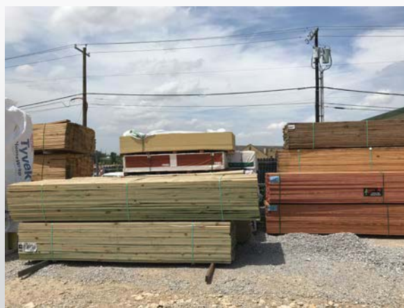
Stored Framing Material
