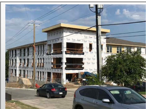
Building B South and East Elevation
