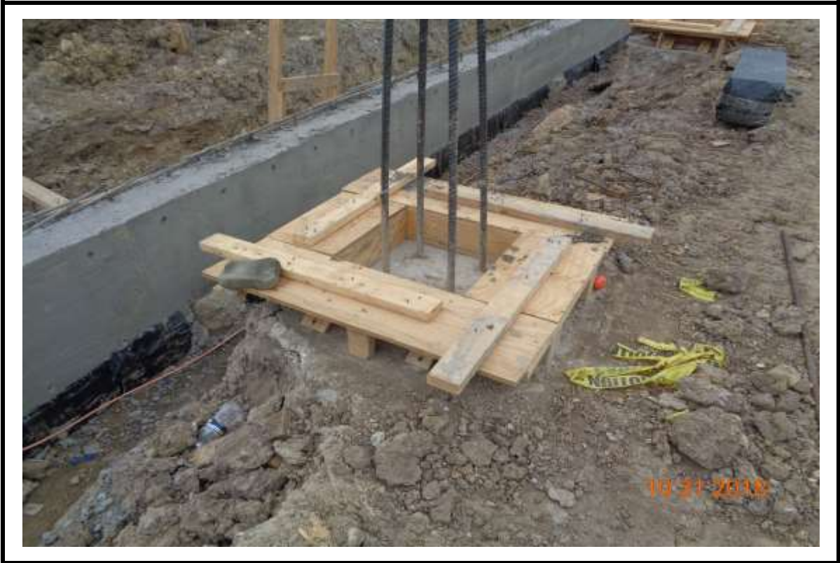
Photograph 7: Column form base.
