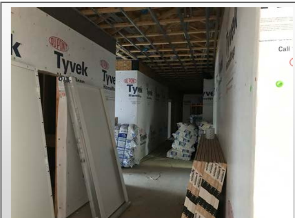
Building B Corridor
