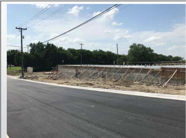
Retaining wall at Building B
