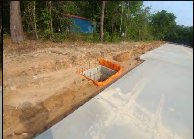
Photo # 4 Pouring of curb inlets still required
