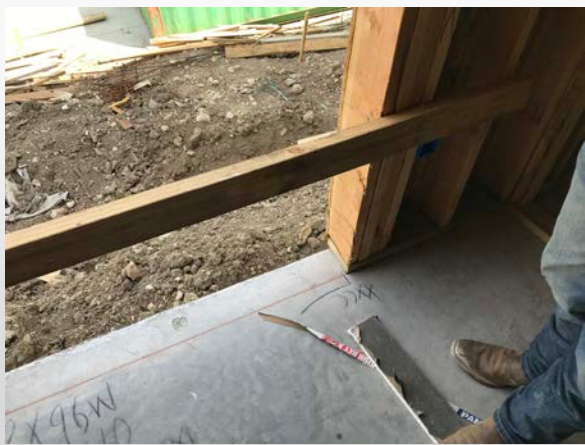
Building B window sill
