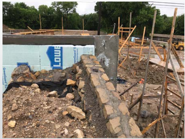
Retaining wall at Building B
