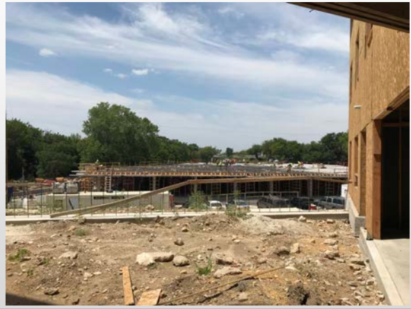
Building B Courtyard
