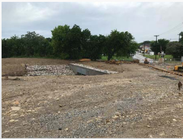
Headwall at Creek
