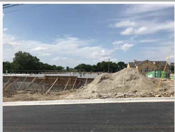
Retaining wall at Building B
