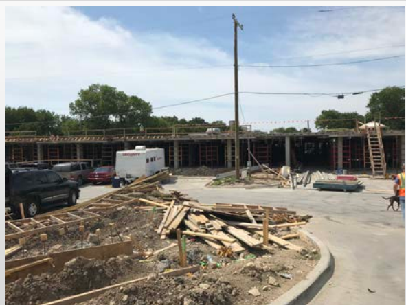
Building A Podium
