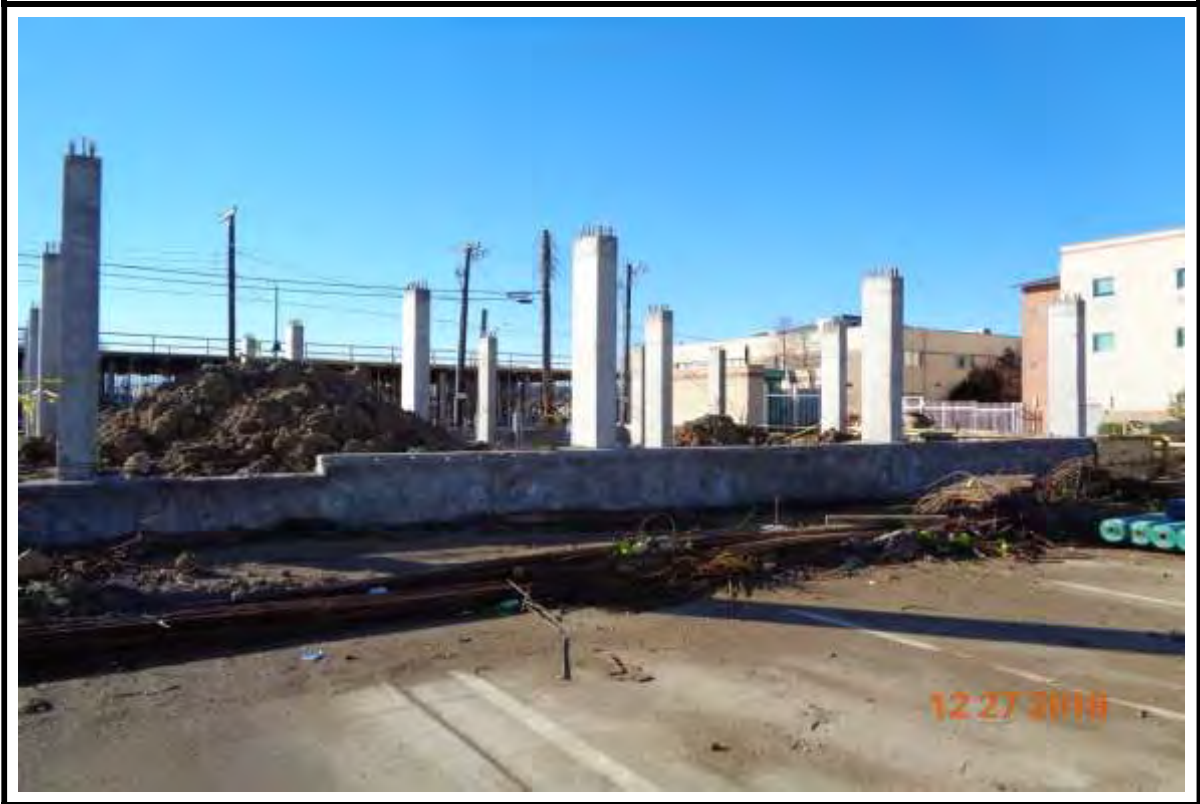
Photograph 9: Completed Podium columns at Building "B" West end.
