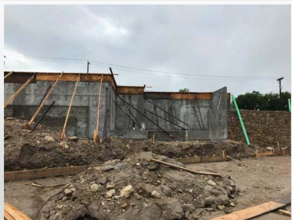
Retaining wall at Building B Stair
