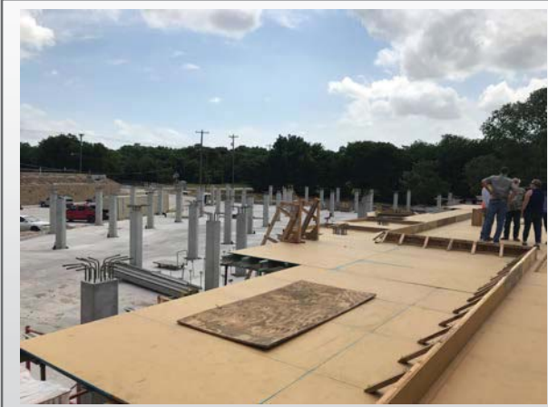
Building A Podium Forming
