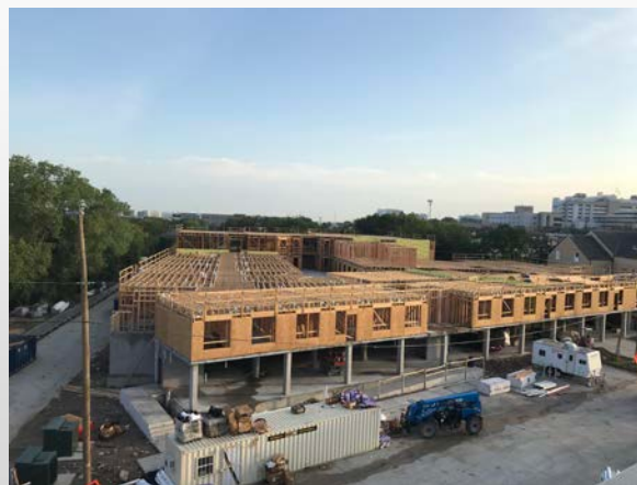
Building A looking from B
