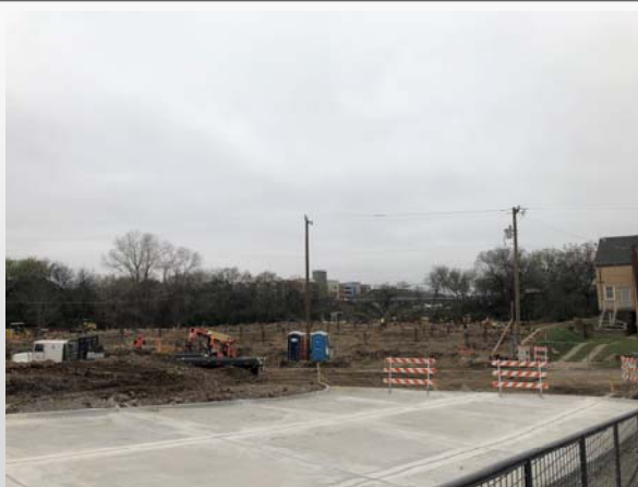
North end of Beckman rd. Bldg. A beyond
