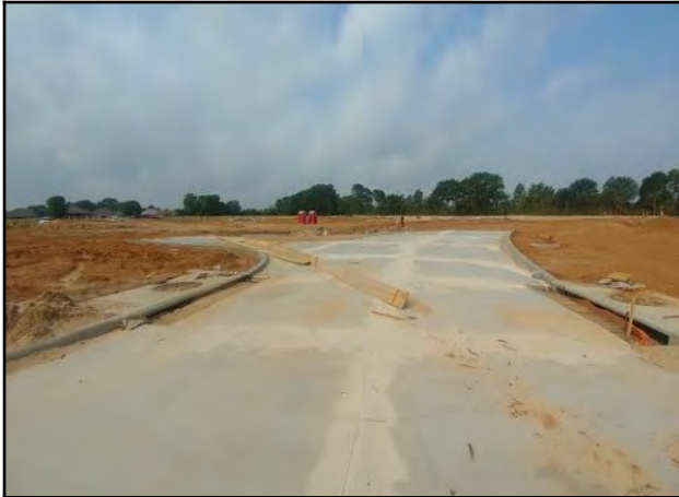
Photo # 7 Paving between building pads and detention pond complete
