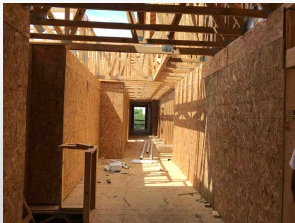
Building B Interior Framing
