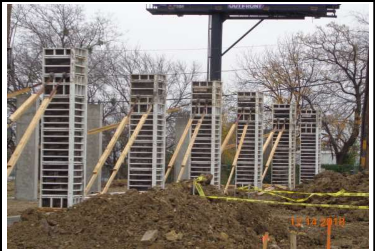
Photograph 3: Last column forms at Building "B".
