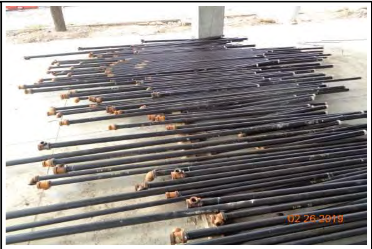
Photograph 4: Sprinkler piping staged for installation at Building "A".
