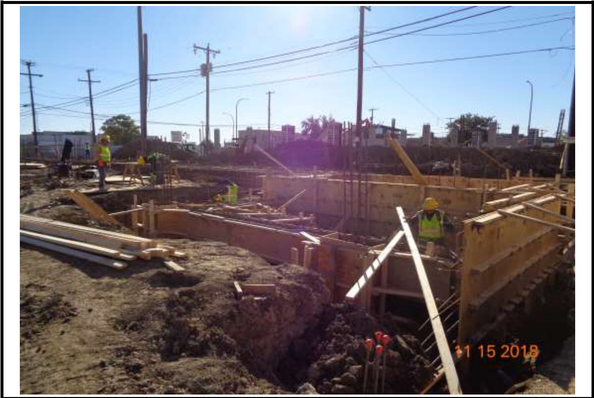
Photograph 1: Setting forms at North grade beam at Building "B".
