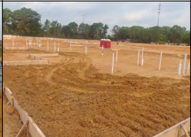
Photo # 16 Building 8 - Concrete forms and under slab plumbing complete
