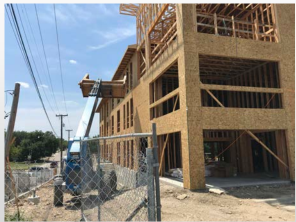
Building B Framing
