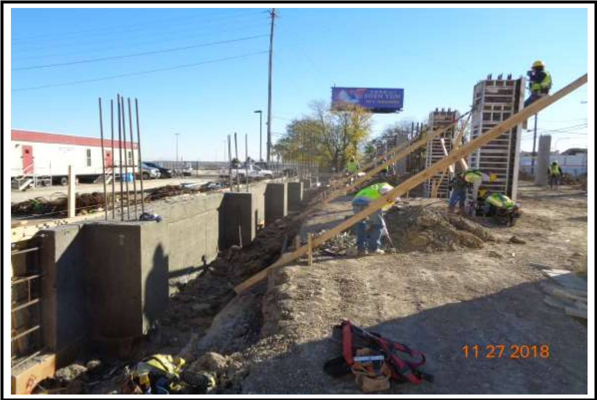
Photograph 2: North grade beam rubbed and ready for backfill Building "B".
