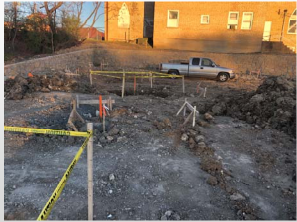
Building A Drilling piers in progress
