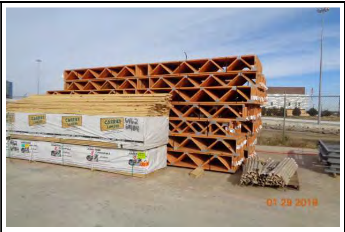
Photograph 1: Sub-floor trusses for 1 st floor units at Building “A”.
