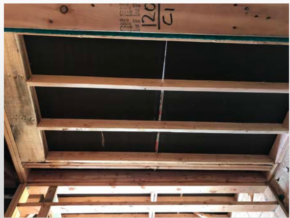
Building B Breezeway
