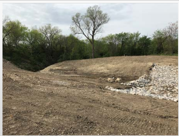
Headwall and drainage construction
