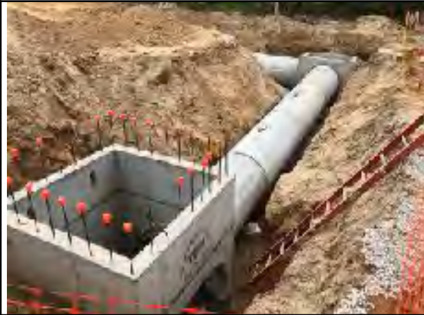
Photo # 1 Storm drainage installed near Lindale Cemetery Road
