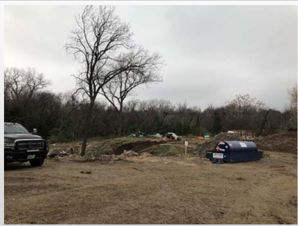
Off-site utility connection work progressing
