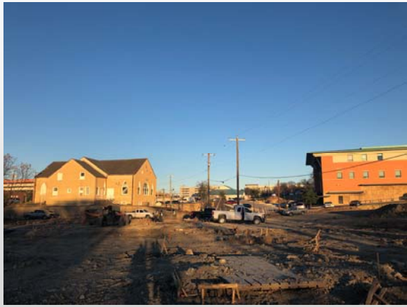
Southwest corner of Building A
