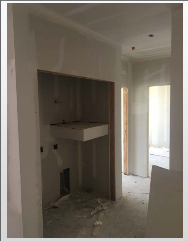
Building A – 2 nd floor
