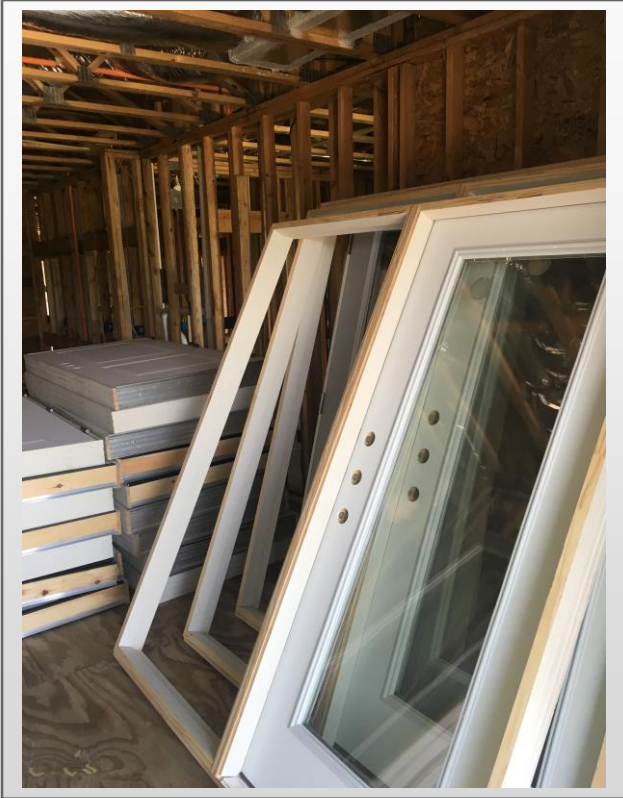
Building #1 – Second Floor
