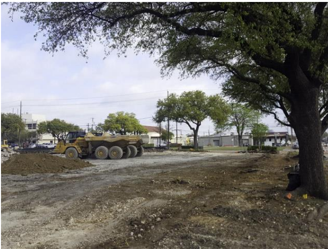
Existing site concrete paving demolition was substantially complete.
