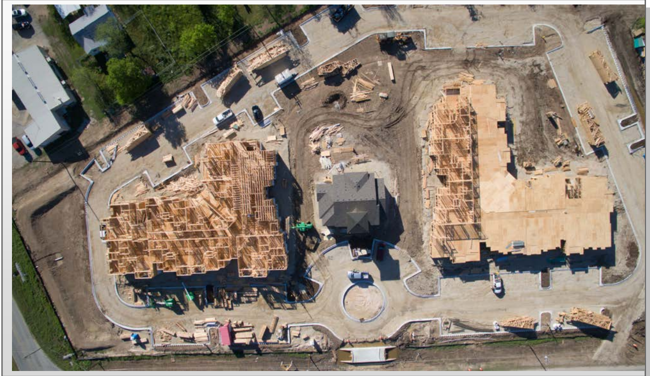
General Site Picture
