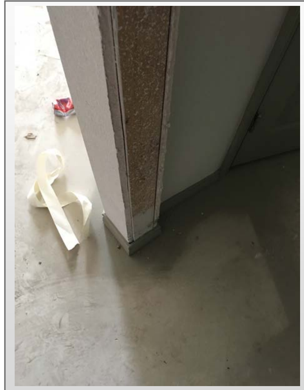
Building #1 trim at unfinished edge
