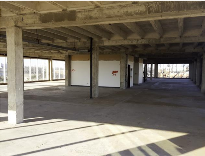
Levels 2 through 6 demolition and abatement were complete.
