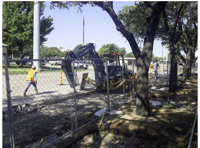
Avenue B roadway improvements were in progress
