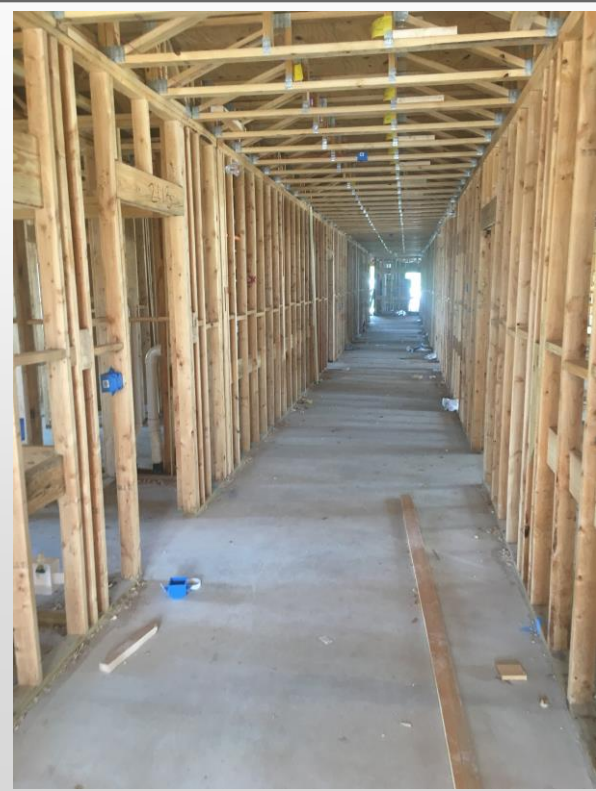
Building #2 – Second Floor
