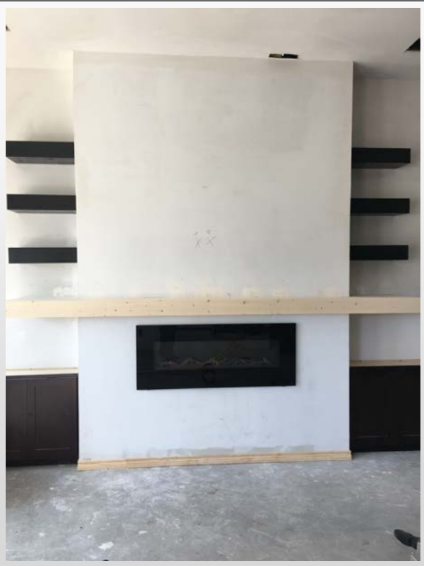
Club great room fireplace installed
