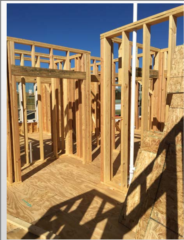
Building #1 – 3 rd Floor
