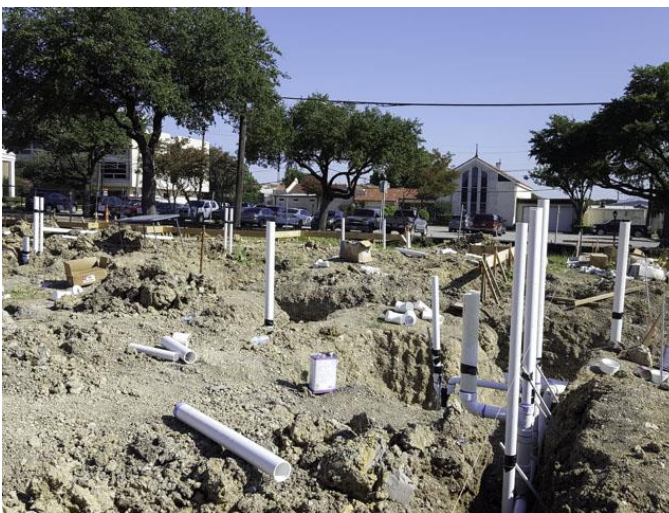
Building A under slab utility rough-ins were nearing completion.
