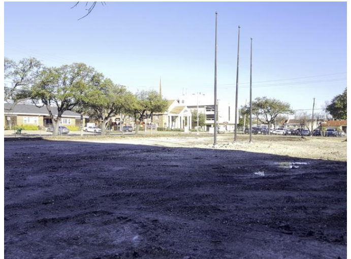
Office building site parking paving demolition was complete.
