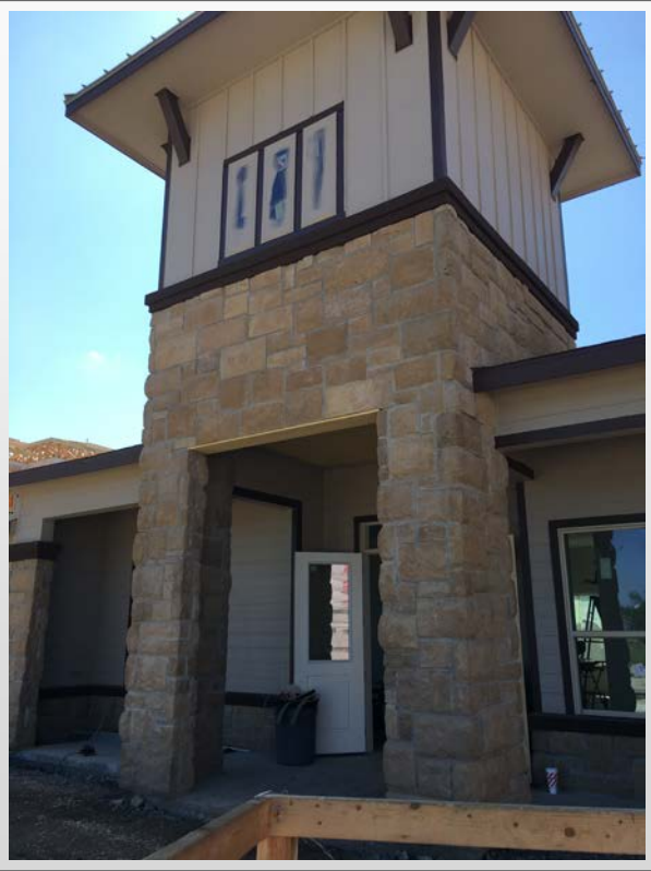
Club exterior nearing completion
