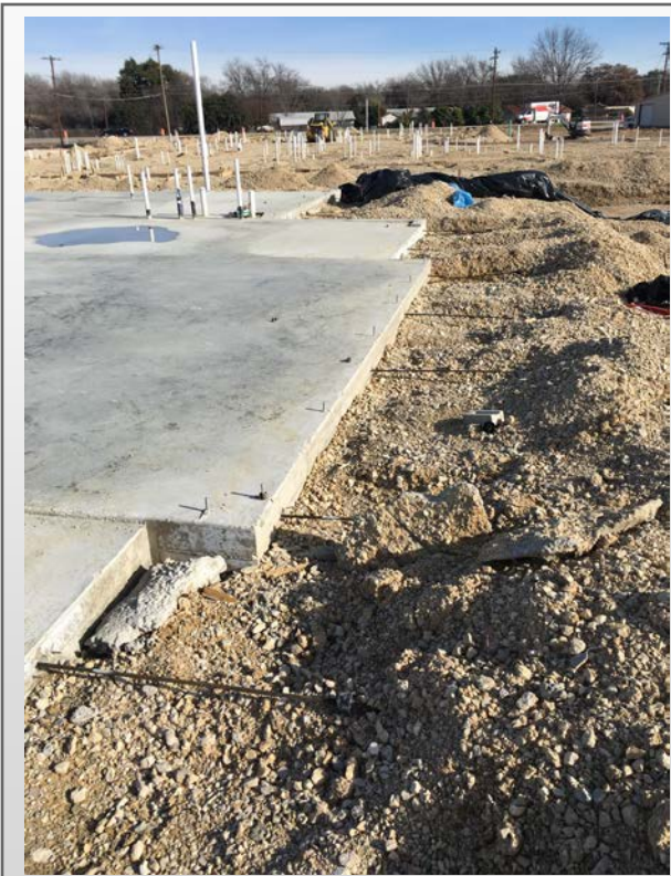
Building #3 – Slab in place
