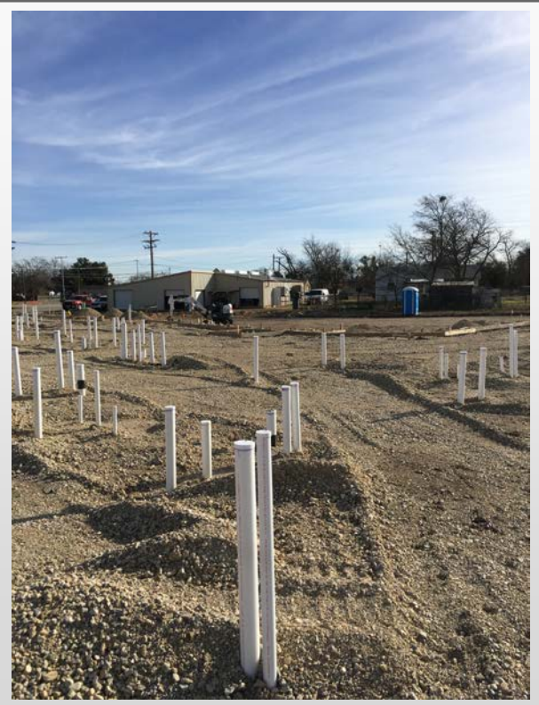
Building #1 – Forms in place
