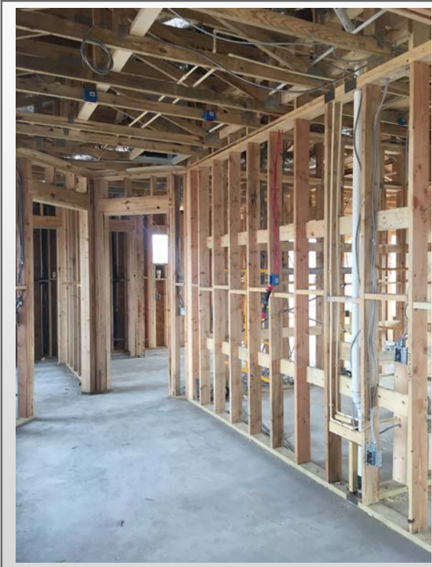
Club – interior ready for insulation
