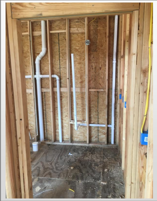
Building #1 – Third Floor
