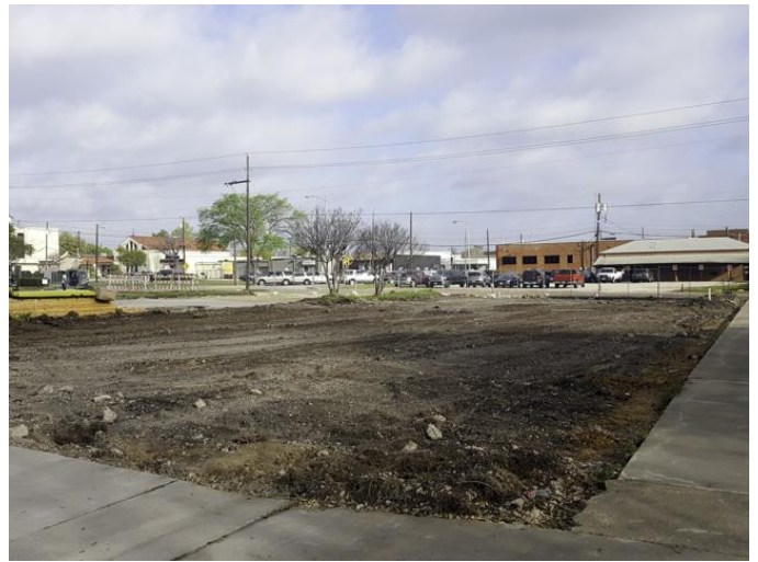
Existing site concrete paving demolition was substantially complete.
