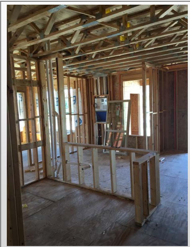
Building #2 - 2 nd floor
