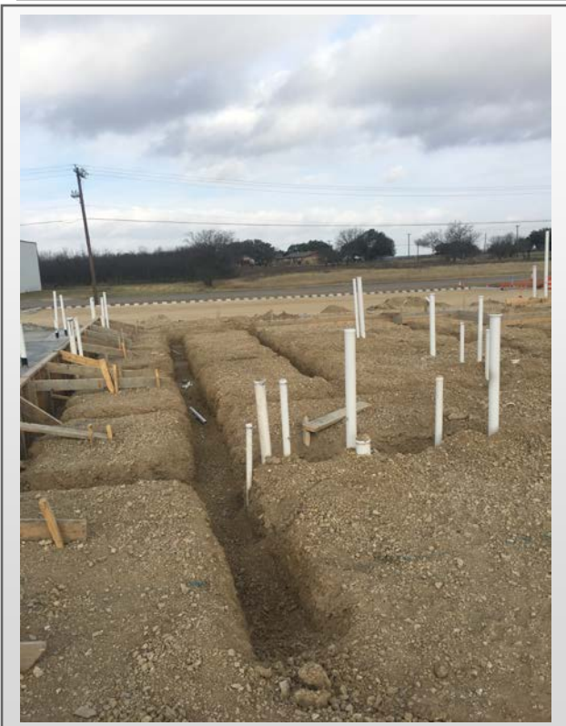
Building #2 grade beams in preparation for the last pour
