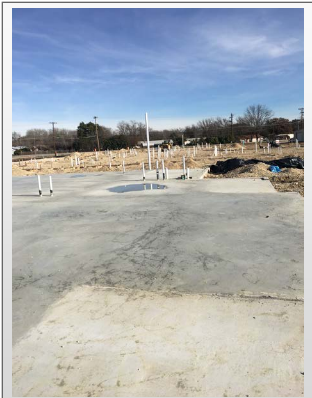
Building #3 – Slab in place
