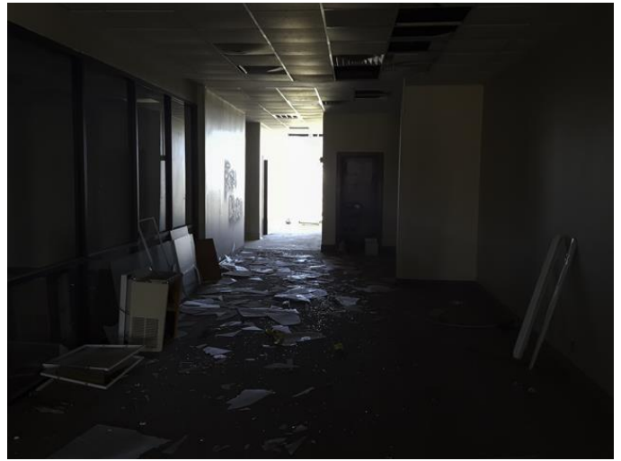
Level 1 demolition was nearing completion.
