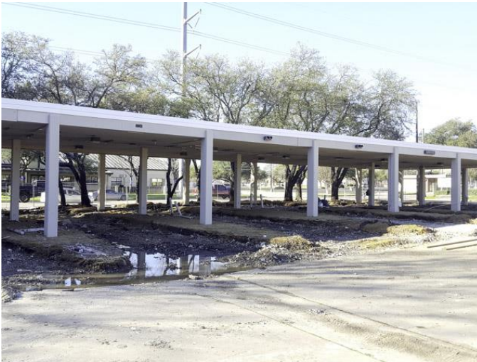
Existing drive-thru bank demolition was in progress.
