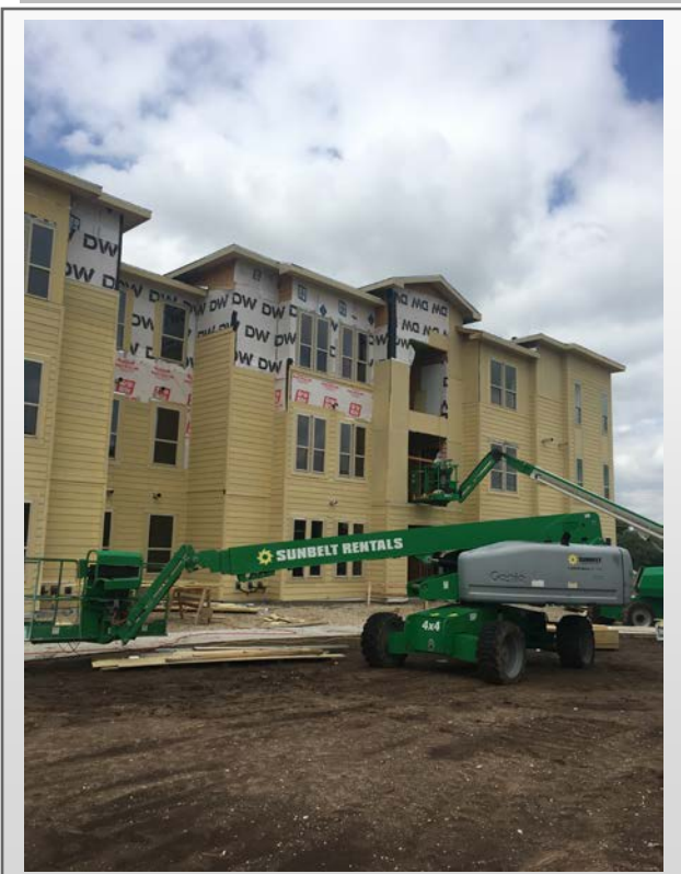
Building B - Exterior
