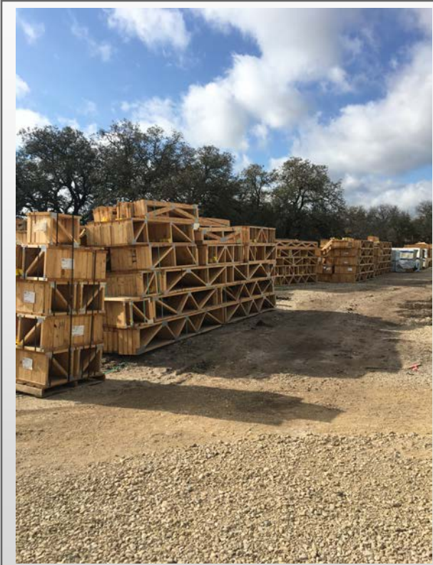
Stored Floor Trusses
