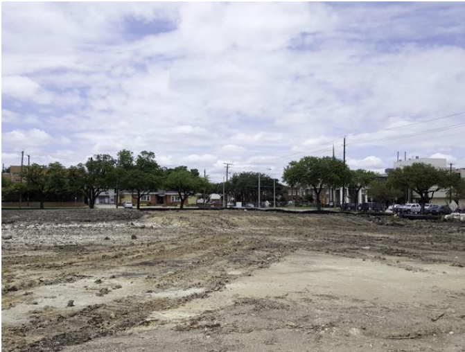
Building A pad preparation was substantially complete.
