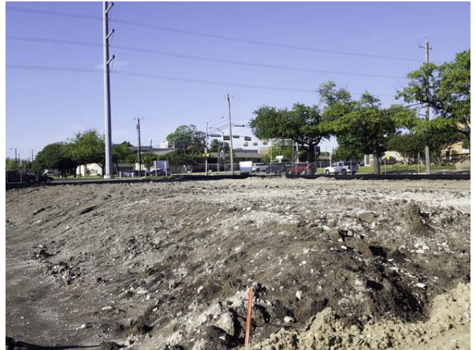
Building A pad preparation was nearing completion.
