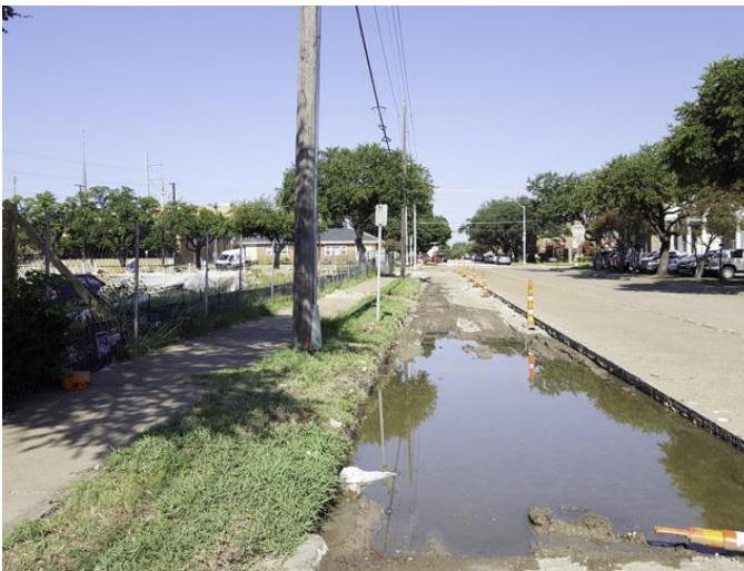
Avenue A roadway improvements were in progress.
