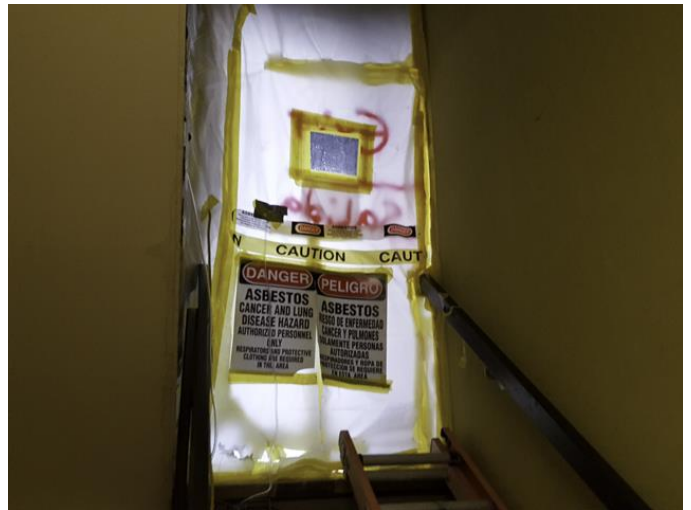
Existing Building Levels 5 and 6 abatement was observed in progress.
