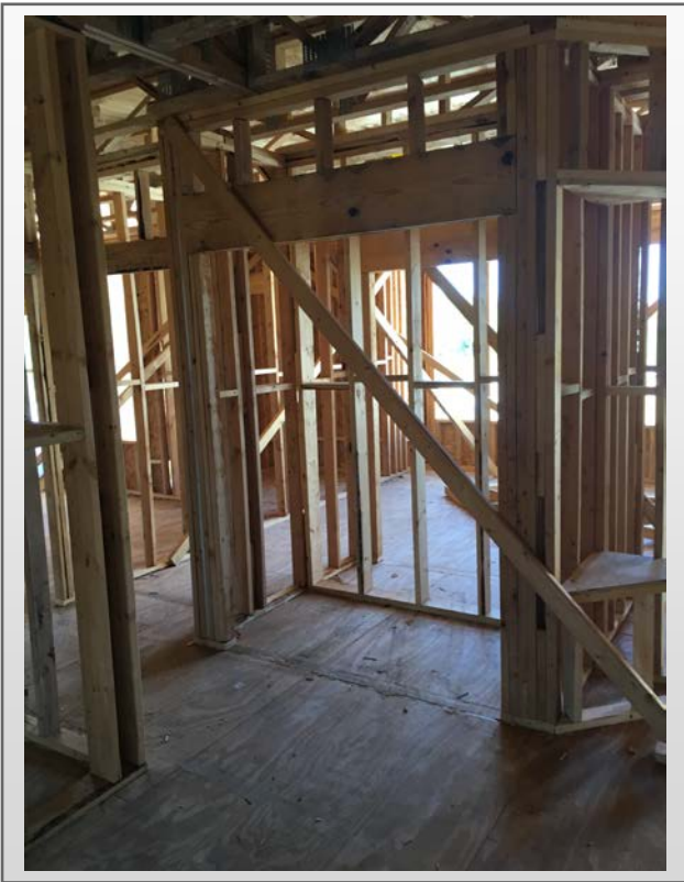
Building #2 – 2 nd floor
