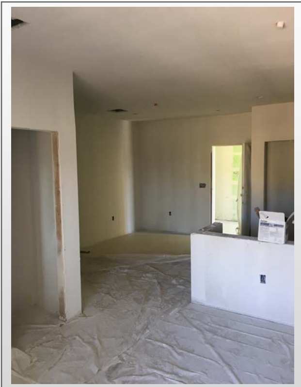
Building #1 Unit 1310- tape bead and texture complete
