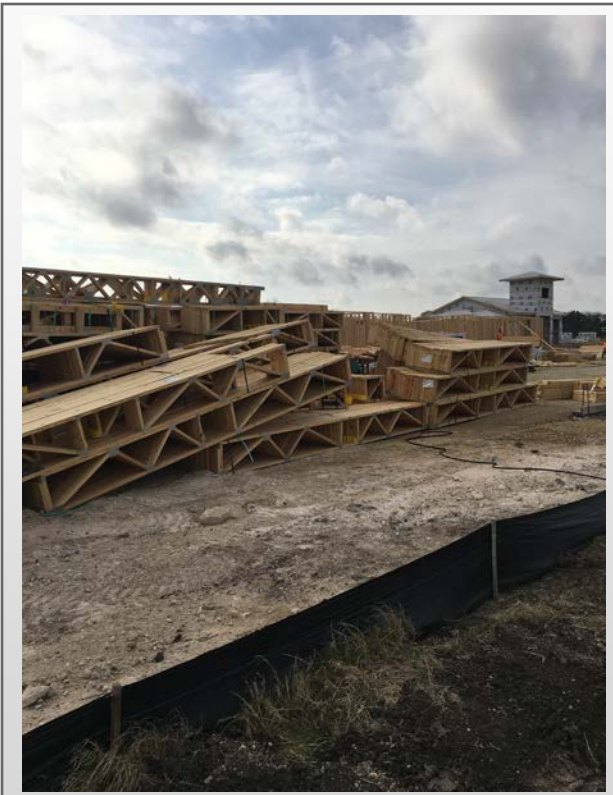
Building #1 – ensure proper laydown of trusses
