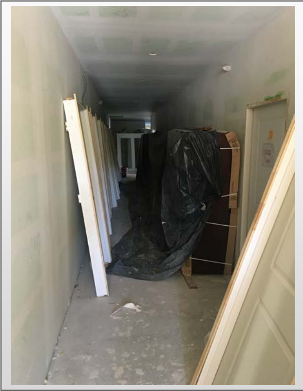
Building #1 – doors and cabinets stocked and ready for install
