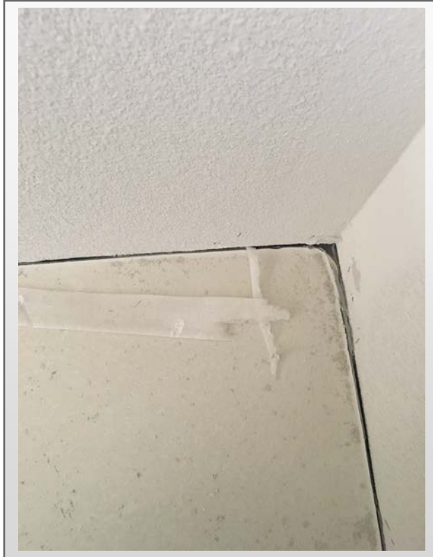
Building #1 Unit 1202 – Gypcrete installed. Ensure fireproofing is maintained
