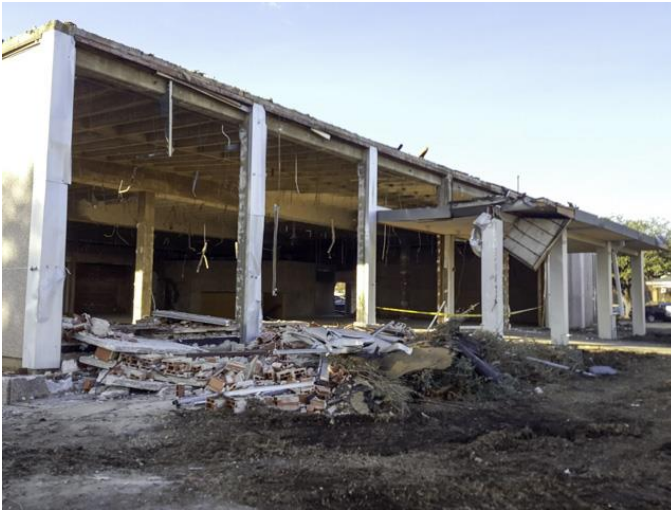
Existing Bank Building demolition was well under way.
