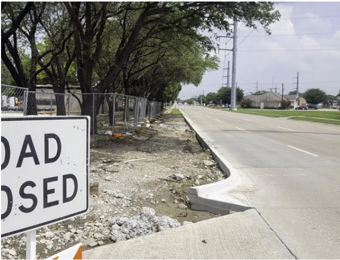
Avenue B roadway improvements were complete.
