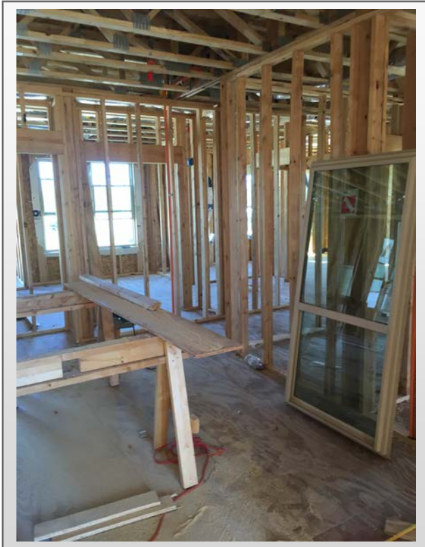
Building #1 – 2 nd Floor
