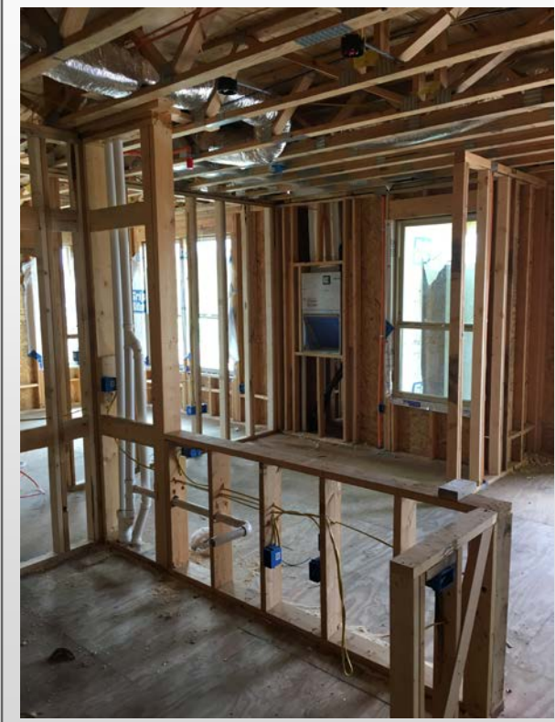
Building B – 2 nd floor
