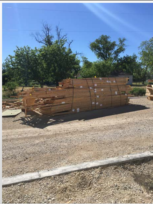
Building #1 Roof Trusses
