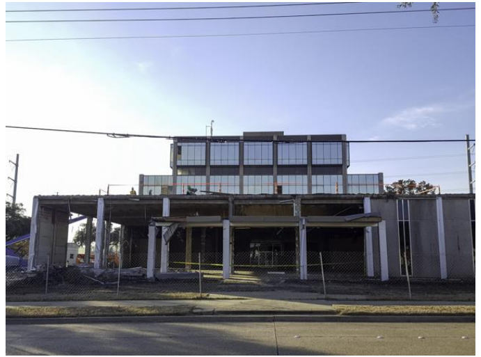
Existing Bank Building demolition was well under way.
