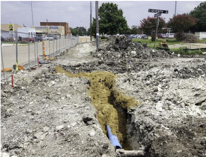
Off-site water main connection was nearing completion.
