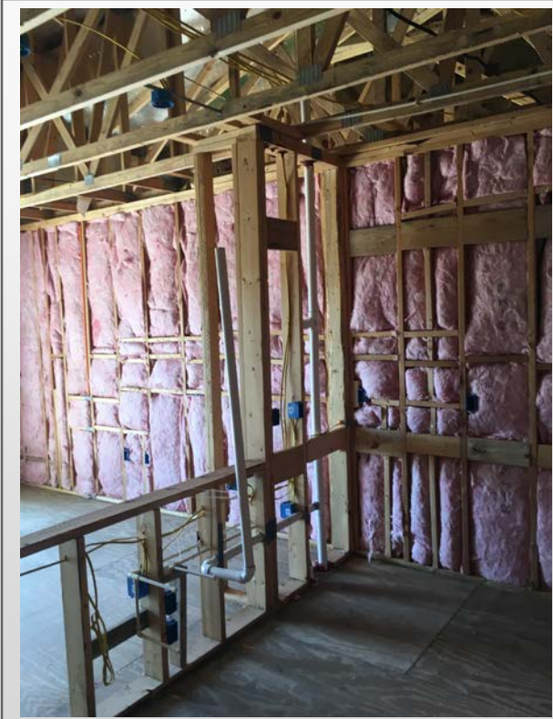
Building #2 Third floor unit
