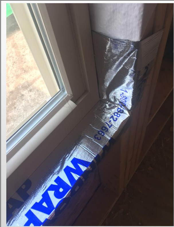
Window wrap sill flashing installed
