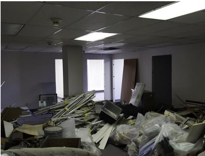
Existing Building Levels 2, 3, and 4 demolition was in progress.
