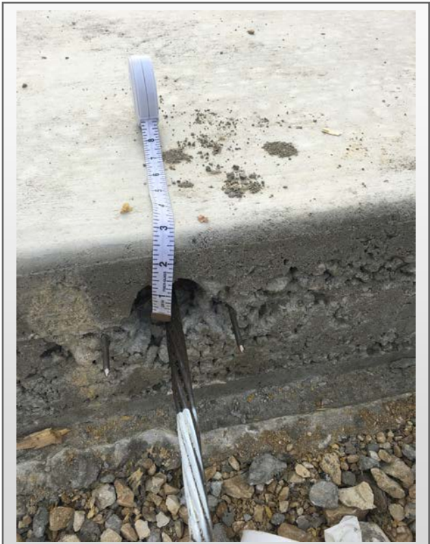
Building #1 – ensure proper tendon head coverage
