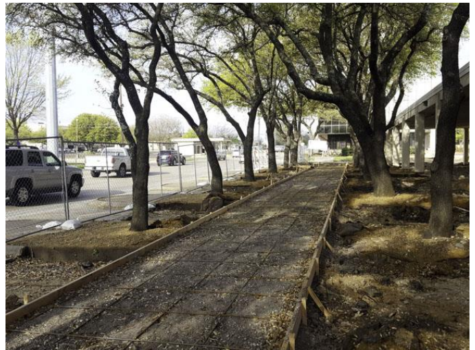
Perimeter sidewalk construction was in progress.
