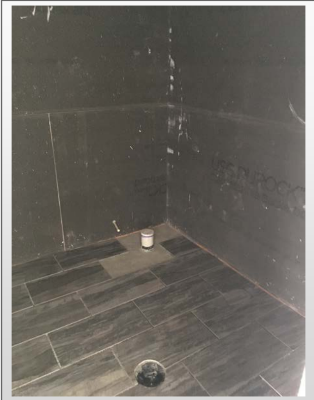
Club restroom tile being installed
