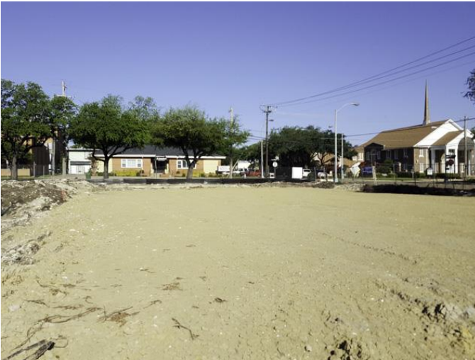
Building A pad preparation was nearing completion.
