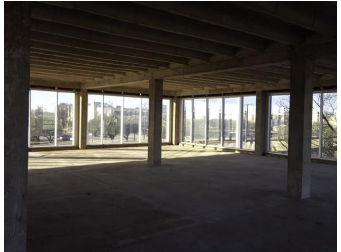
Levels 2 through 6 demolition and abatement were complete.
