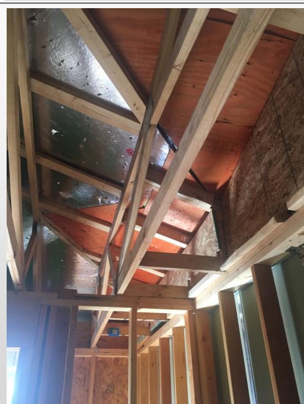
Building #2 – Third Floor
