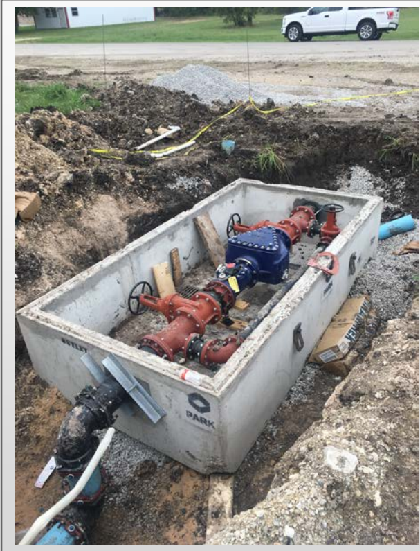
Water main installed
