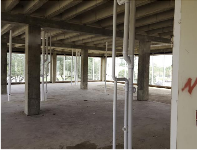
Building B unit sewer utility rough-ins were nearing completion.
