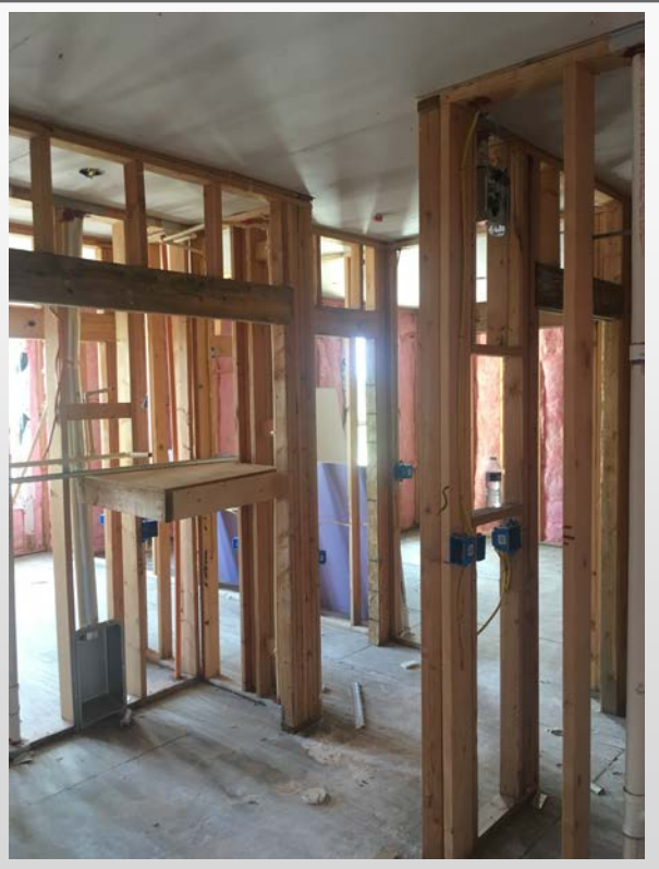
Building A – 3 rd floor
