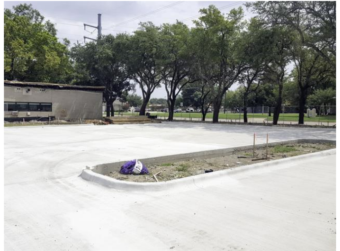
Site parking area concrete paving was in progress.
