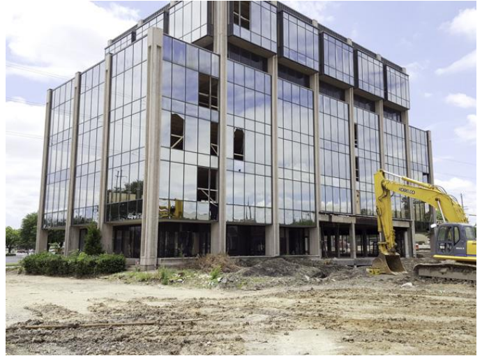
Existing bank building demolition was substantially complete.
