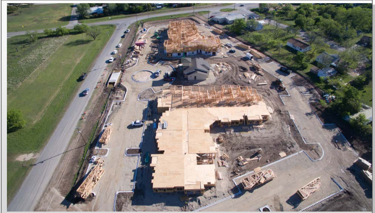
General Site Picture
