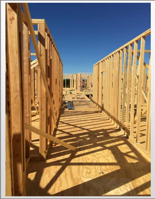
Building #2 – 3 rd floor
