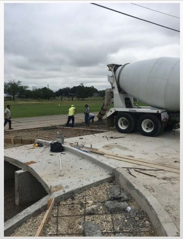
Main entry being poured
