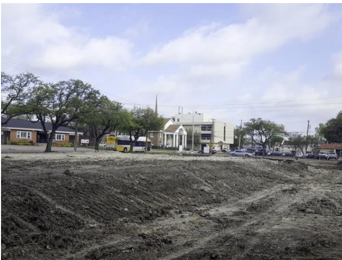
Building A pad preparation was well under way.
