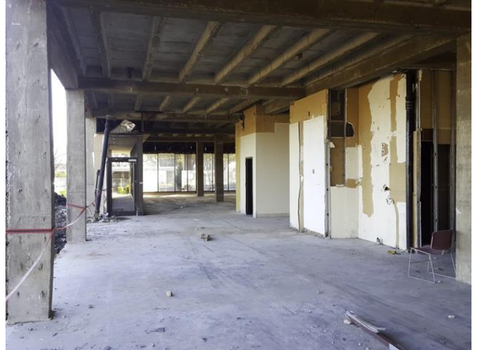
Level 1 demolition was complete.
