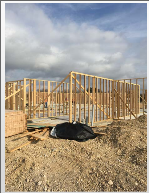
Building #1 framing underway
