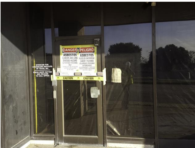
Existing Building Levels 1 and 2 abatement was observed in progress.
