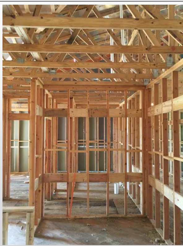
Building #2 - 3 rd floor
