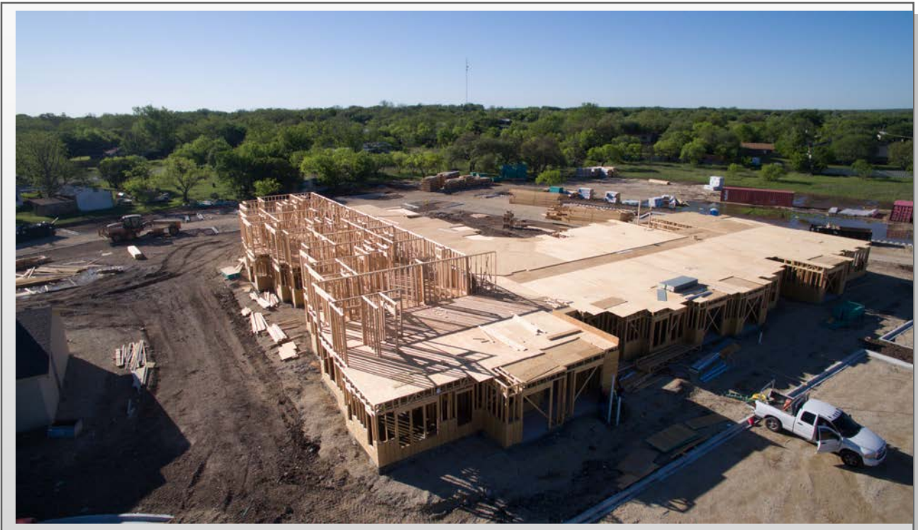
General Site Picture
