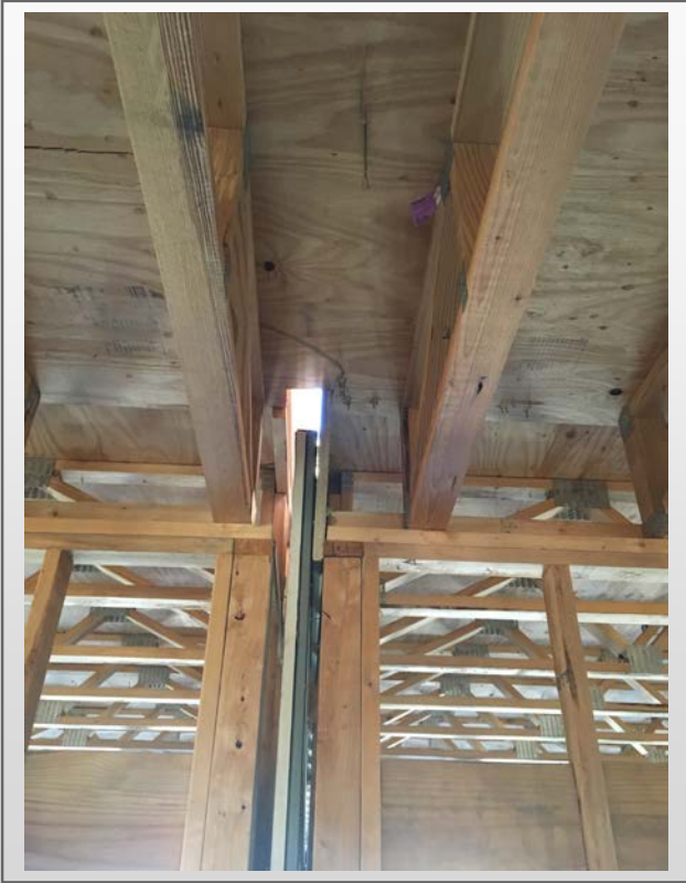
Building #2 firewall at 2 nd floor
