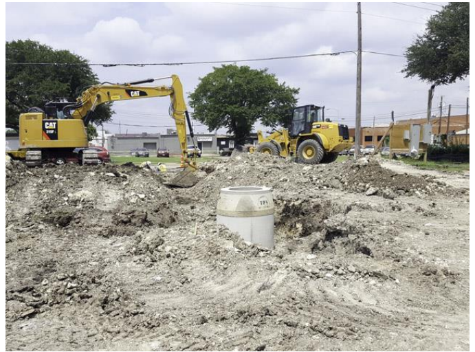
Off-site sanitary sewer main connection was nearing completion.
