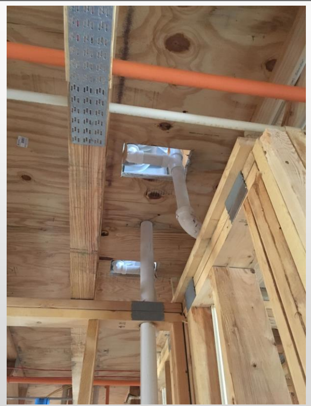
Ensure tub holes are patched
