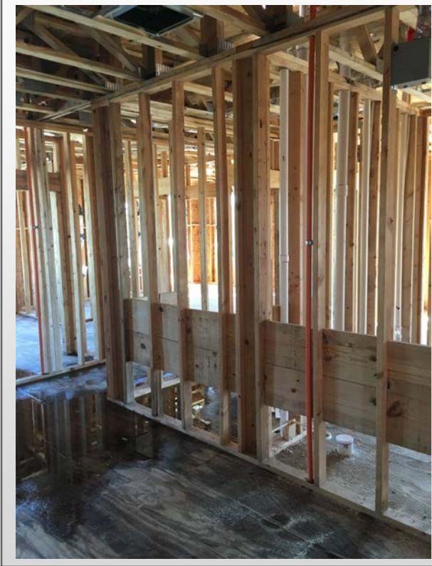
Building #1 - 2 nd floor
