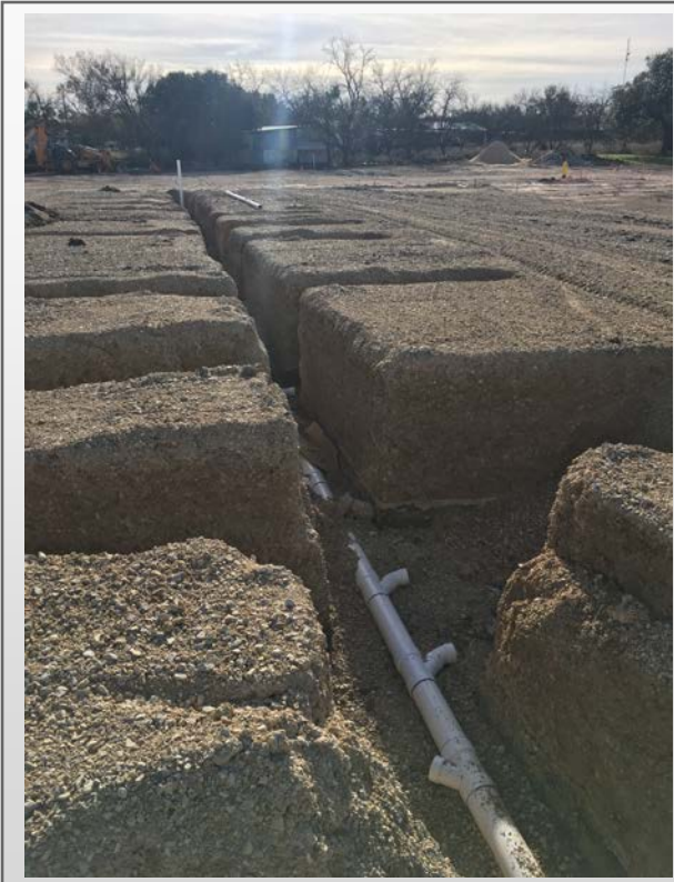
Building #2 – Plumbing underway
