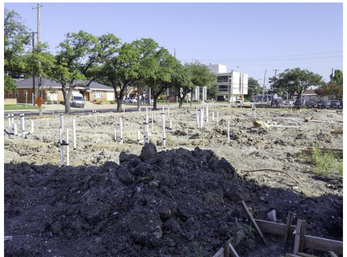
Building A under slab utility rough-ins were nearing completion.
