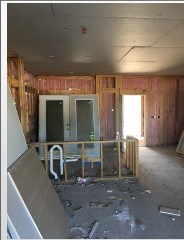
Building #2 First floor unit
