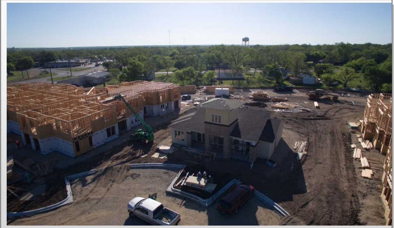
General Site Picture
