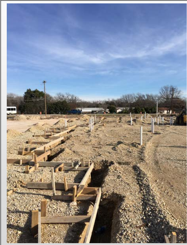
Building #1 – Forms in place
