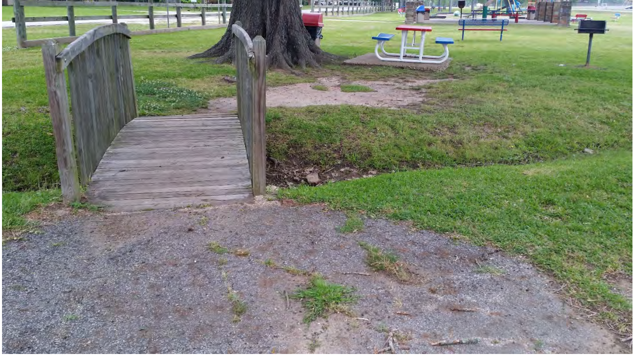
'Bridge' crossing over drainage ditch
