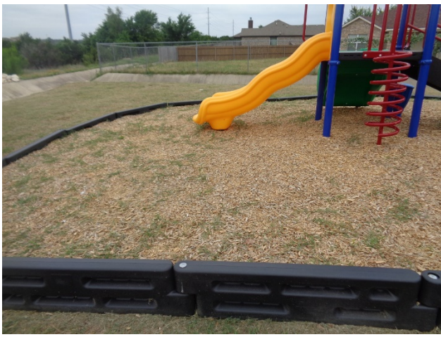
Grass growing through accessible surface
