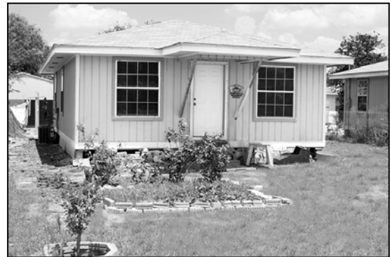
Above: This home in Pharr was built through the Texas Bootstrap Loan Program with funds from TDHCA and labor from the homeowner.
