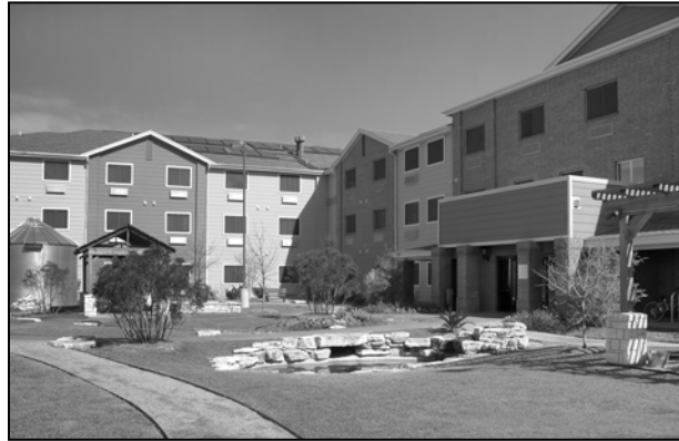
Above: A Multifamily Bond development, Spring Terrace in Austin is a Single-Room-Occupancy complex that has “green” features such as solar panels and a rain collector.
